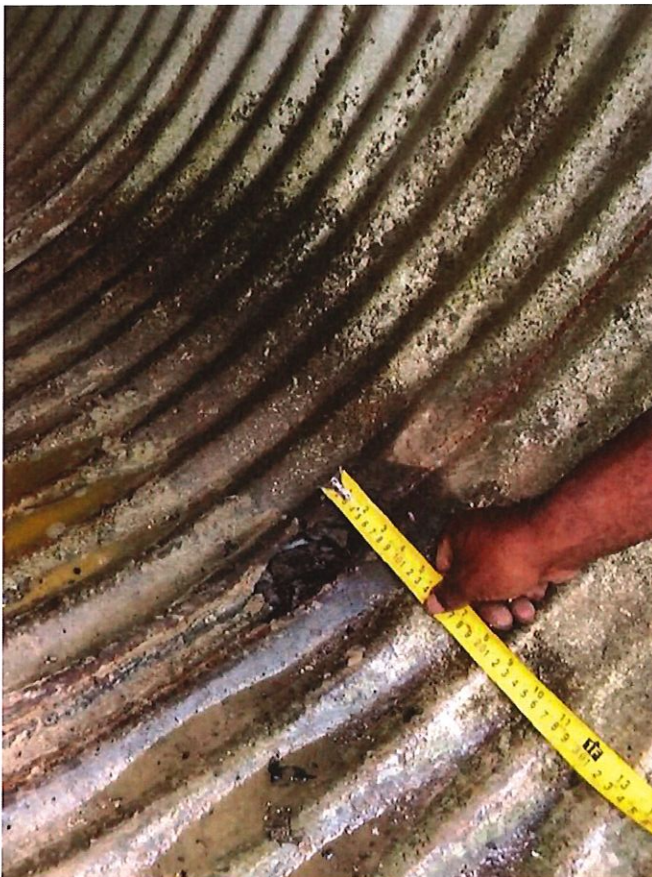
Photo 25 (Hole In invert 6" x 8")
