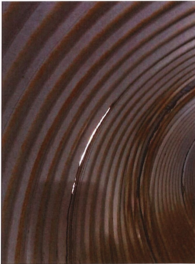
Photo 17 7' 10" from Joint Circumferential Crack – 4' 6" Long from 1:00 – 5:00
