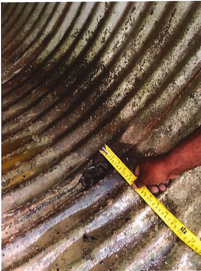
Photo 25 (Hole In invert 6" x 8")
