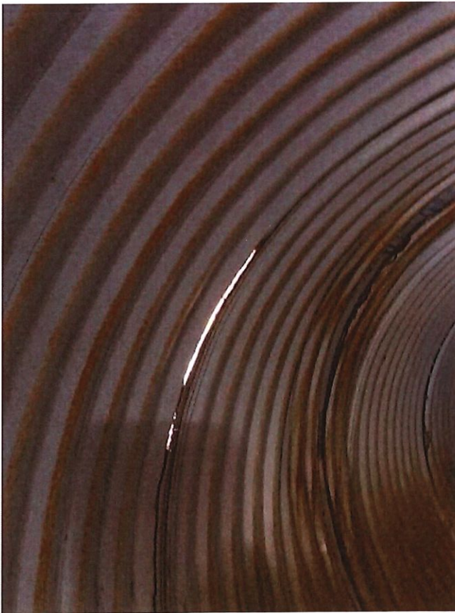
Photo 17 7' 10" from Joint Circumferential Crack – 4' 6" Long from 1:00 – 5:00
