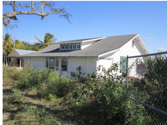
Photo #4 View of building facing northeast.
