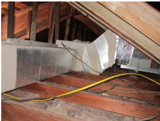
Photo #11 View of attic.
