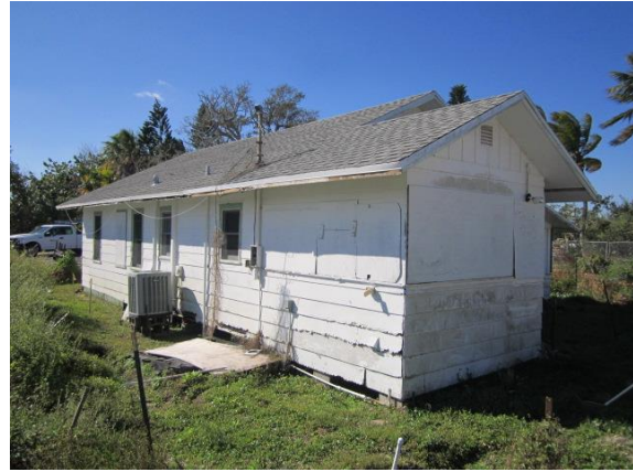
Photo #2 View of building facing southwest.
