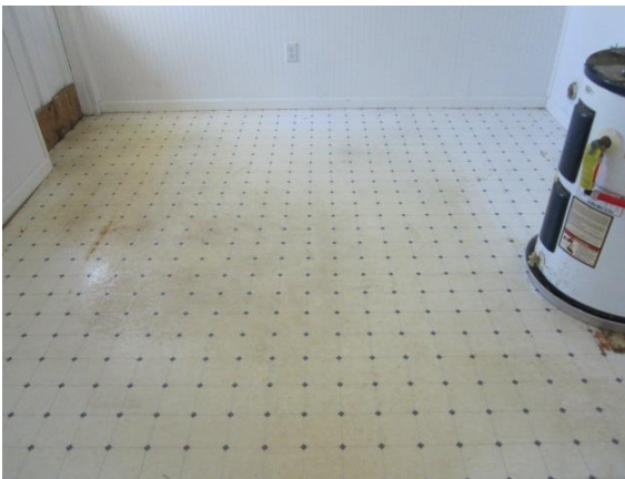
Photo #5 View of off-white & blue "box" pattern SVF reported to be ACM.
