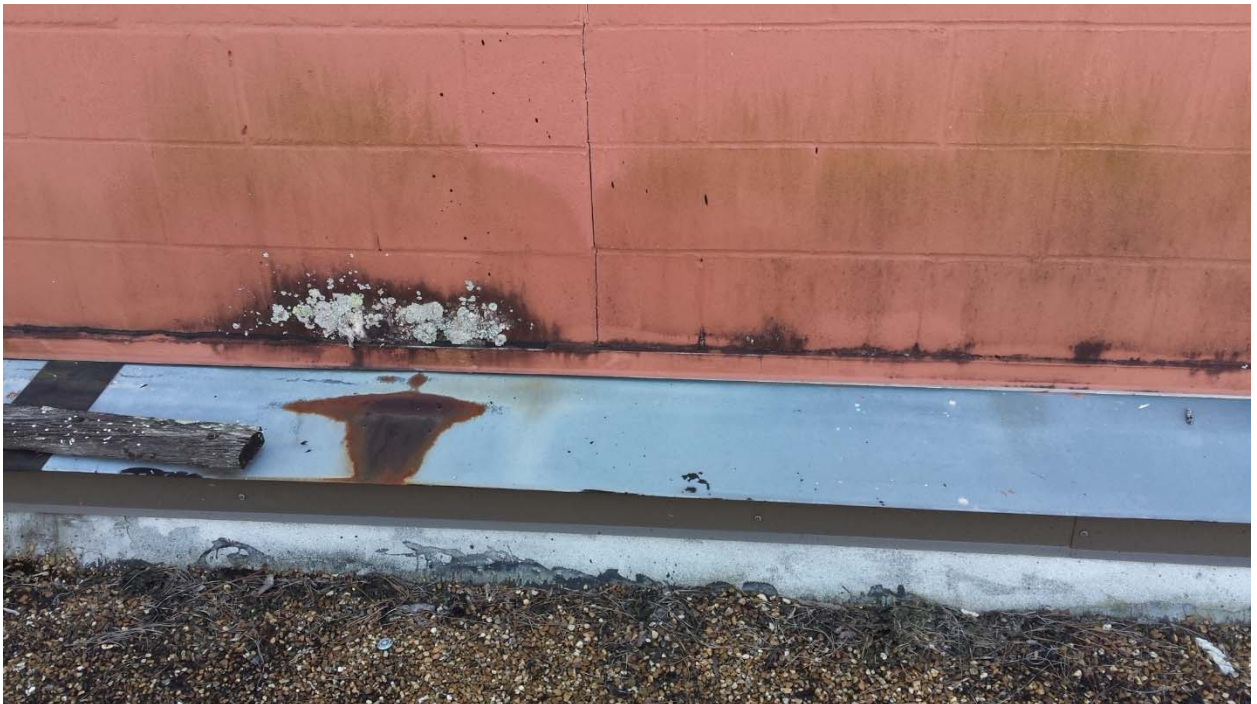
Existing reglet flashing (same color as block). Also shown is vertical crack in block.
