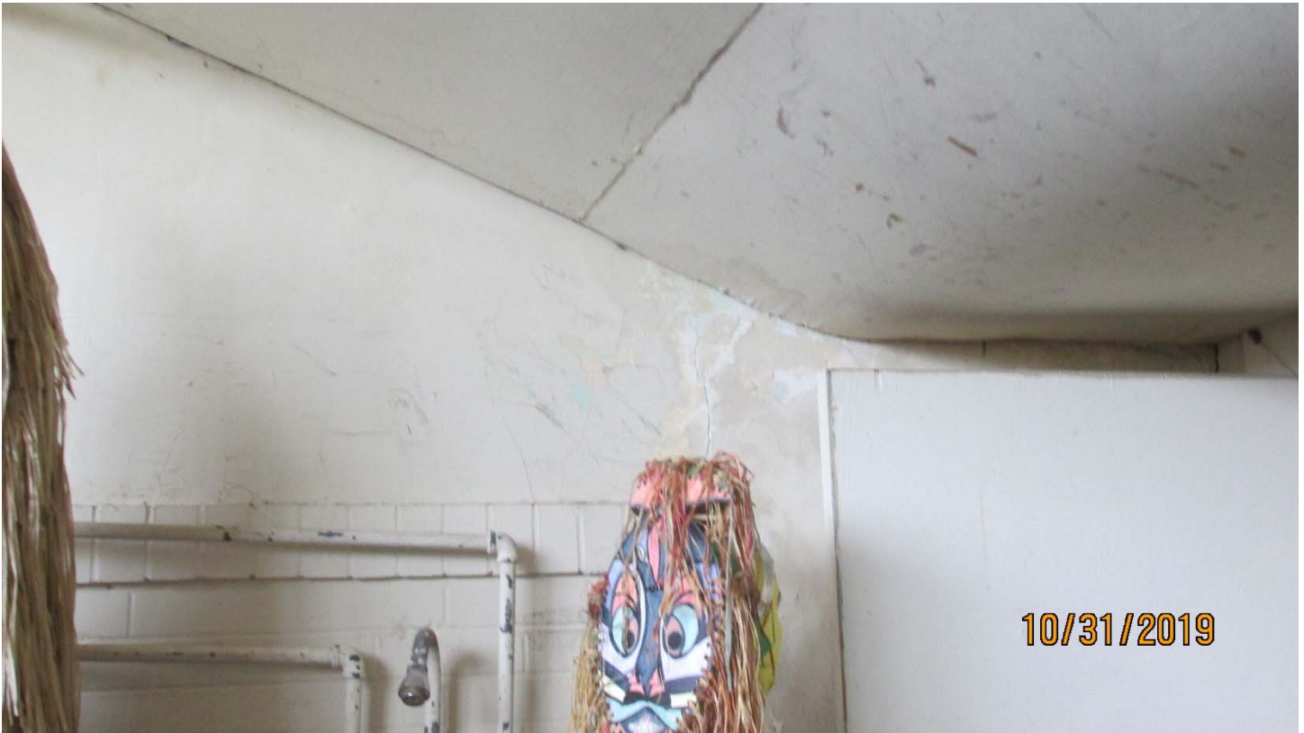
Picture #14: Cracks in Exterior Brick Wall – South End of Gymnasium underneath bleachers (DL-3)
