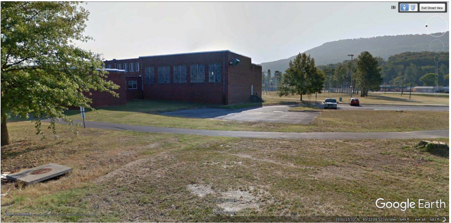
Picture #04: Partial Elevation – South End – Gymnasium Roof (Courtesy Google Earth)
