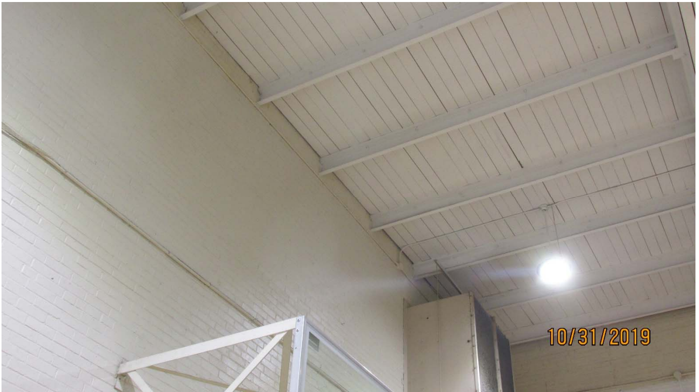
Picture #08: Roof framing – North Wall – Gymnasium
