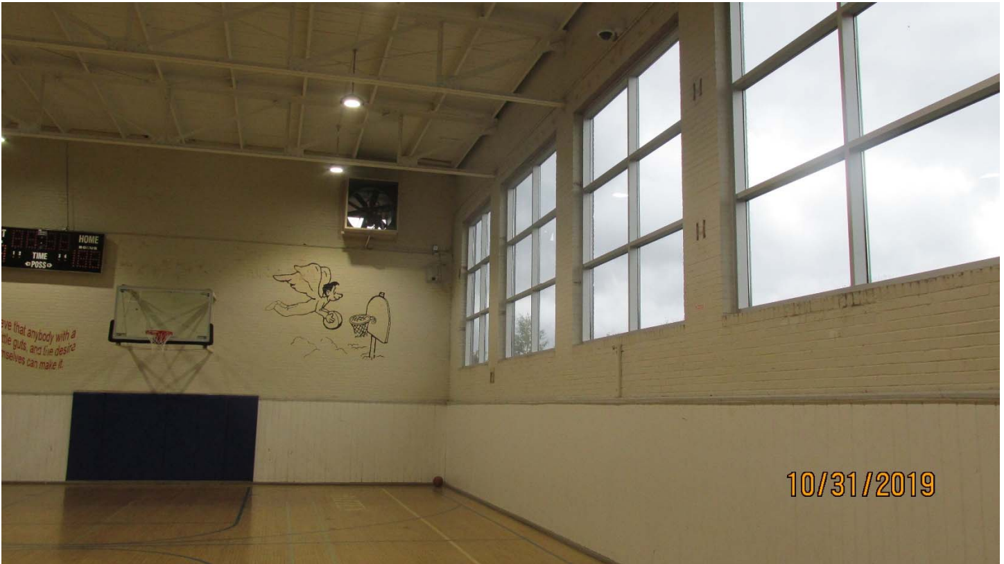
Picture #06: Interior Elevation – Southwest corner – Gymnasium
