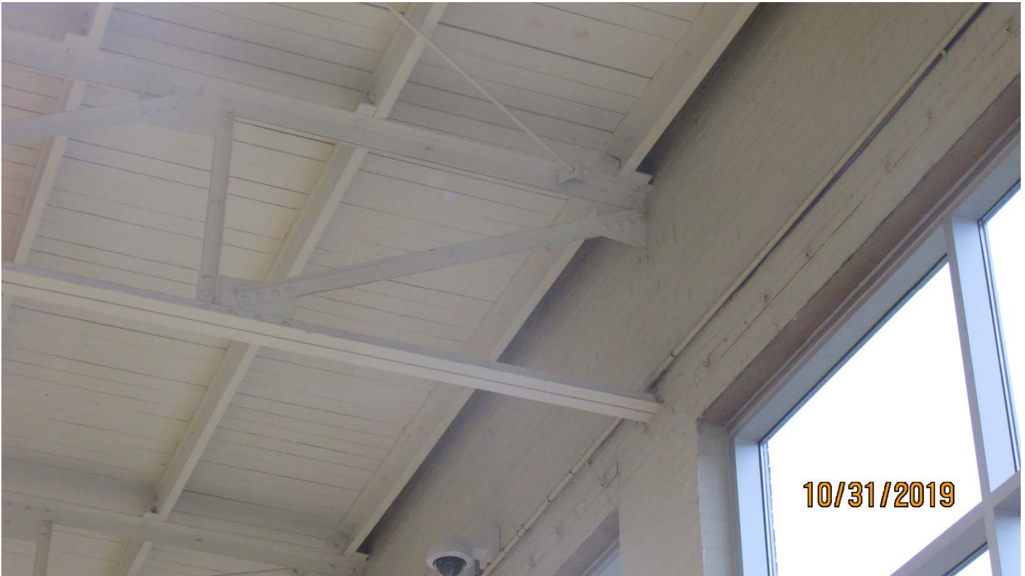
Picture #07: Roof framing – West Wall – Gymnasium
