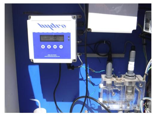
Description: Meter Reading Residual Chlorine, Temperature and pH of the Effluent
