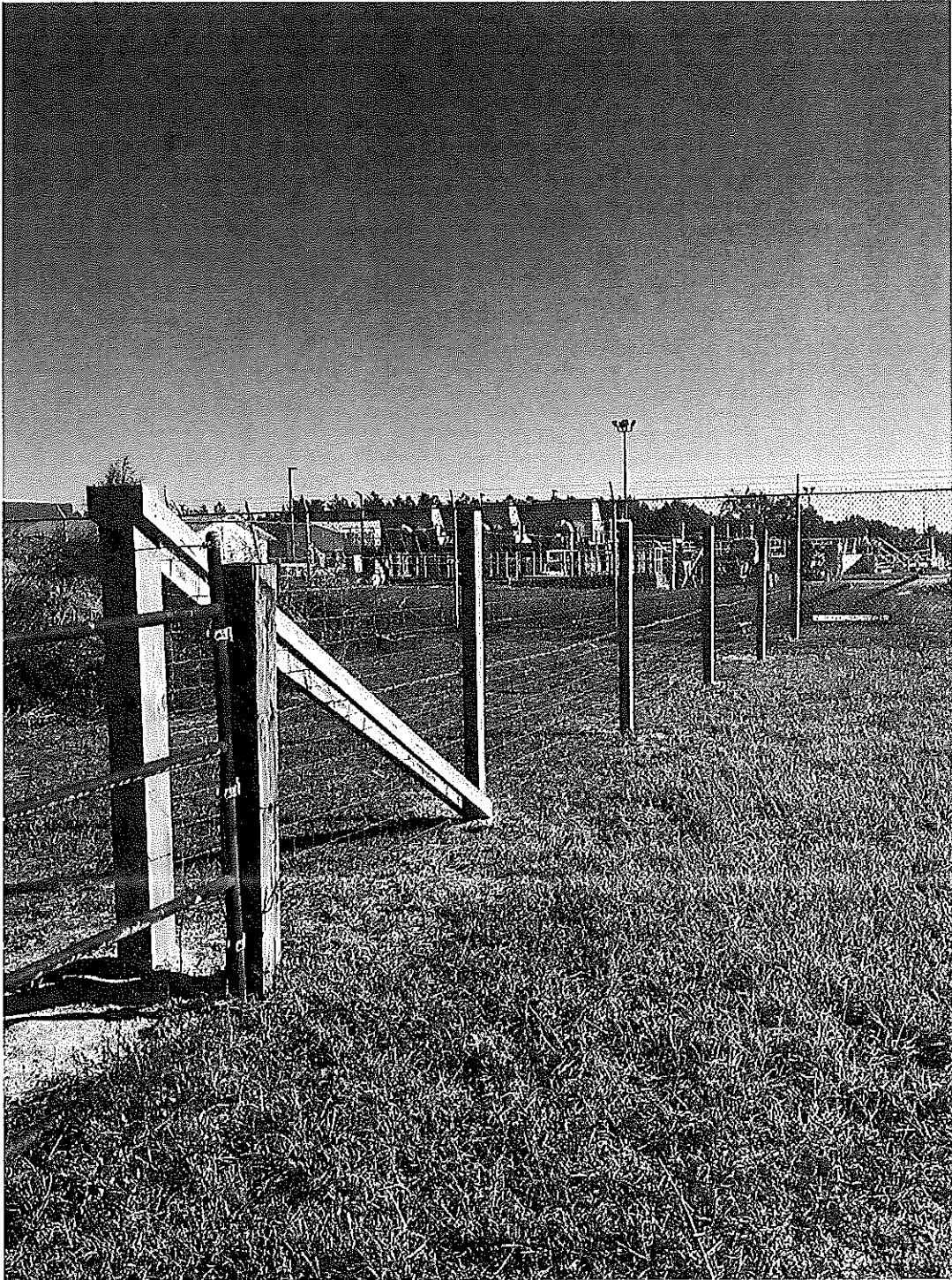
The gate is also in poor shape and scheduled for repairs.
