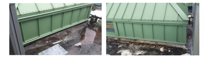
**Answer:** In the sections were there is no window system installed, install plywood sheets cut to fill the section, run the TPO up to the top of the plywood, and use a termination bar. Item to be paid under lump sum price for roofing installation. No additional money will be given for this item.
