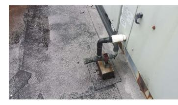
**Answer:** Please repair the drain connection that is currently in place. Connect a PVC connector to where the water is currently draining, extending new PVC pipe past the center window section, to allow the A/C unit to drain onto the roof at a location where it will not become trapped and can drain freely, preferably into a gutter. <u>An additional</u> pay item has been added to the bid <u>schedule for this work.</u>
