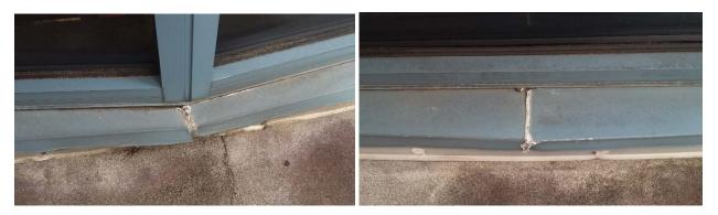
**Answer:** It was decided between the experts present that the best solution practicable was to seal the joint with a polyester mesh, 6" in width, coated with a urethane coating tinted to match the color of the metal. Coating to be turned down to the bottom of the flashing. A detail can be provided if requested. <u>An additional pay</u> item has been added to the bid schedule for this work.
