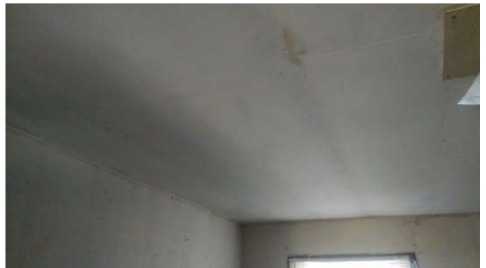
Photo 6 – Drywall and joint compound throughout ceilings and walls.
