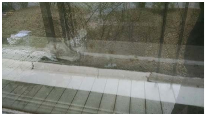
Photo 6 – Exterior window glazing.
