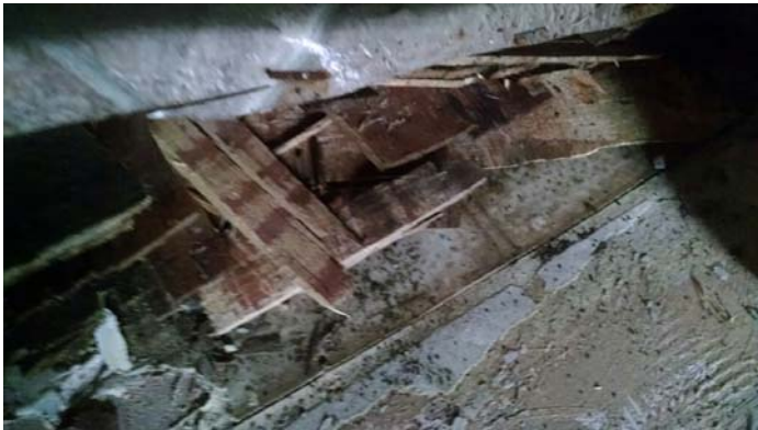
Photo 3 – Flooring under layer of sub-floor at kitchen entrance.
