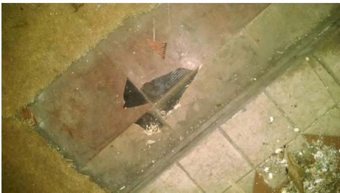
Photo 5 – 9"x9" floor tile and mastic in bedroom.
