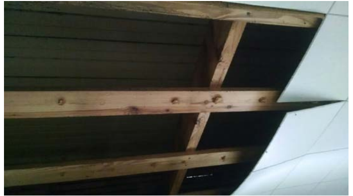
Photo 2 – 1'x1' ceiling tile in the living room.
