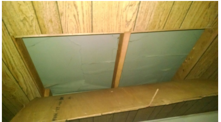
Photo 10 – Plaster with finish.
