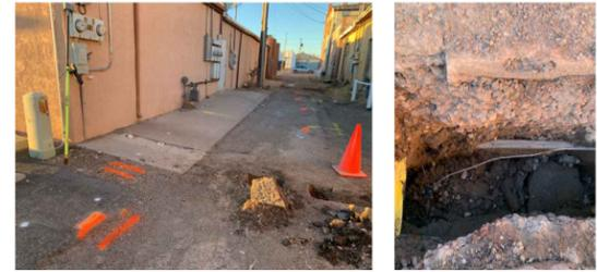
Remarks: 1.5"Ø black PVC communication conduit; approximately 1.21± of cover. Note yellow marking tap on gas line on left edge of Photo #2 (gas line below).
