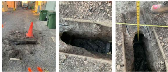
Remarks: 3"Ø black PVC communication conduit; approximately 1.89± of cover. Communication line located west of the gas line.
