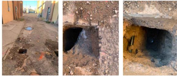
Remarks: Electric line is concrete encased just below alley asphalt surfacing. Concrete encasement is approximately 0.5' below finished alley surfacing.
