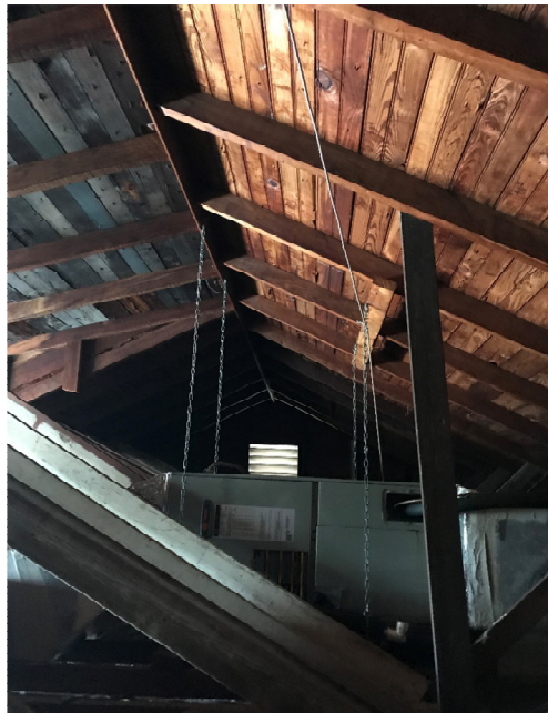
Picture showing rafters in attic with diagonal to wall below
