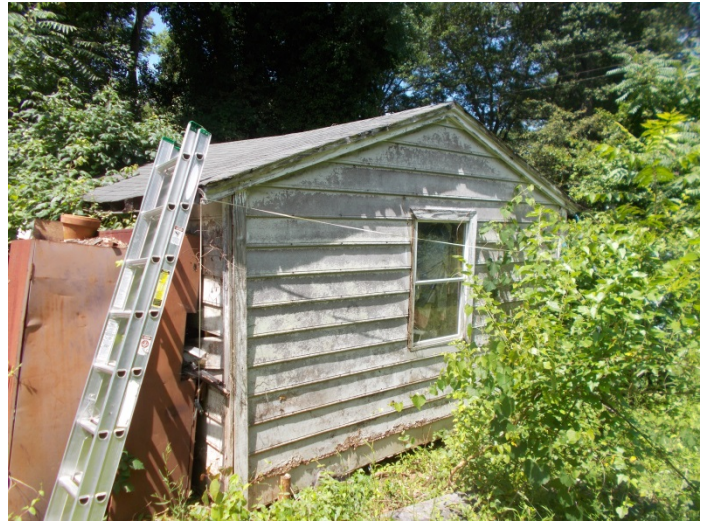
Photo 2 – Exterior shed in back yard.
