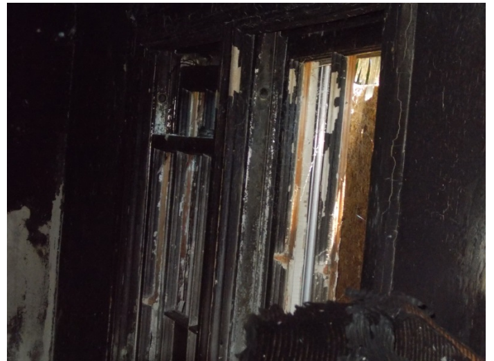
Photo 10 – Glazing on exterior wooden windows.
