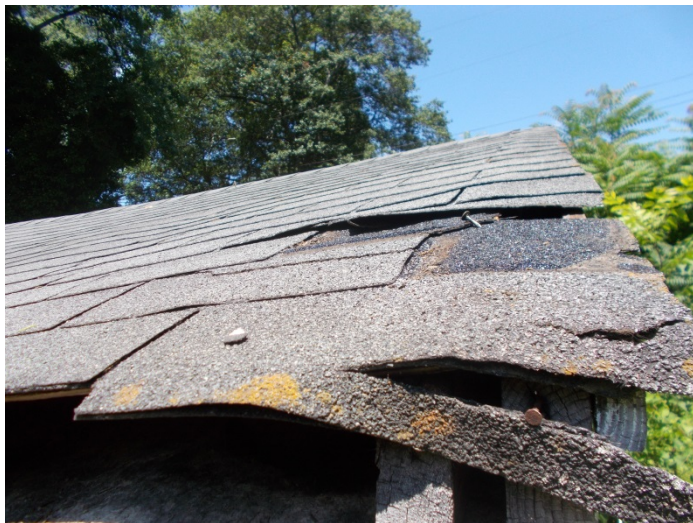
Photo 5 – Roofing shingles (2 layers) and no felt on main exterior shed roof.
