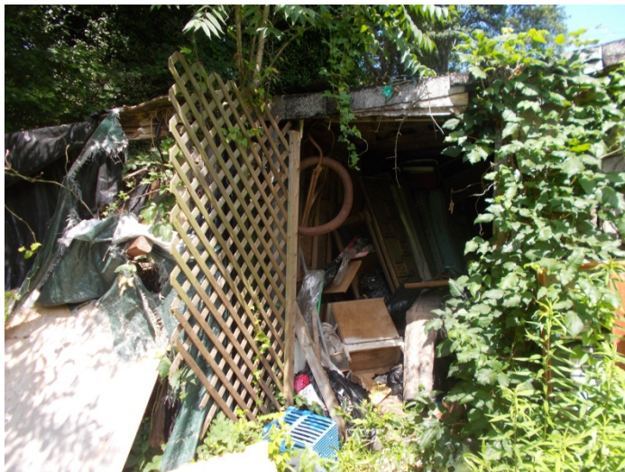
Photo 3 – Large amount of debris stacked in and around shed.
