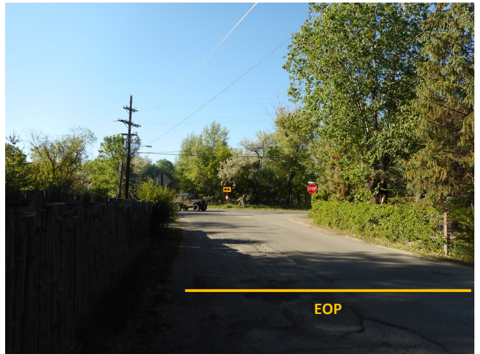
R. End of Project on Carabajal Road- Facing South
