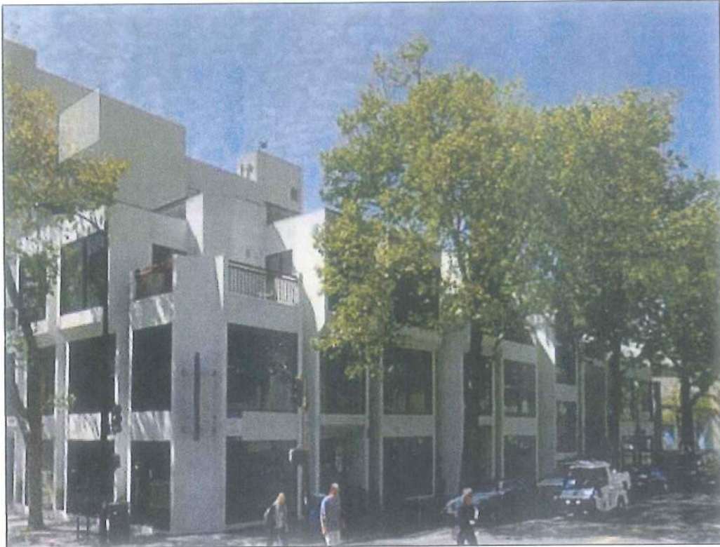
View of Project Site: Corner of Center Street and Milvia Street
