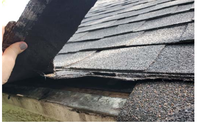
Photo 2 – Vinyl paper under shingles.
