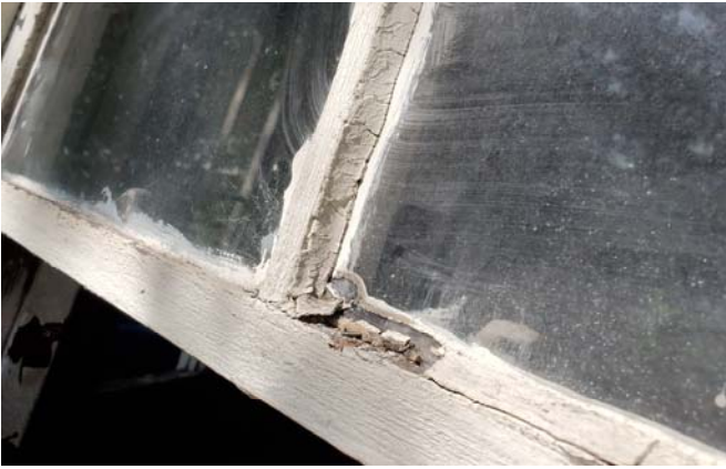
Photo 3 – Exterior window glazing.
