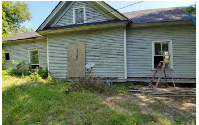
Photo 6 – Side view of structure.
