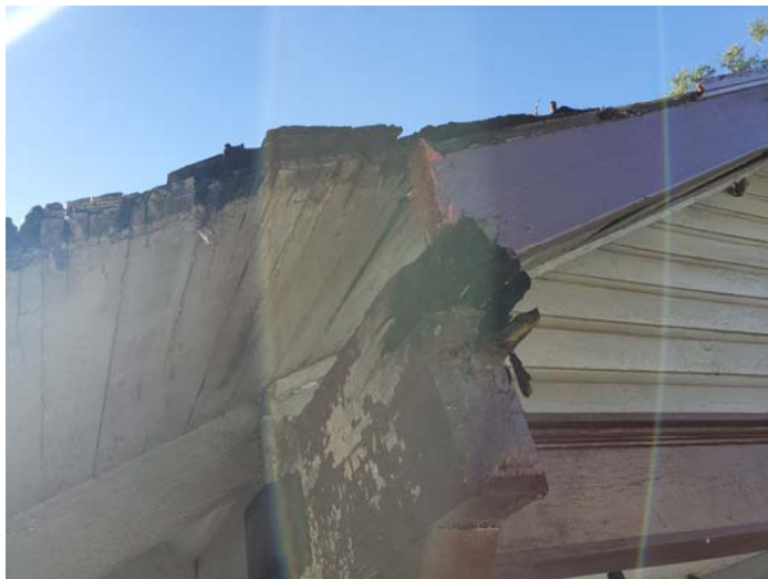
Photo 3 – Shingles with no felt.
