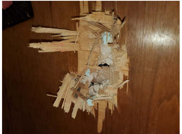
Photo 8 – Plaster with finish under wood paneling on walls throughout.
