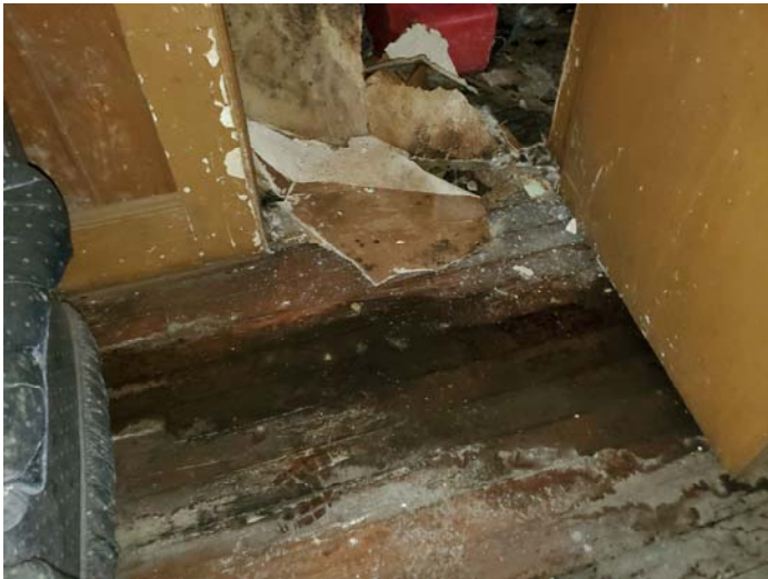
Photo 9 – Wood floors throughout.
