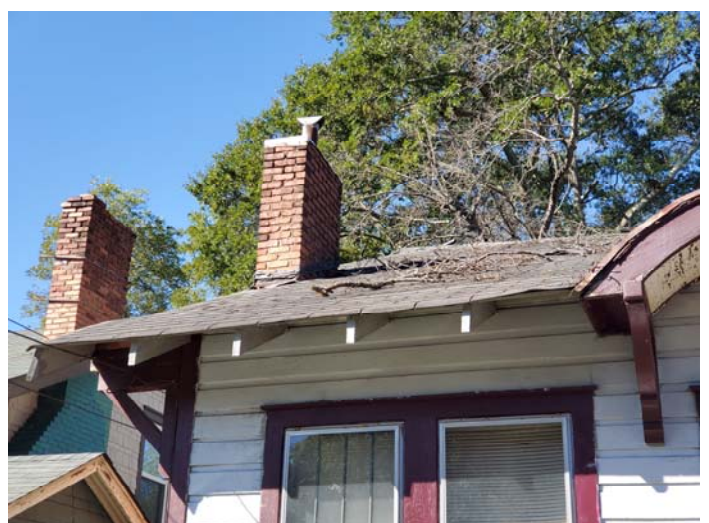
Photo 6 – Assumed ACM on chimney.
