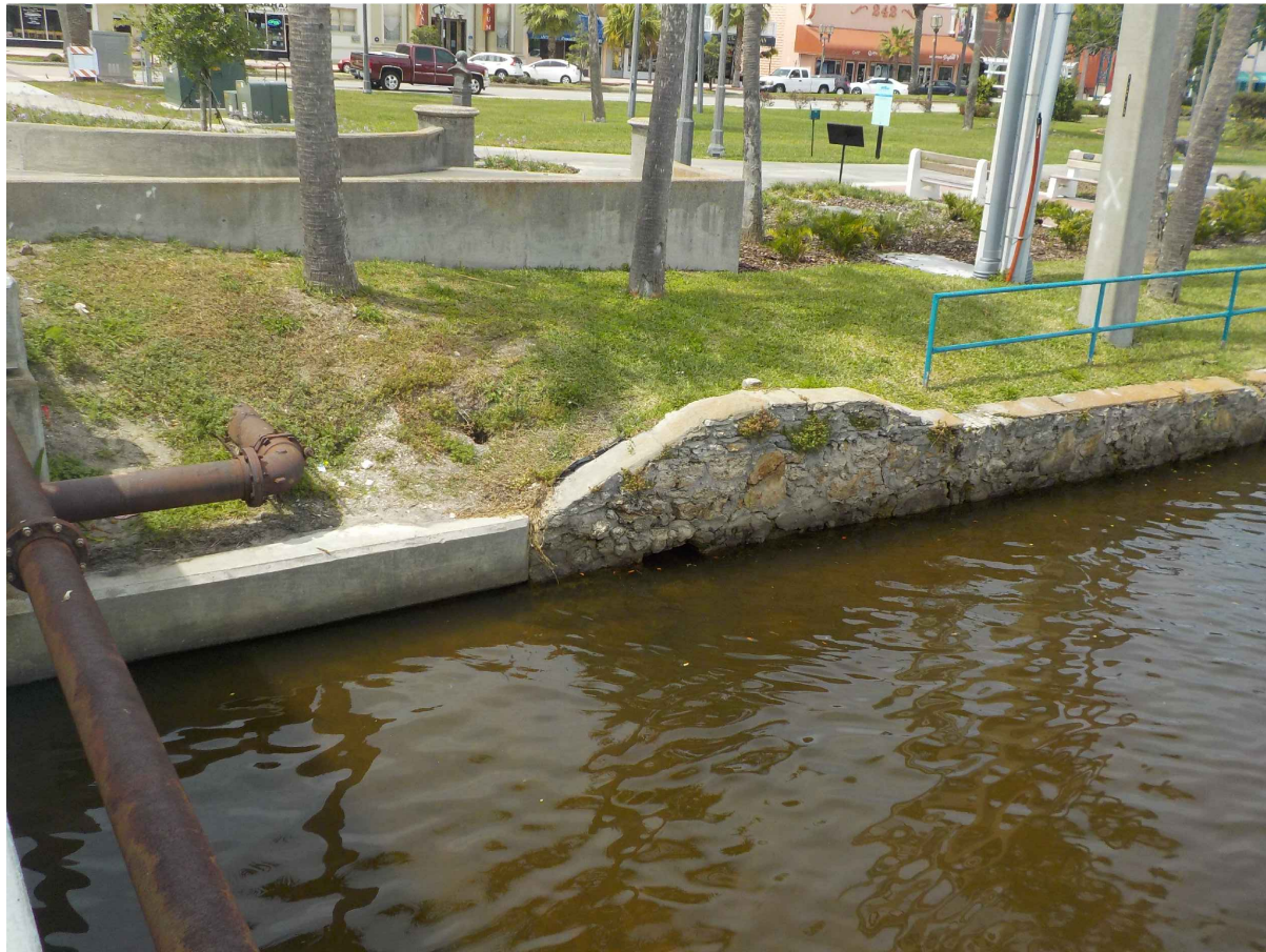
EXISTING BULKHEAD AND BRIDGE ABUTMENT AT ORANGE AVENUE DMC, 03.24.2019
