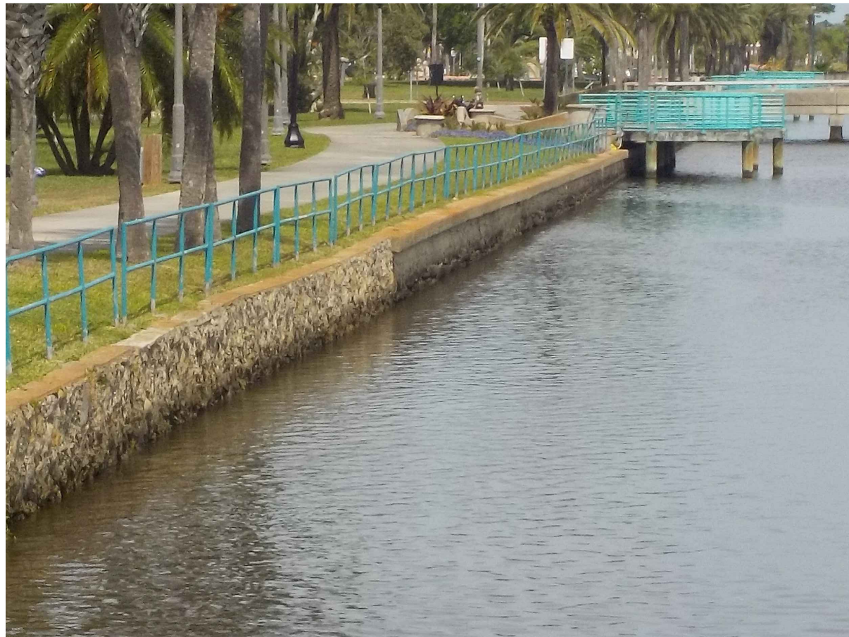
EXISTING BULKHEAD LOOKING NORTH FROM ORANGE AVENUE DMC, 03.24.2019
