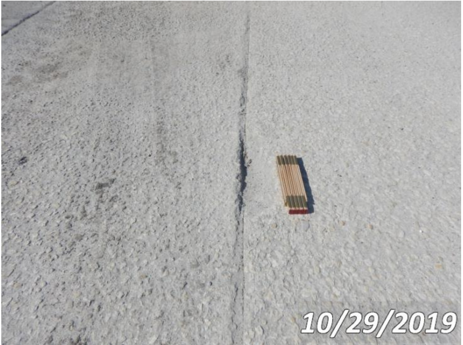
Photo 38-S03 (Unit 0: Re Concrete Slab)
