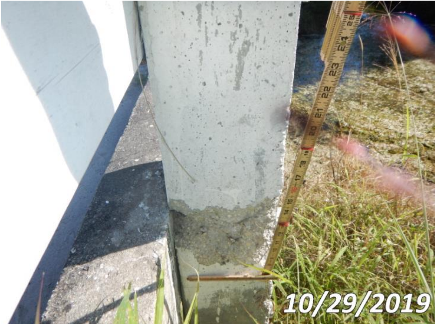
Photo 333-S01 (Unit 0: Other Bridge Railing)
