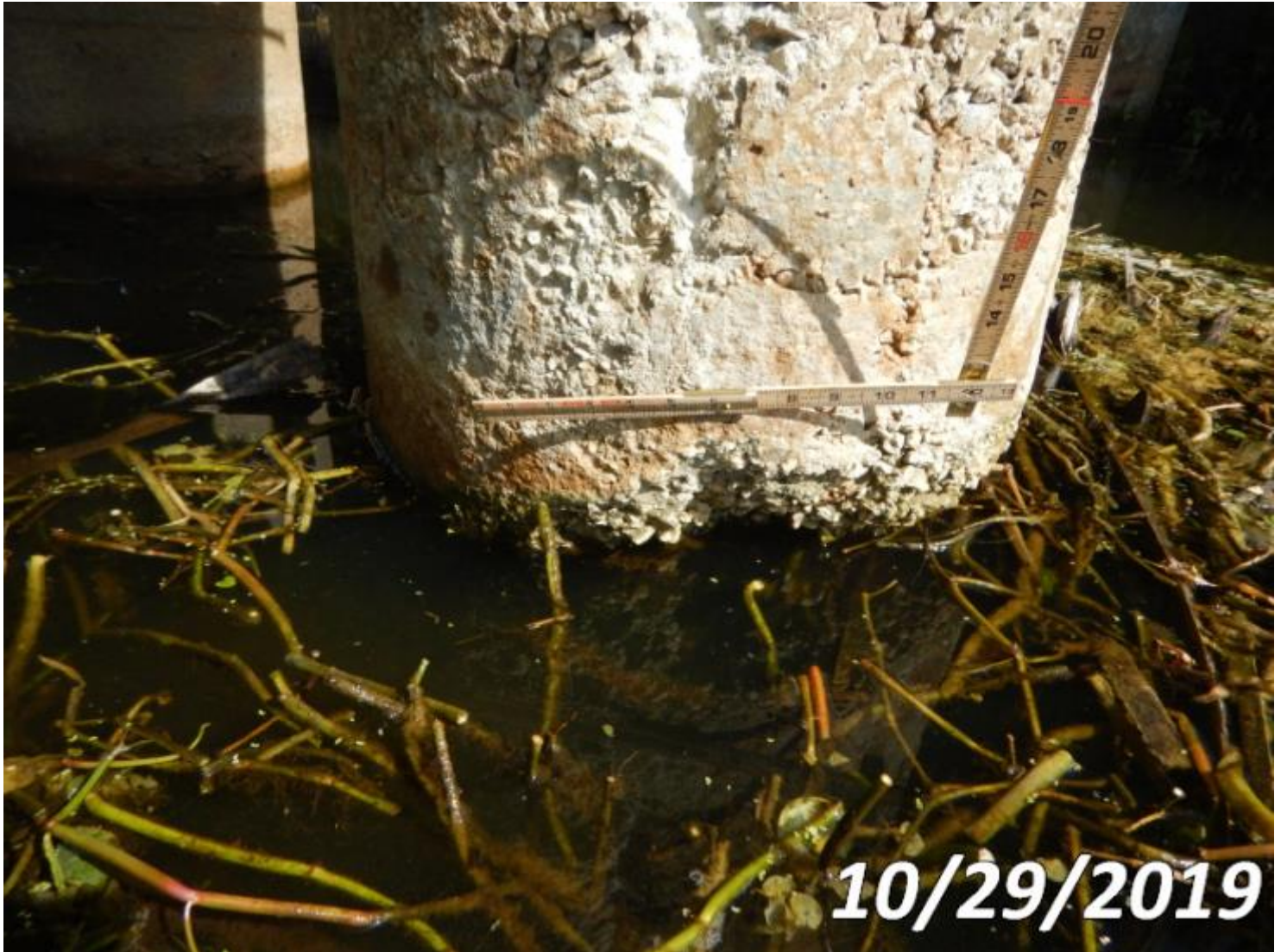
Photo 8298-S01 (Unit 0: Pile Jacket Bare)
