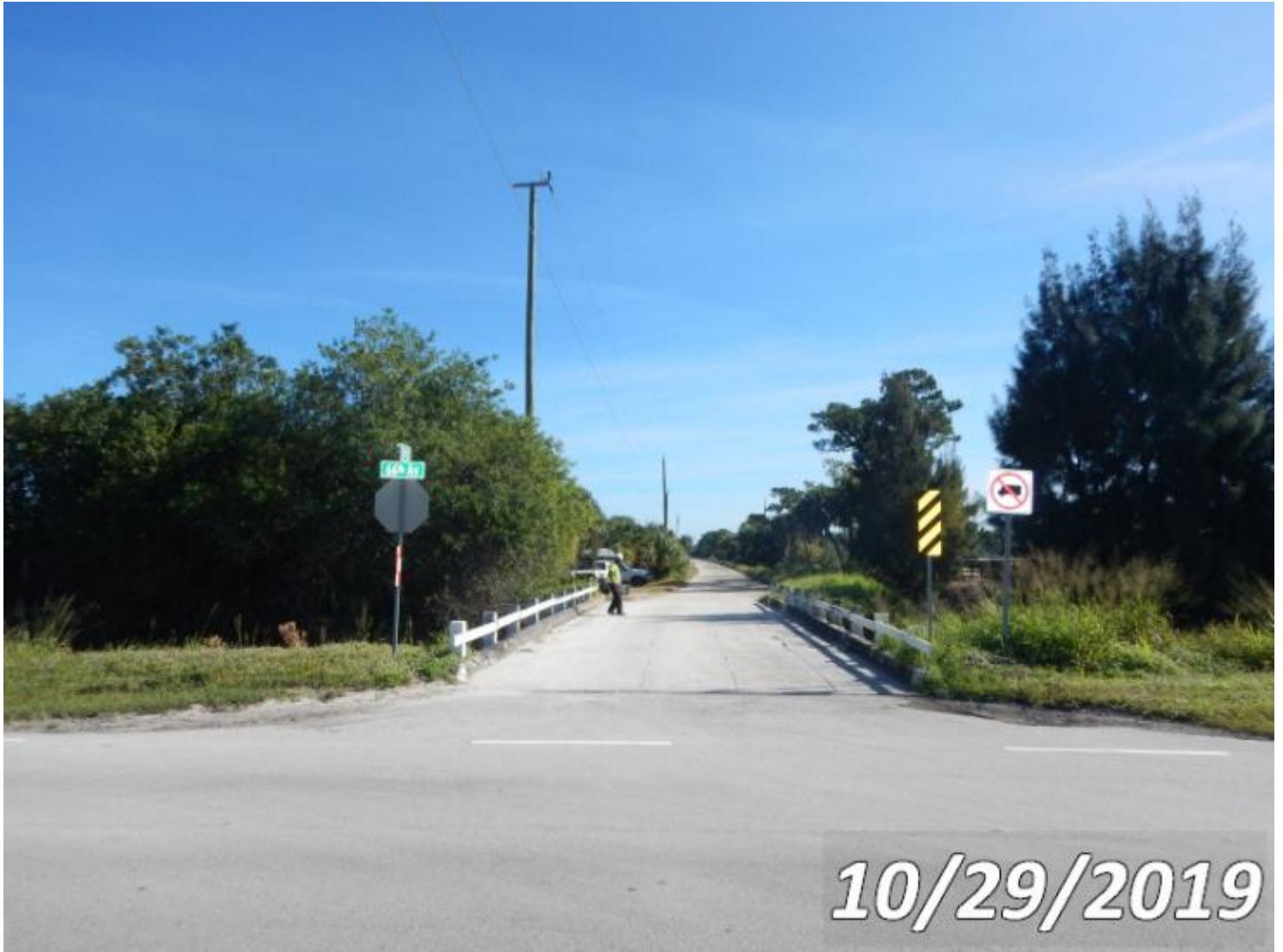
Photo 38-S09 (Unit 0: Re Concrete Slab)
