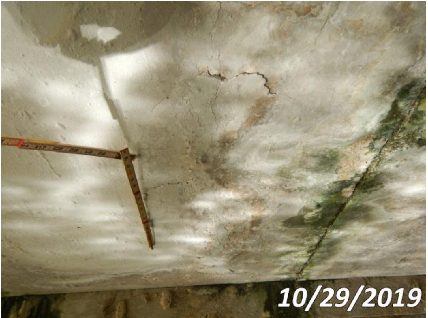
Photo 38-S05 (Unit 0: Re Concrete Slab)
