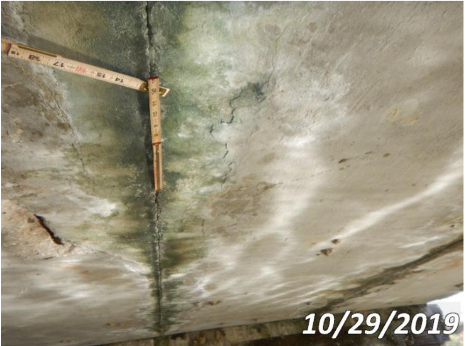
Photo 38-S06 (Unit 0: Re Concrete Slab)
