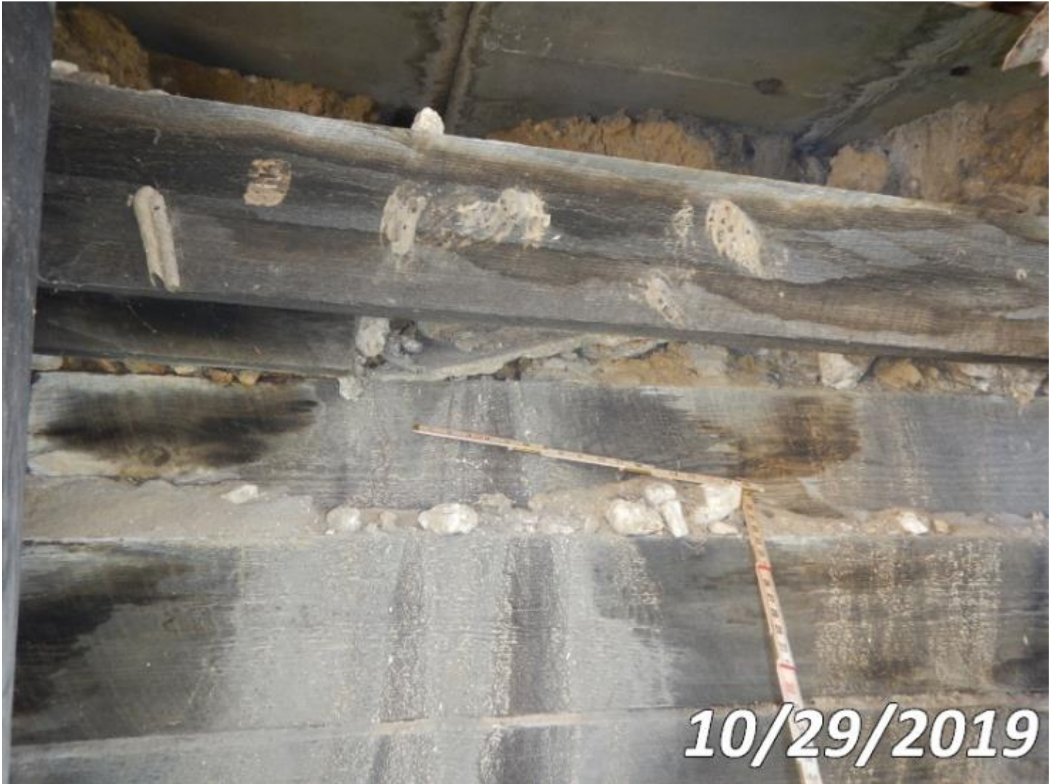
Photo 8395-S01 (Unit 0: Timber Abutment Slope Protection)
