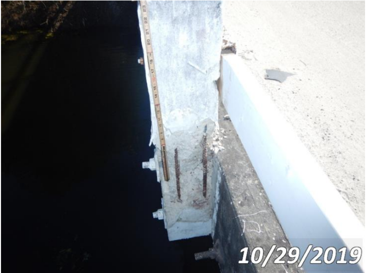
Photo 333-S02 (Unit 0: Other Bridge Railing)
