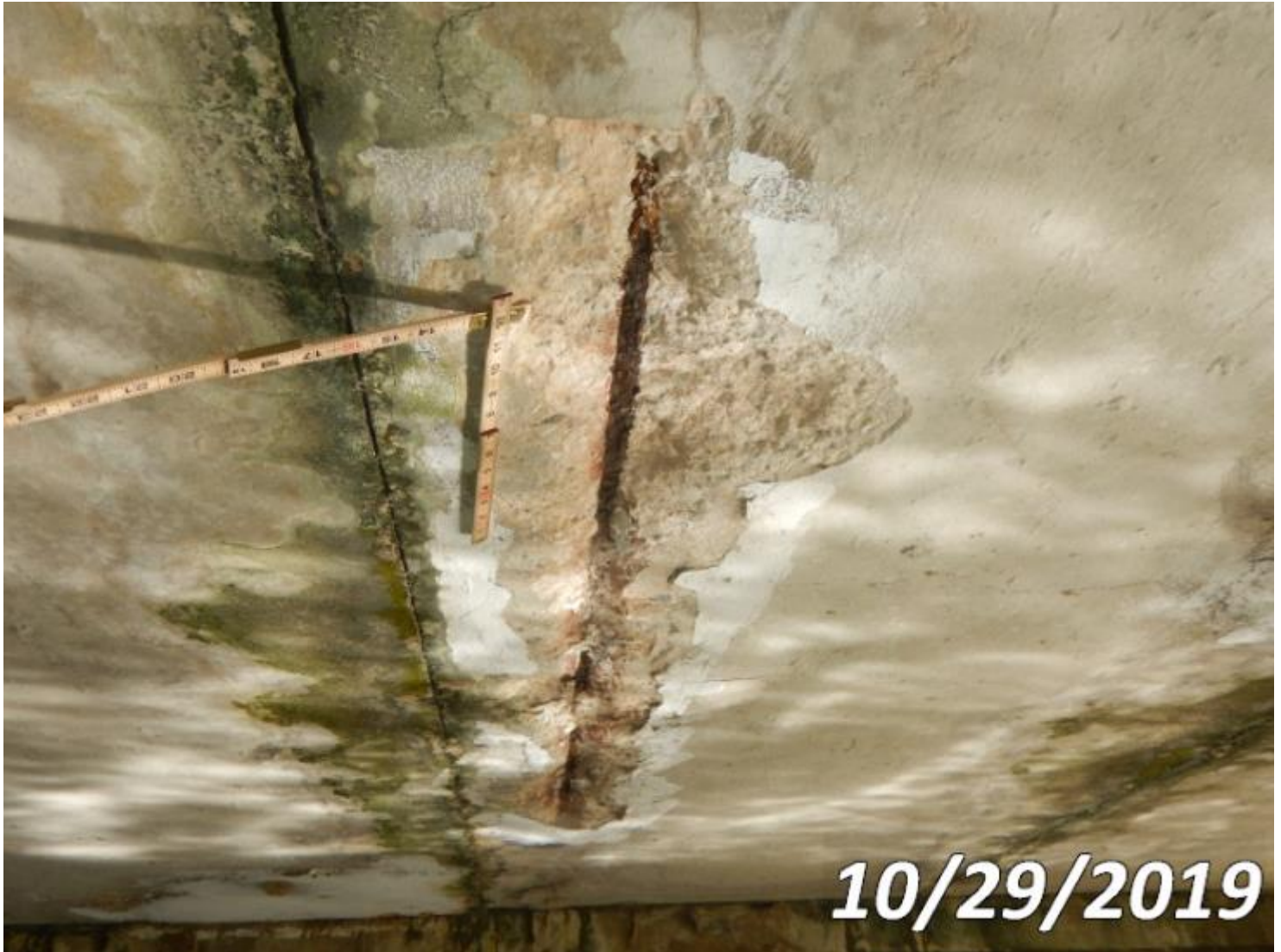
Photo 38-S01 (Unit 0: Re Concrete Slab)
