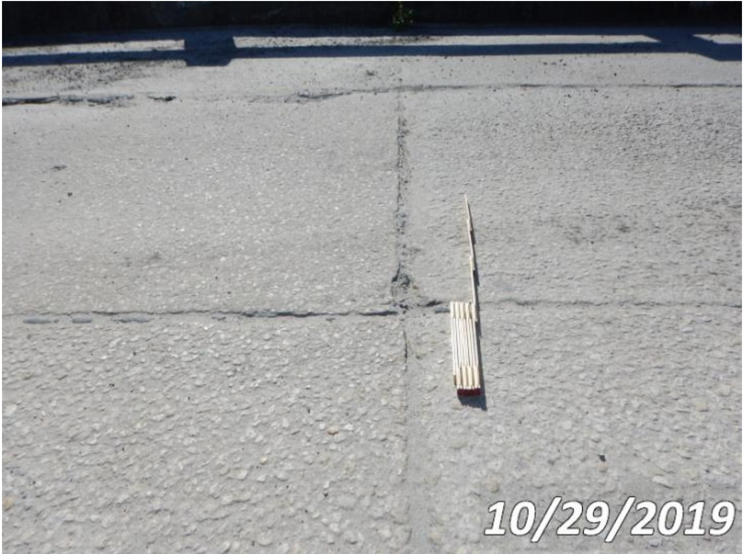
Photo 301-S01 (Unit 0: Pourable Joint Seal)
