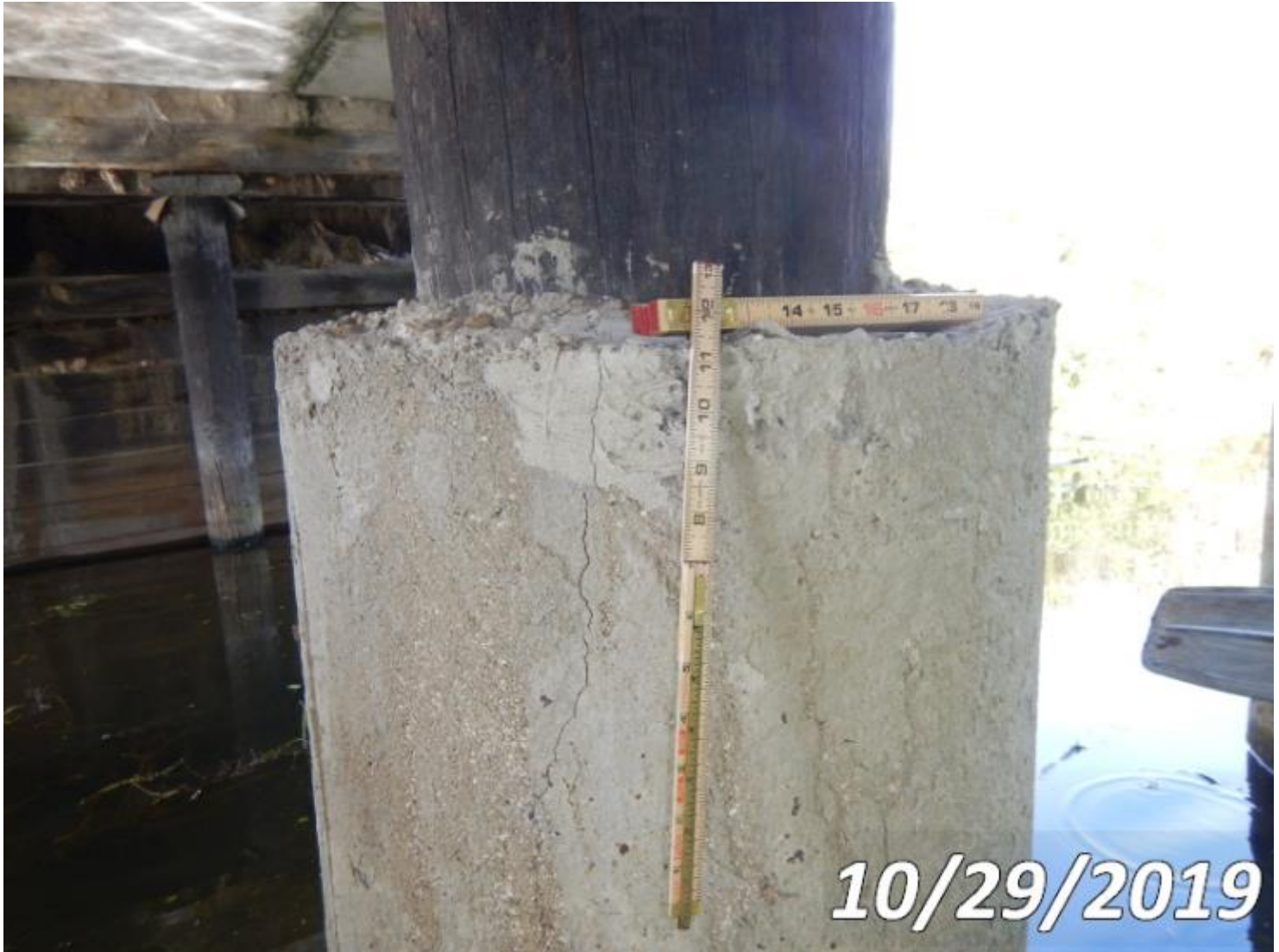
Photo 8298-S02 (Unit 0: Pile Jacket Bare)
