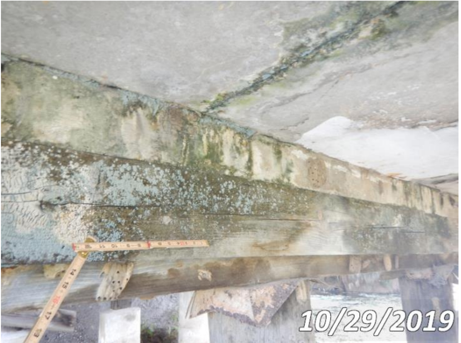
Photo 235-S01 (Unit 0: Timber Pier Cap)
