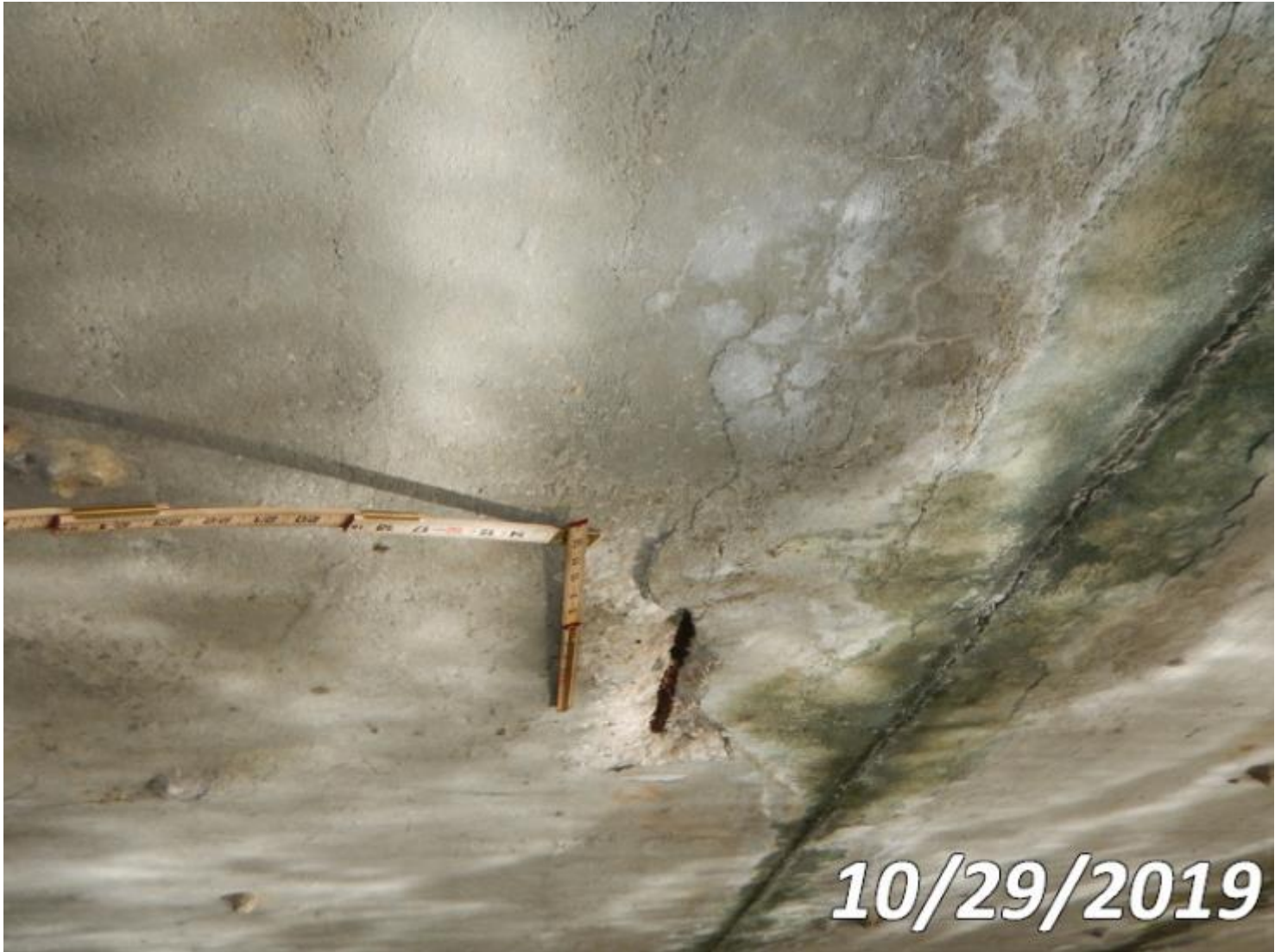
Photo 38-S02 (Unit 0: Re Concrete Slab)
