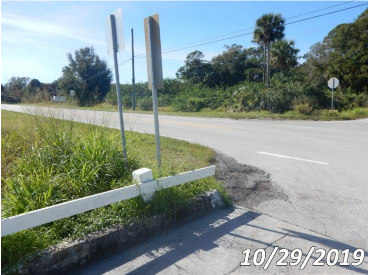
Photo 333-S03 (Unit 0: Other Bridge Railing)
