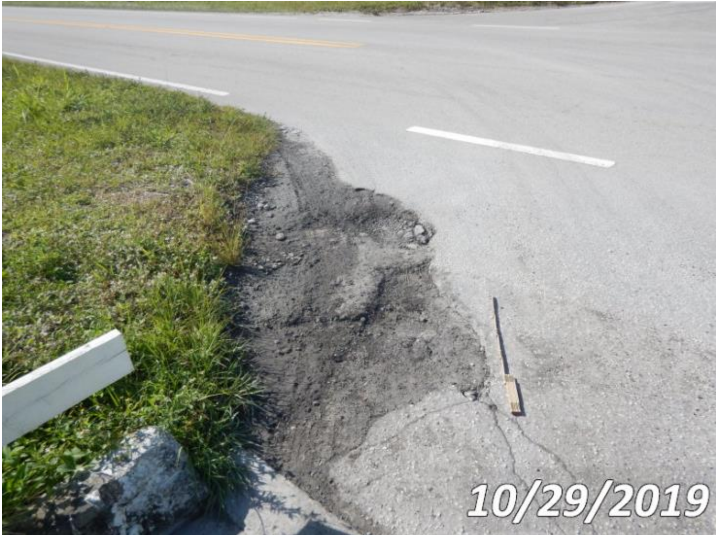
Photo 38-S08 (Unit 0: Re Concrete Slab)
