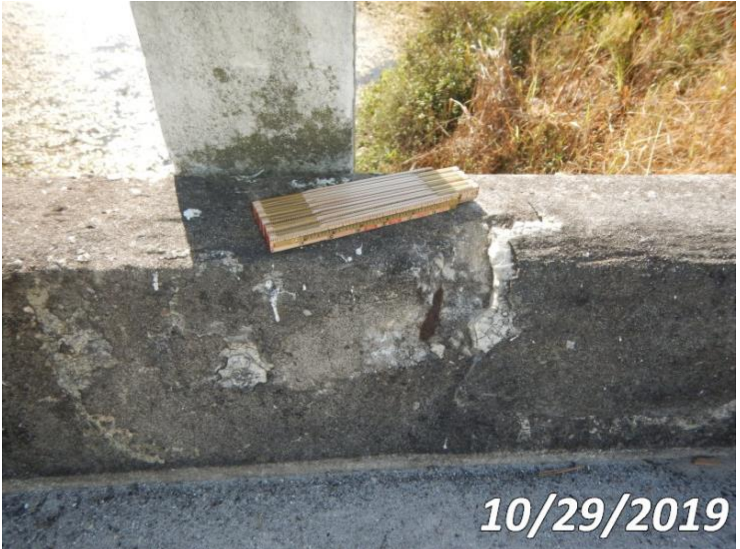
Photo 38-S07 (Unit 0: Re Concrete Slab)
