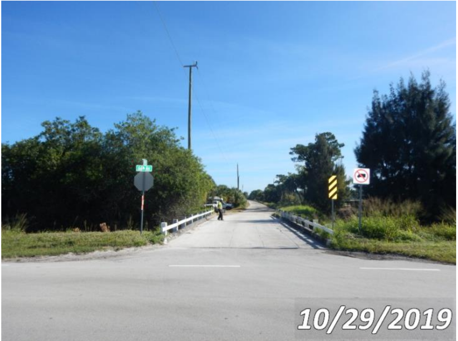
WEST APPROACH LOOKING EAST
