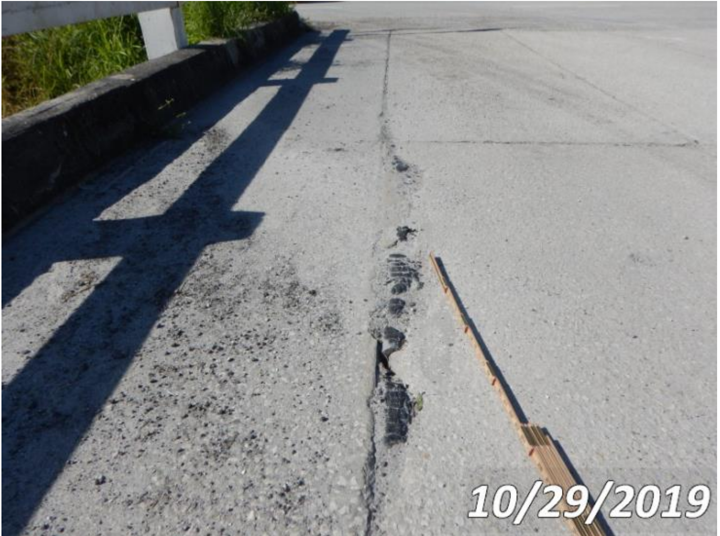
Photo 38-S04 (Unit 0: Re Concrete Slab)
