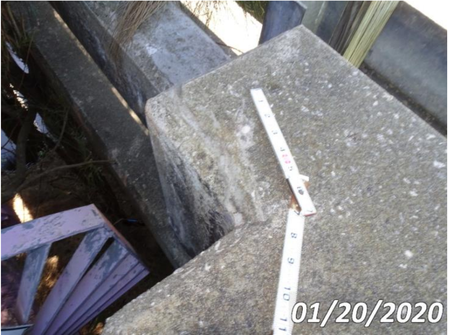
Photo 321-S01 (Unit 0: Re Conc Approach Slab)
