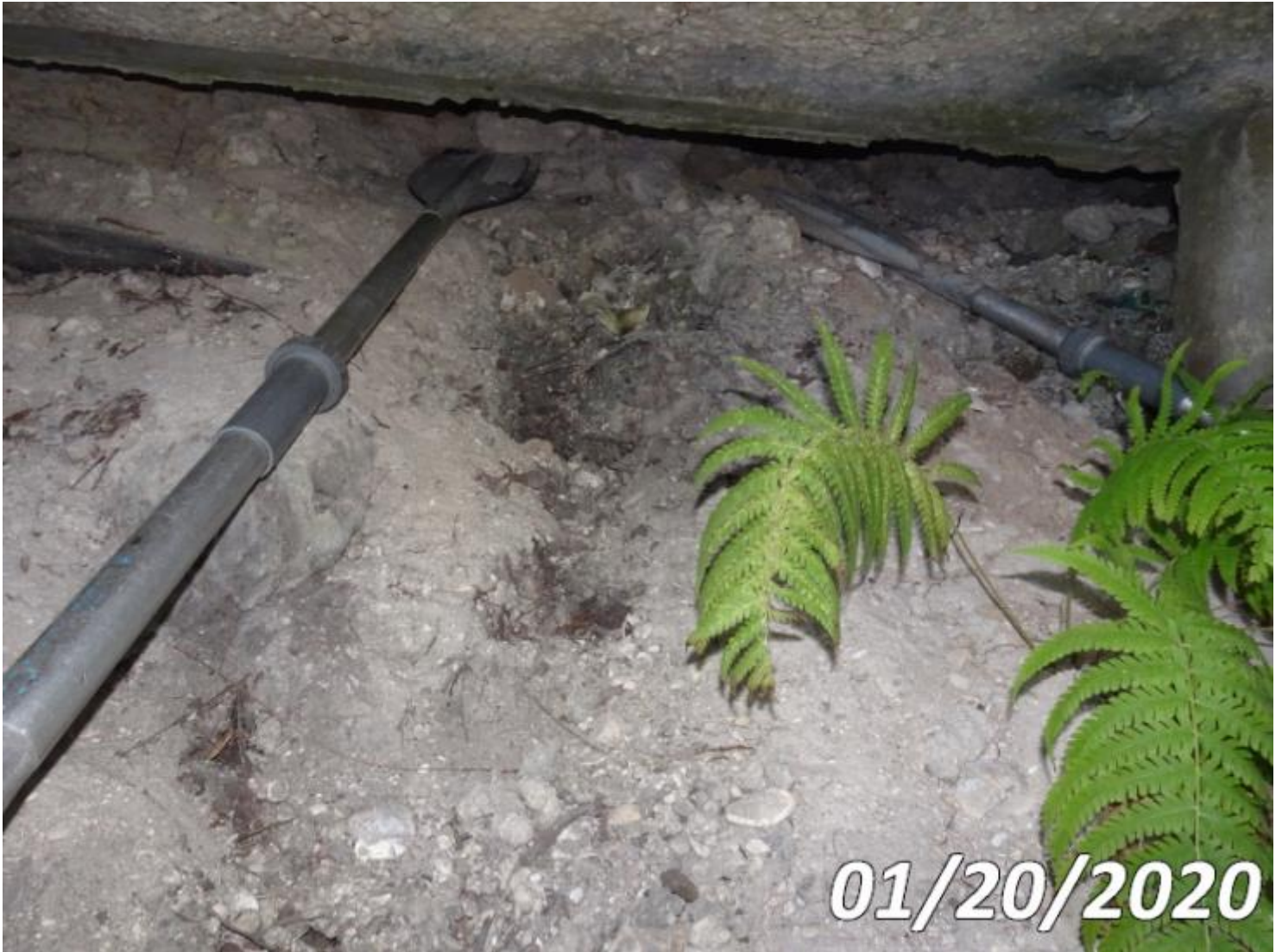
Photo 8290-S02 (Unit 0: Channel) & (Unit 0: Re Conc Approach Slab)
