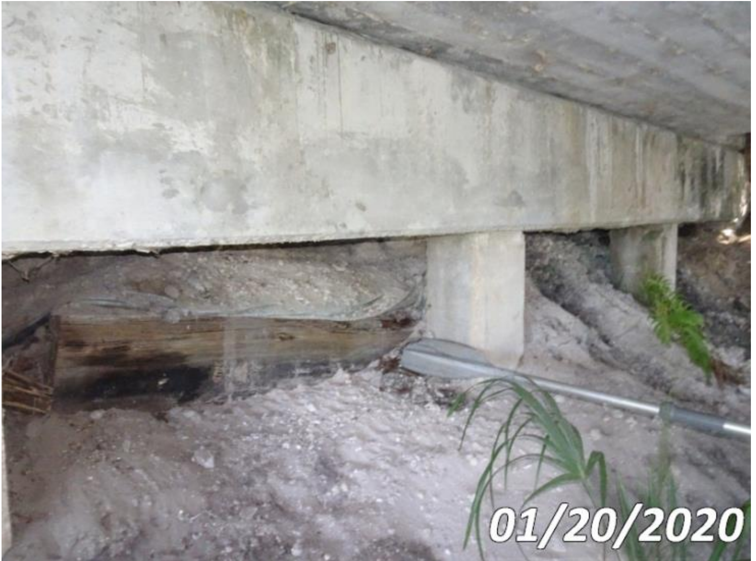
Photo 8290-S01 (Unit 0: Channel) & (Unit 0: Timber Walls)
