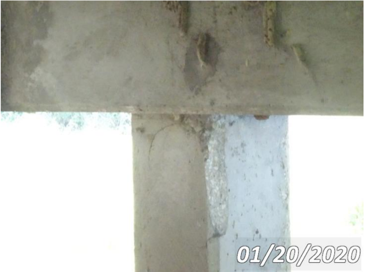
Photo 227-S01 (Unit 0: Re Conc Pile)
