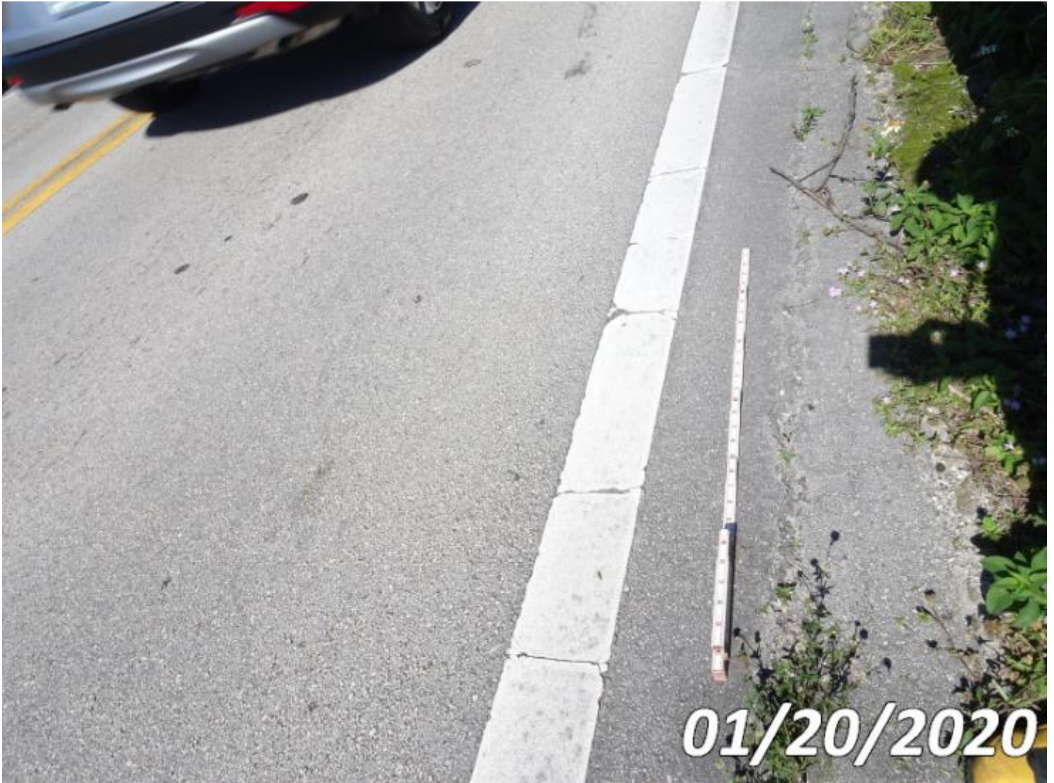
Photo 321-S03 (Unit 0: Re Conc Approach Slab)
