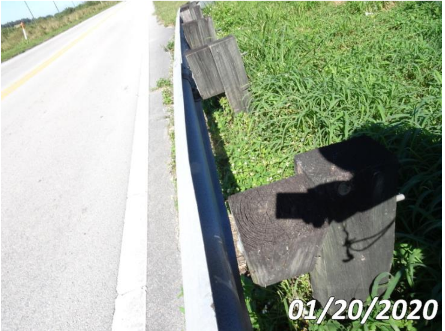
Photo 321-S02 (Unit 0: Re Conc Approach Slab)
