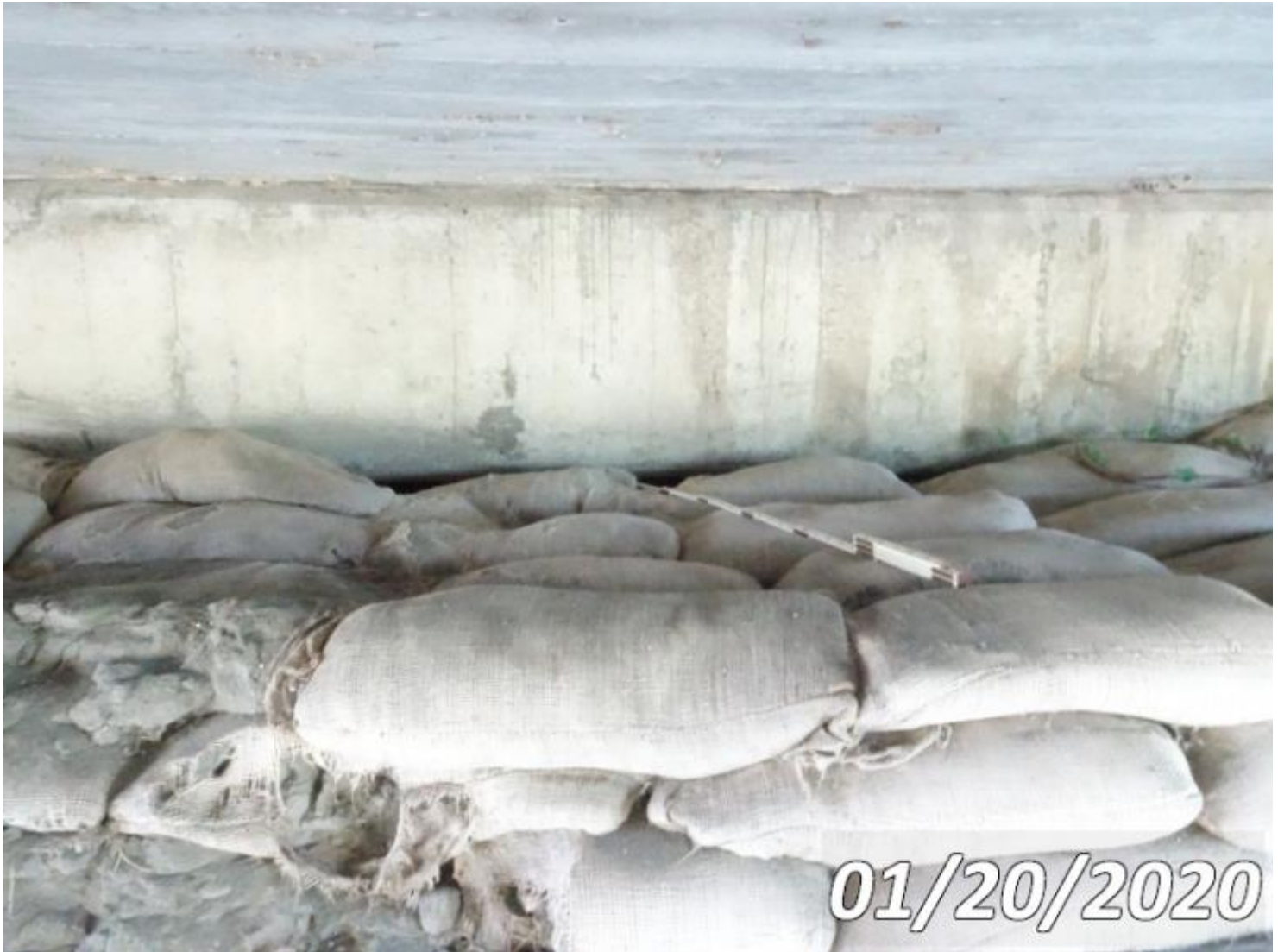
Photo 215-S02 (Unit 0: Re Conc Abutment)
