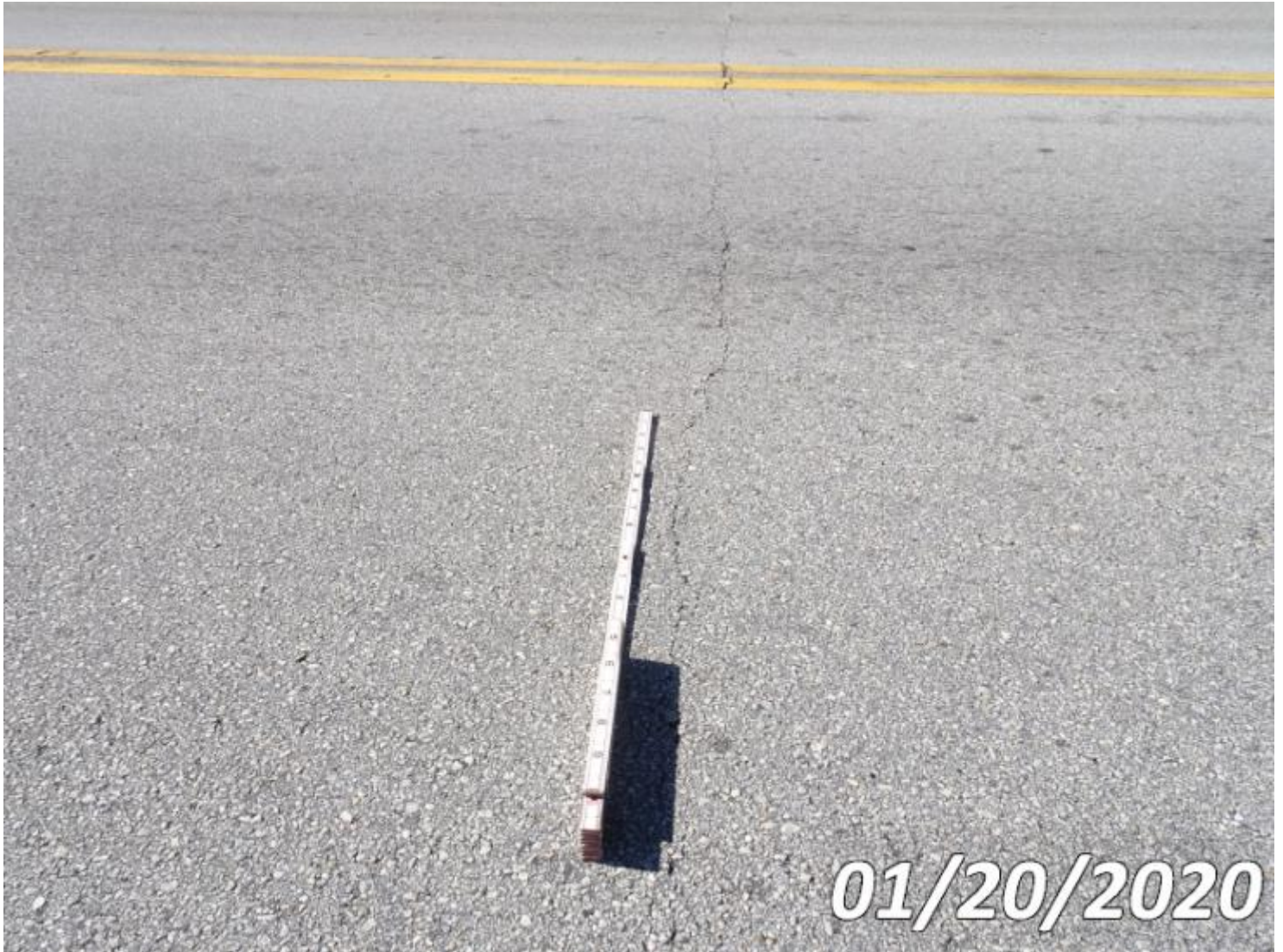
Photo 38-S03 (Unit 0: Re Concrete Slab)
