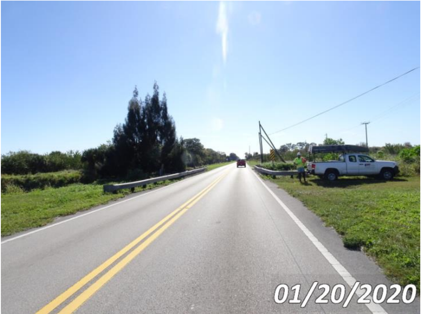
NORTH APPROACH LOOKING SOUTH
