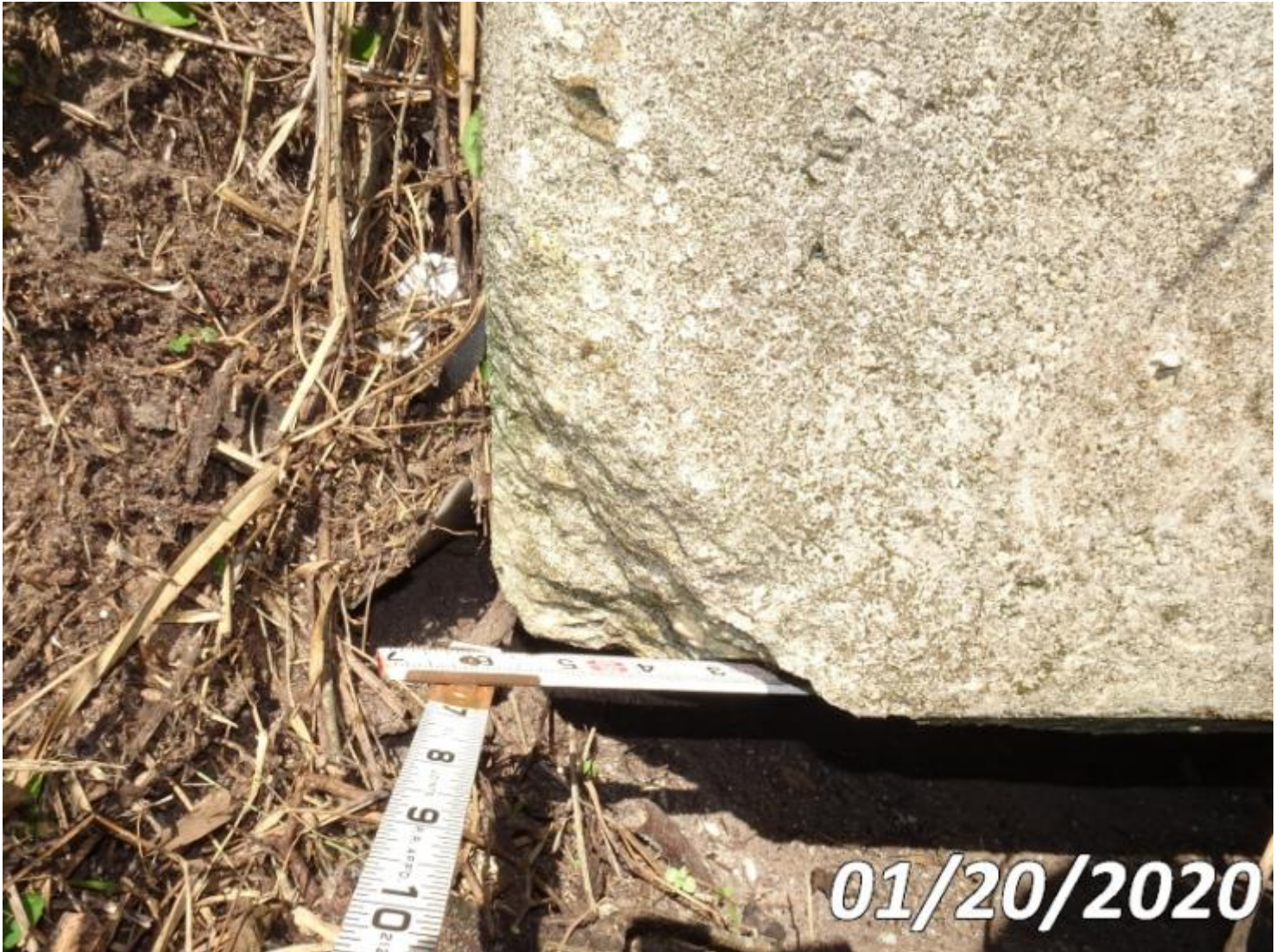
Photo 215-S01 (Unit 0: Re Conc Abutment)
