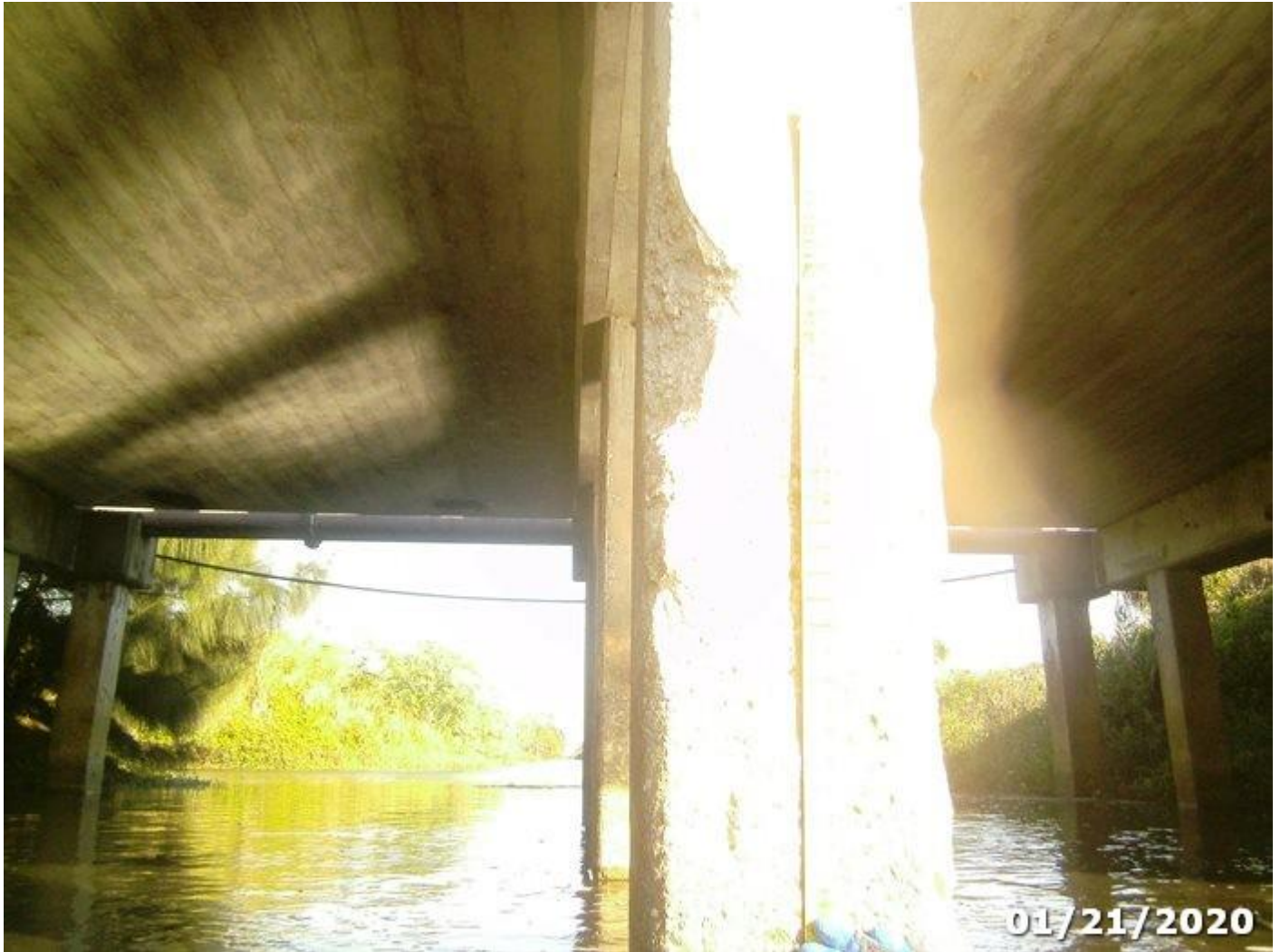
Photo 227-U02 (Unit 0: Re Conc Pile)
