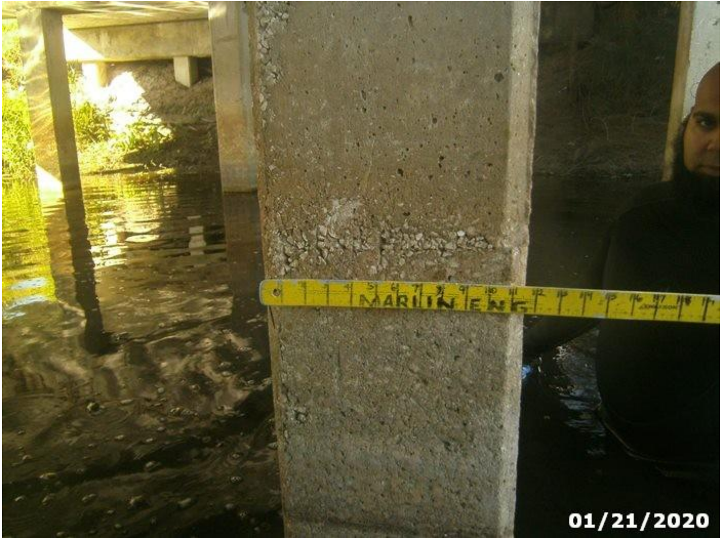
Photo 227-U04 (Unit 0: Re Conc Pile)
