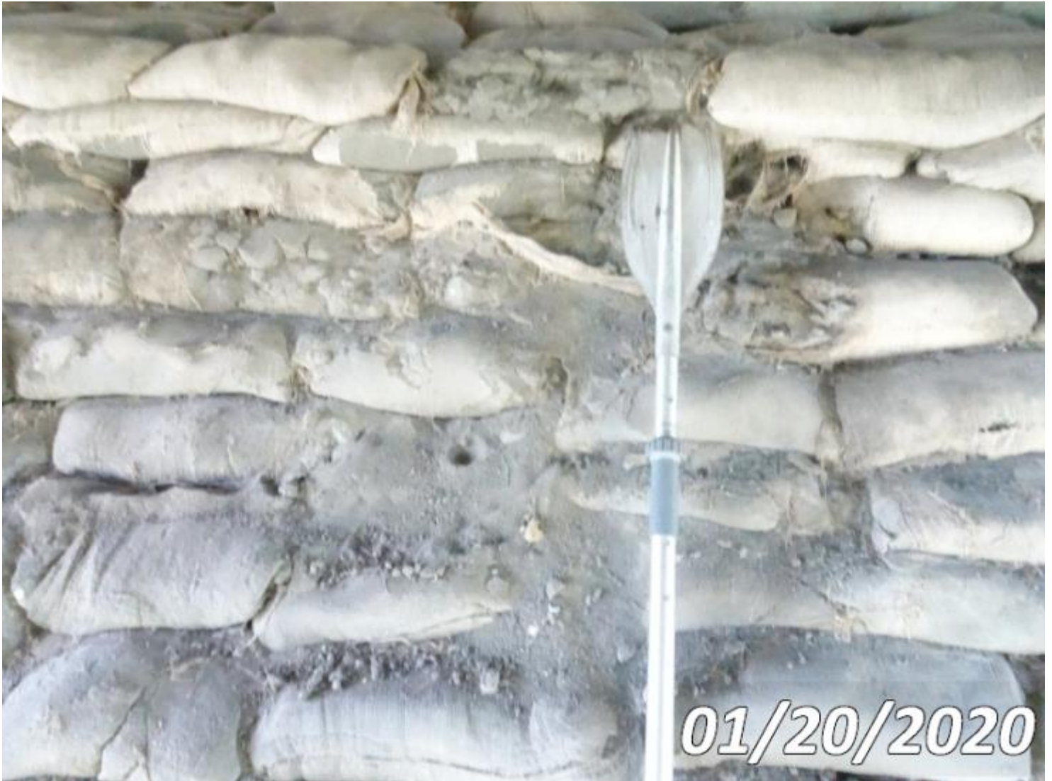
Photo 8396-S01 (Unit 0: Other Abutment Slope Protection)
