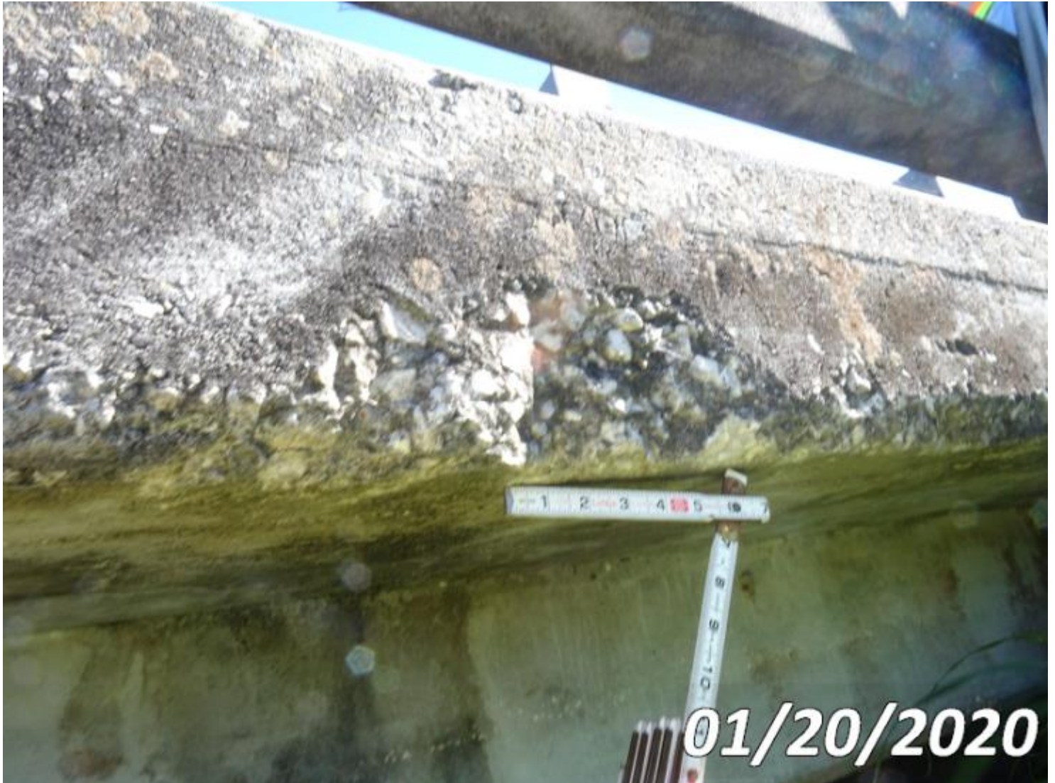
Photo 38-S01 (Unit 0: Re Concrete Slab)
