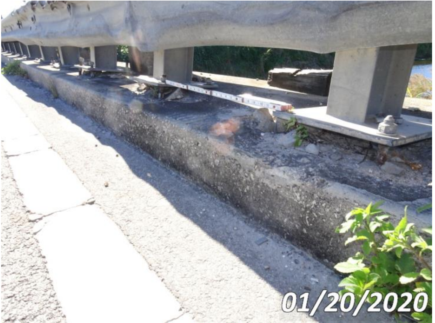
Photo 38-S02 (Unit 0: Re Concrete Slab)
