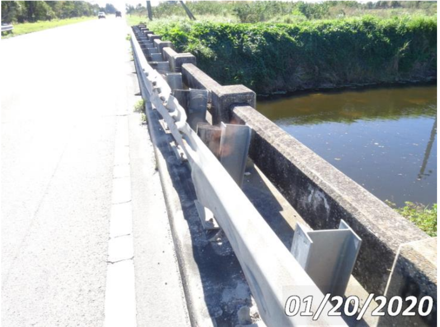
Photo 330-S01 (Unit 0: Metal Bridge Railing)
