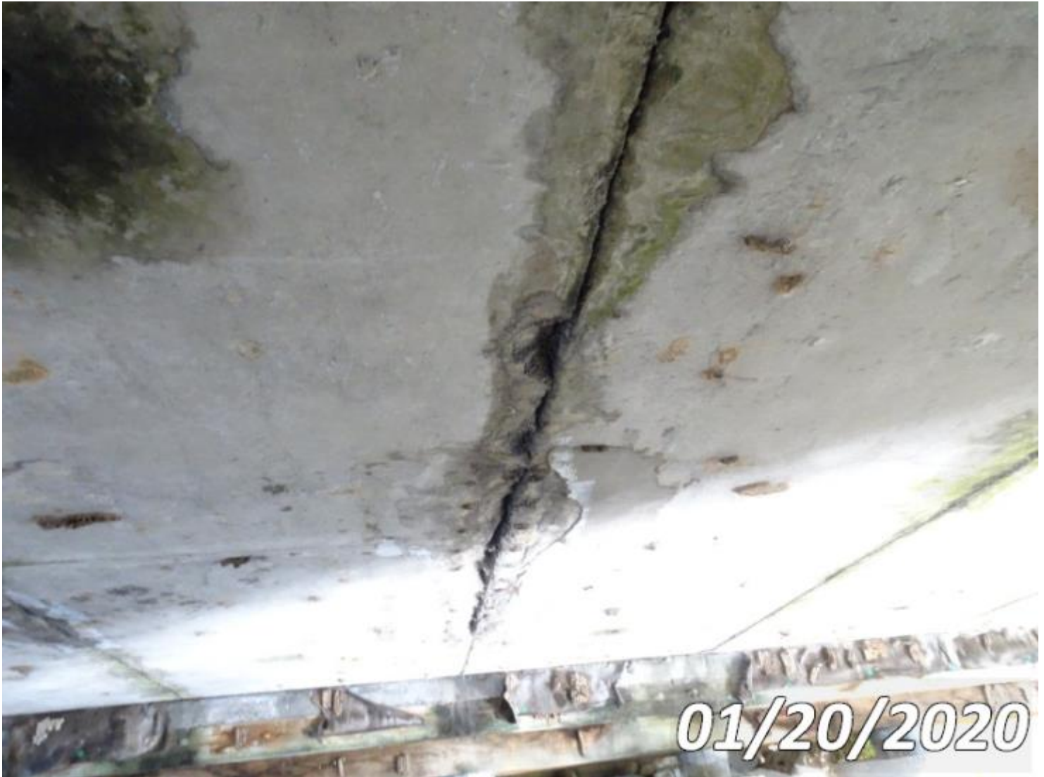
Photo 38-S05 (Unit 0: Re Concrete Slab)
