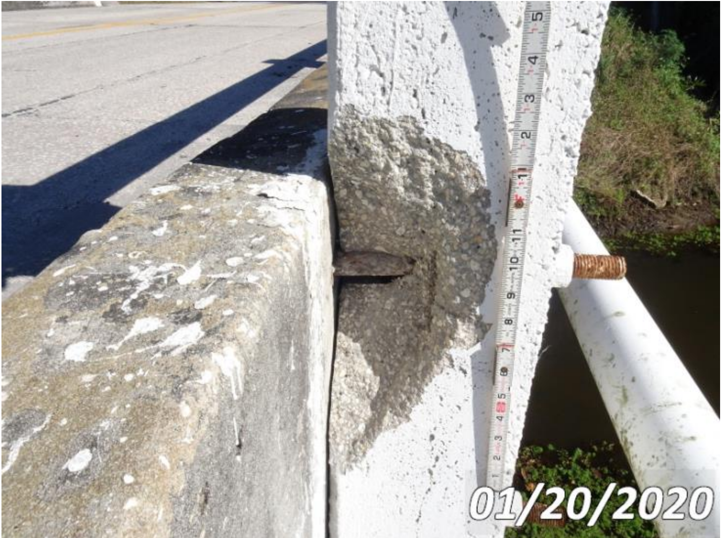
Photo 333-S03 (Unit 0: Other Bridge Railing)
