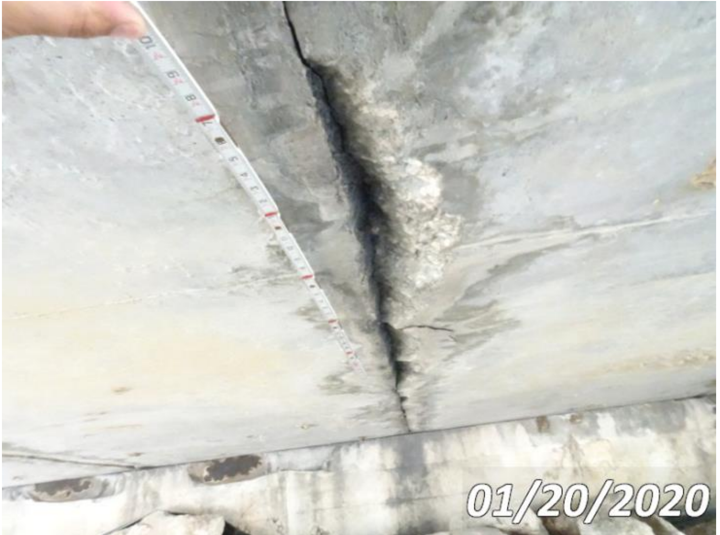
Photo 38-S04 (Unit 0: Re Concrete Slab)
