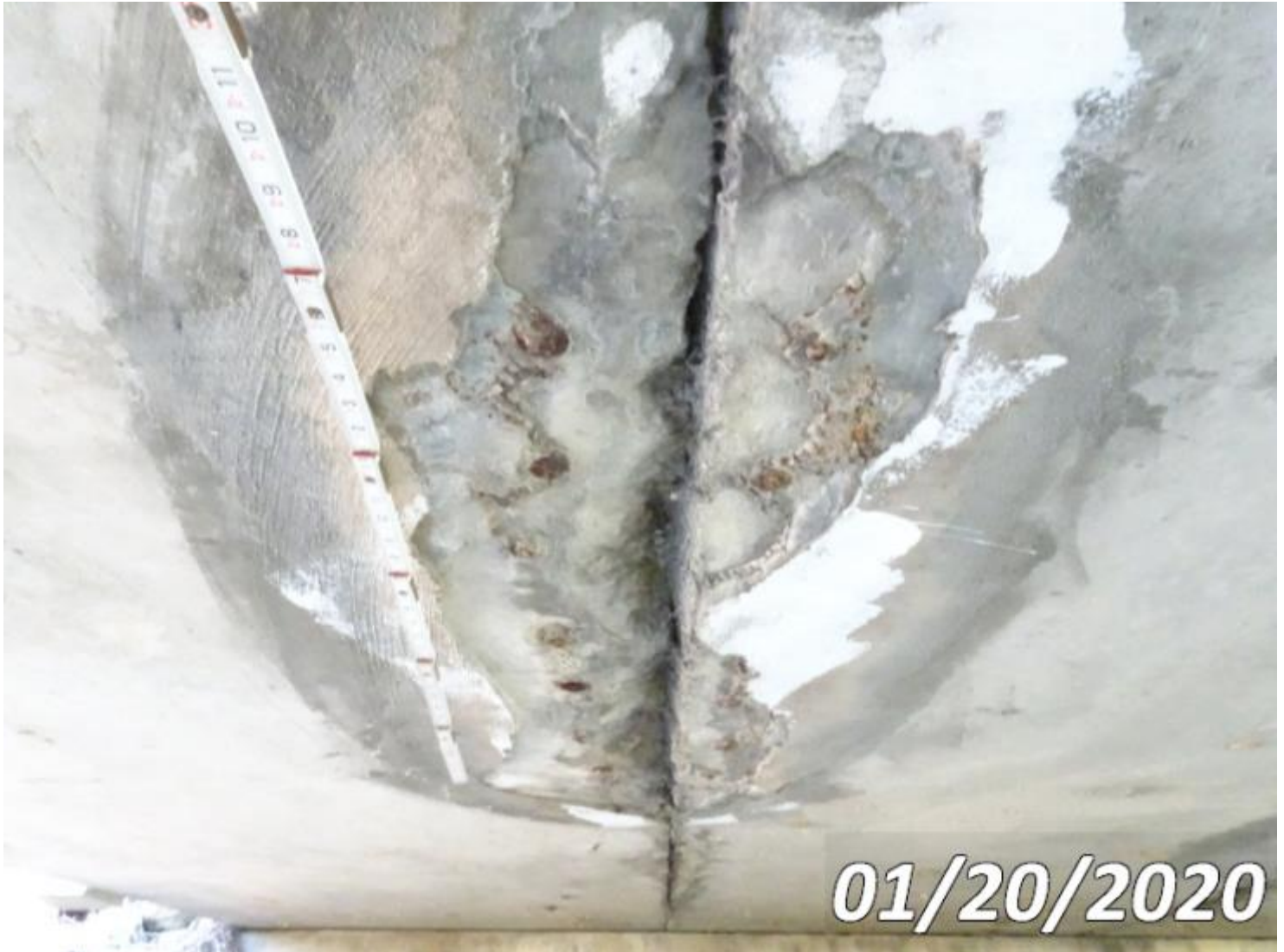
Photo 38-S06 (Unit 0: Re Concrete Slab)
