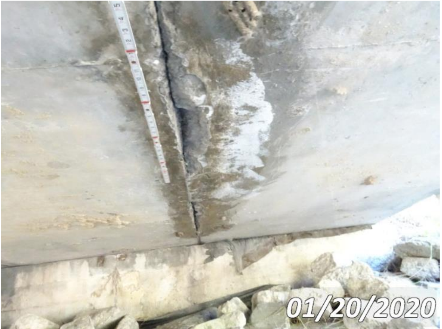
Photo 38-S03 (Unit 0: Re Concrete Slab)
