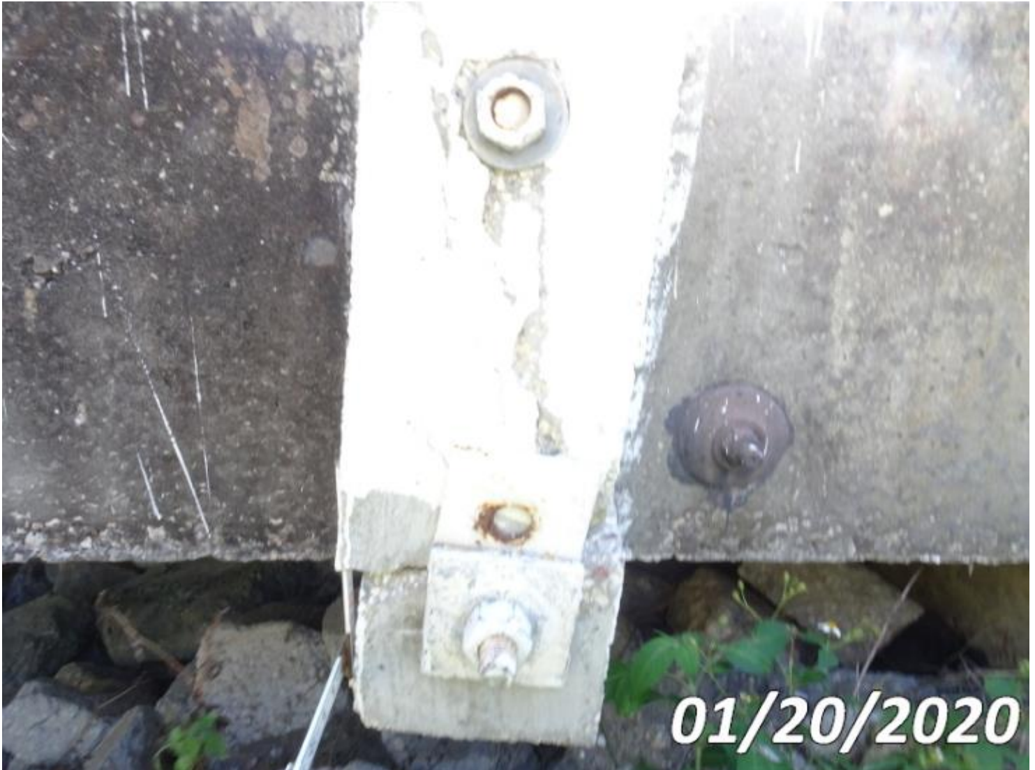
Photo 333-S01 (Unit 0: Other Bridge Railing)
