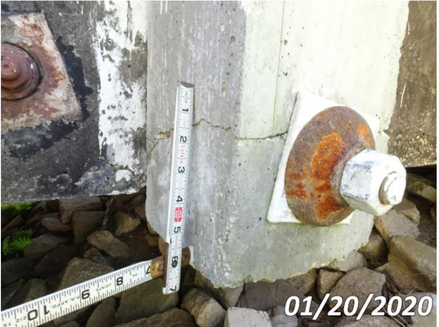
Photo 333-S02 (Unit 0: Other Bridge Railing)
