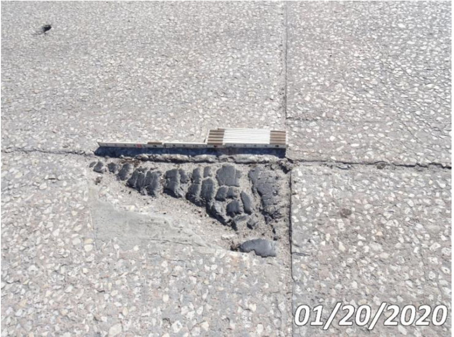
Photo 38-S01 (Unit 0: Re Concrete Slab)
