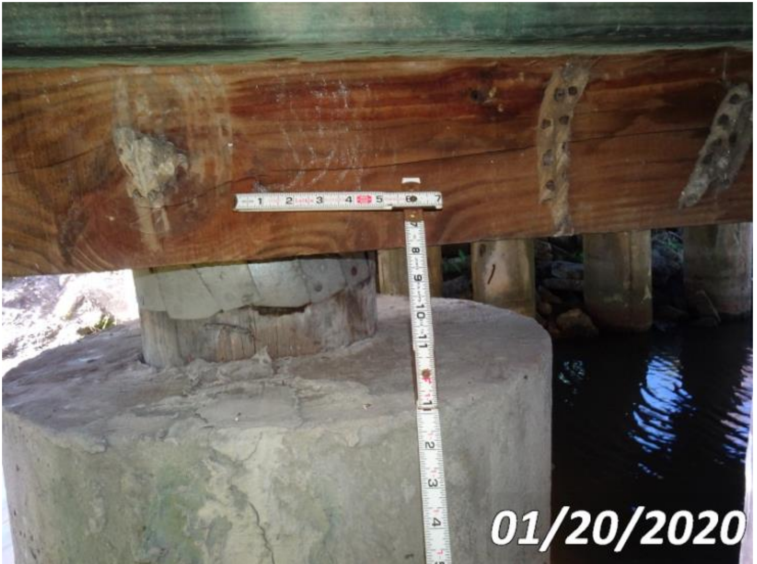
Photo 235-S01 (Unit 0: Timber Pier Cap)
