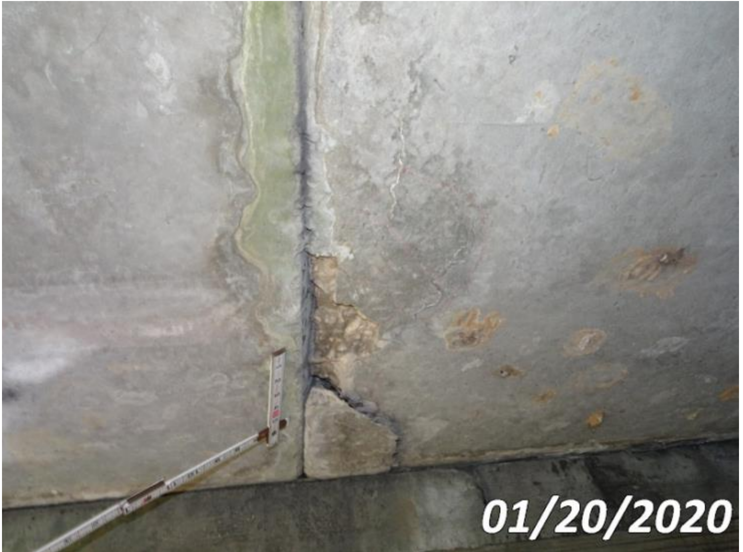
Photo 38-S08 (Unit 0: Re Concrete Slab)
