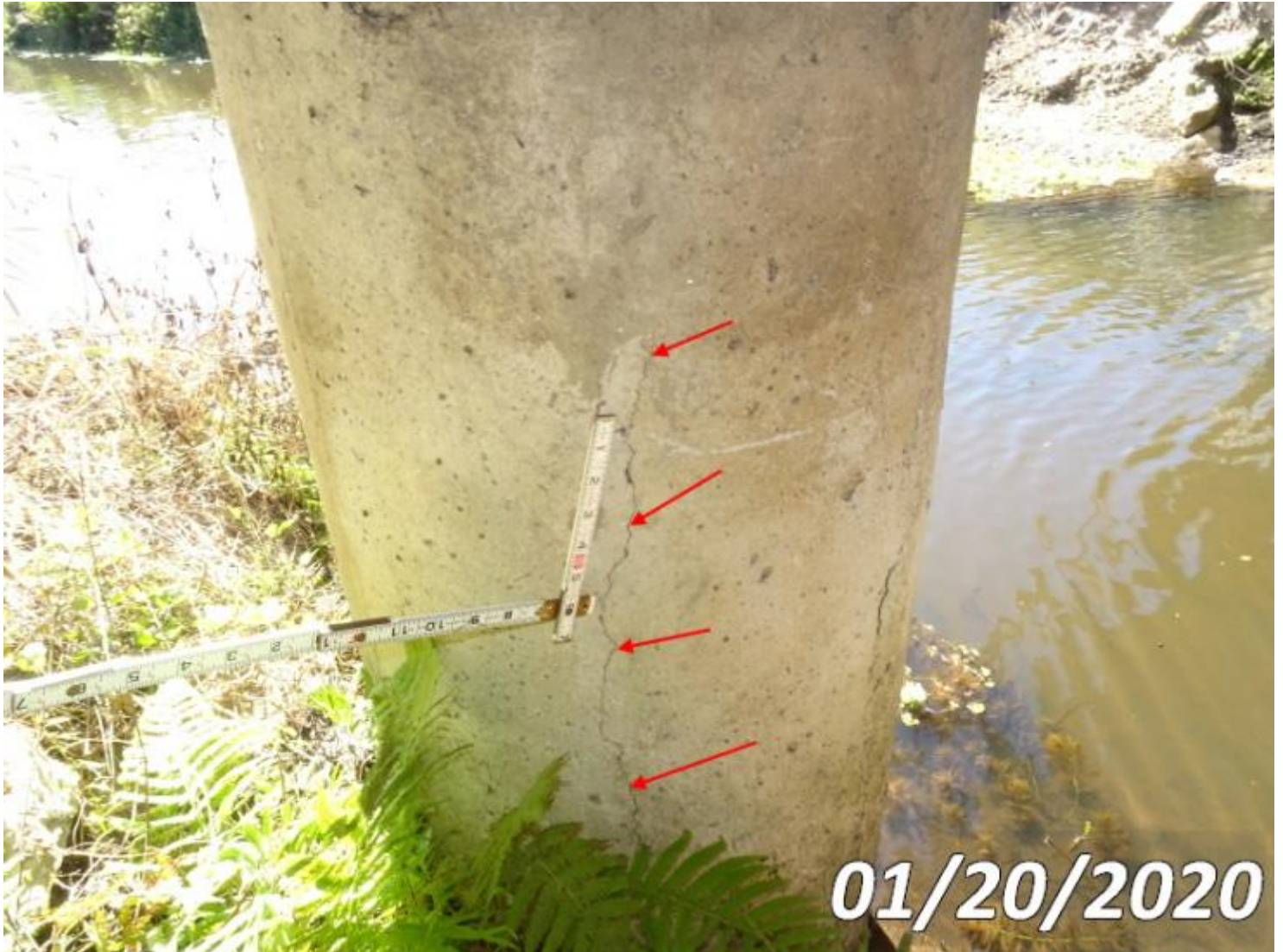
Photo 8298-S01 (Unit 0: Pile Jacket Bare)
