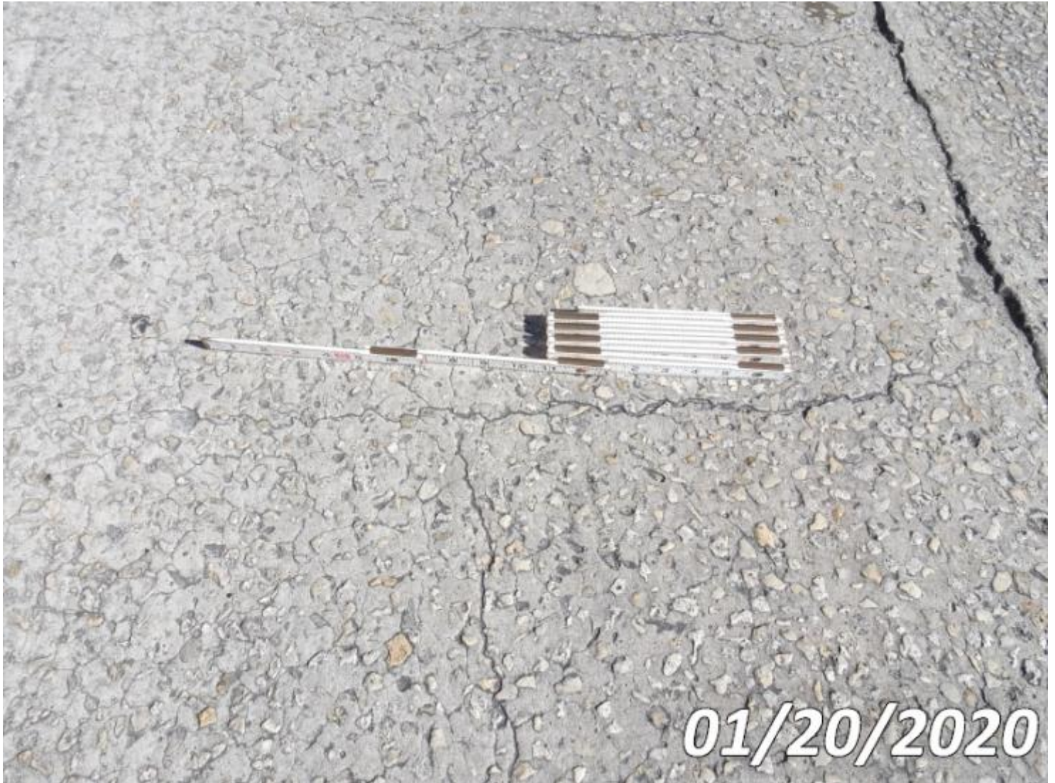
Photo 38-S02 (Unit 0: Re Concrete Slab)
