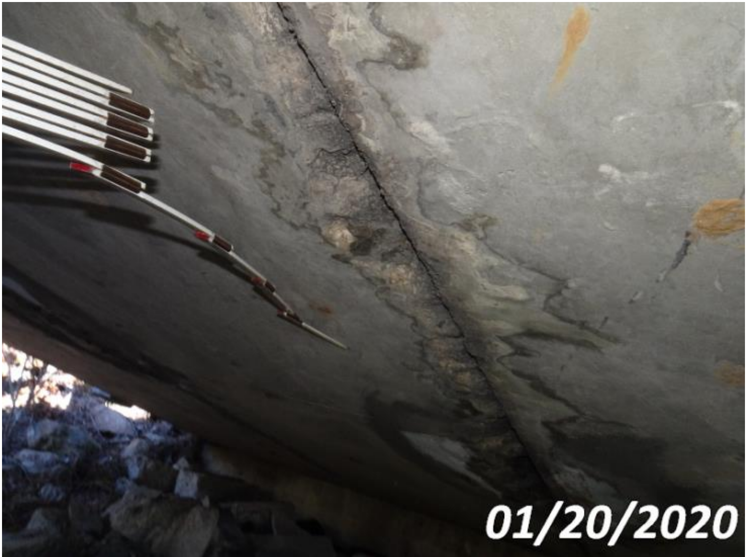
Photo 38-S07 (Unit 0: Re Concrete Slab)
