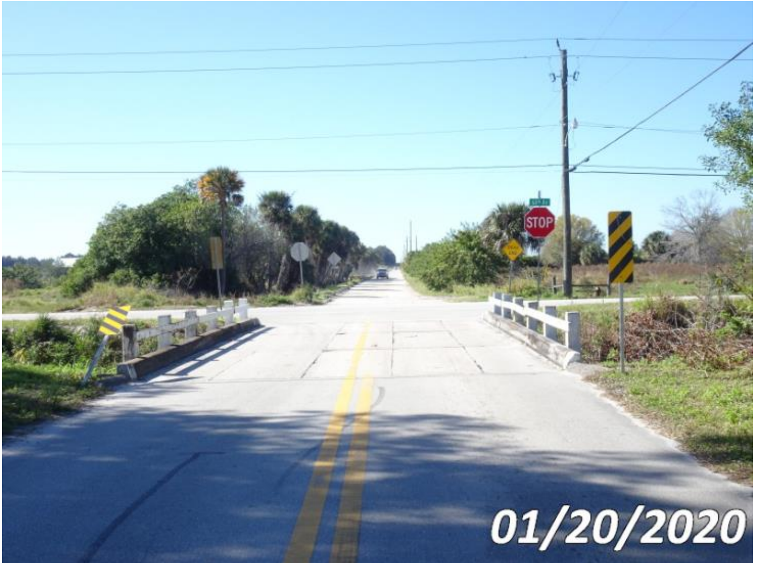
EAST APPROACH LOOKING WEST
