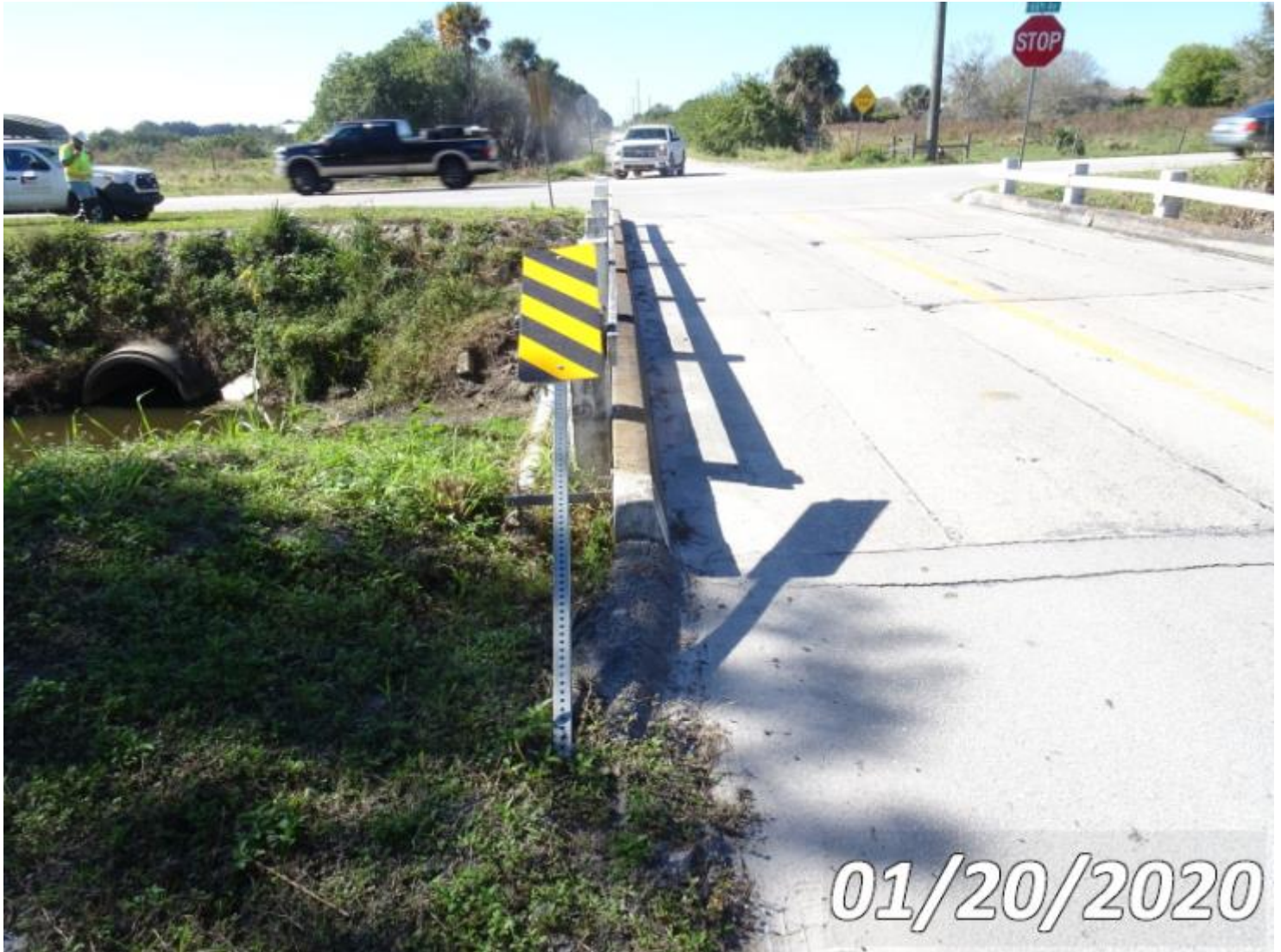
Photo 333-S05 (Unit 0: Other Bridge Railing)
