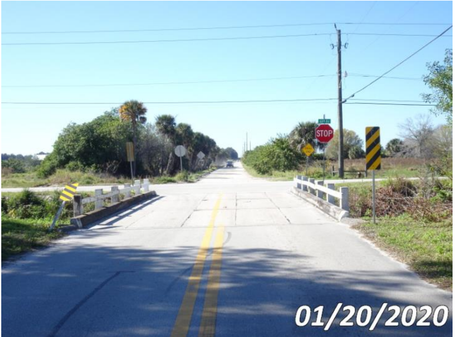
Photo 333-S04 (Unit 0: Other Bridge Railing)
