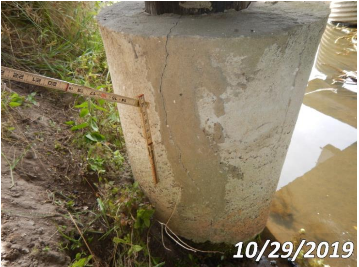
Photo 8298-S03 (Unit 0: Pile Jacket Bare)
