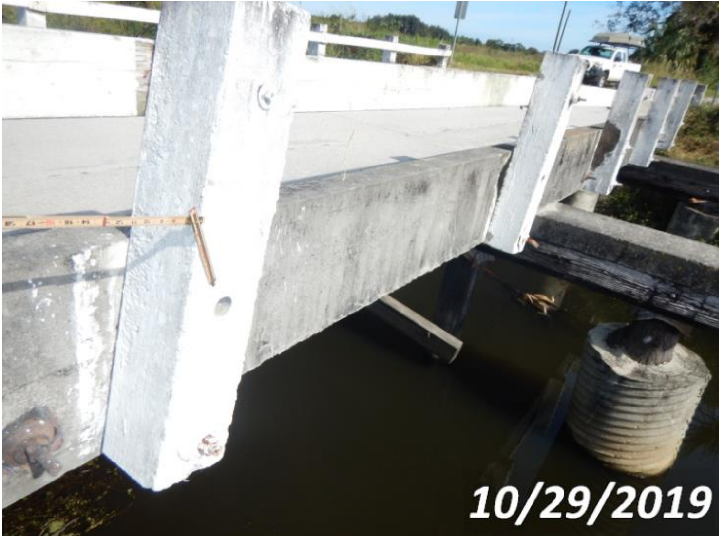
Photo 333-S04 (Unit 0: Other Bridge Railing)
