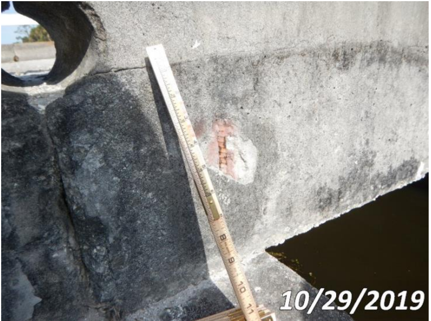
Photo 38-S02 (Unit 0: Re Concrete Slab)
