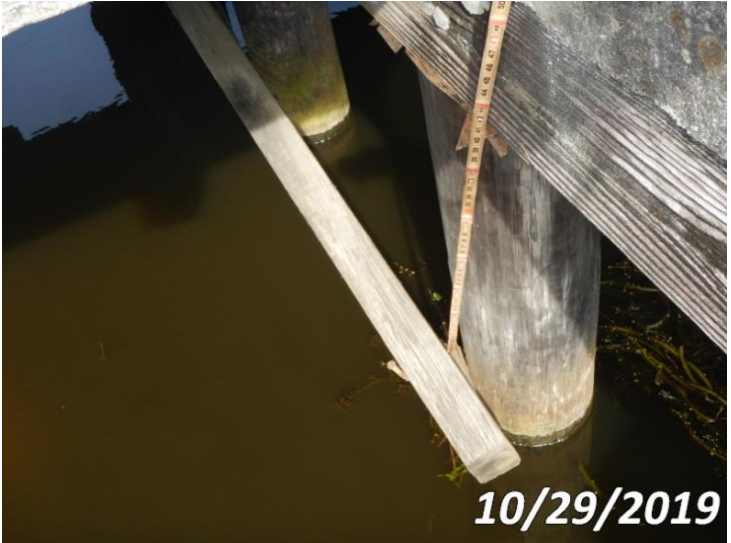
Photo 228-S03 (Unit 0: Timber Pile)
