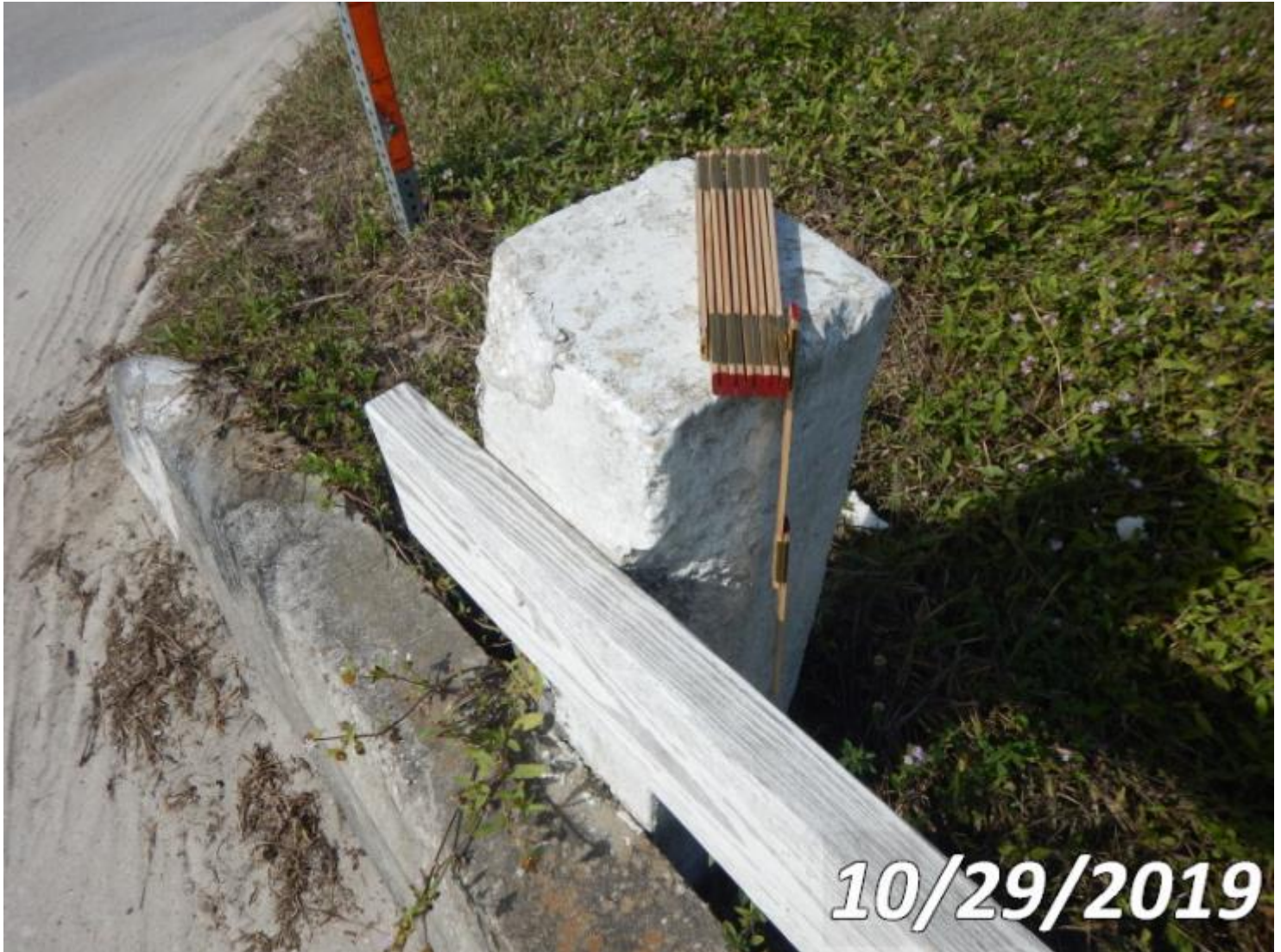
Photo 333-S01 (Unit 0: Other Bridge Railing)
