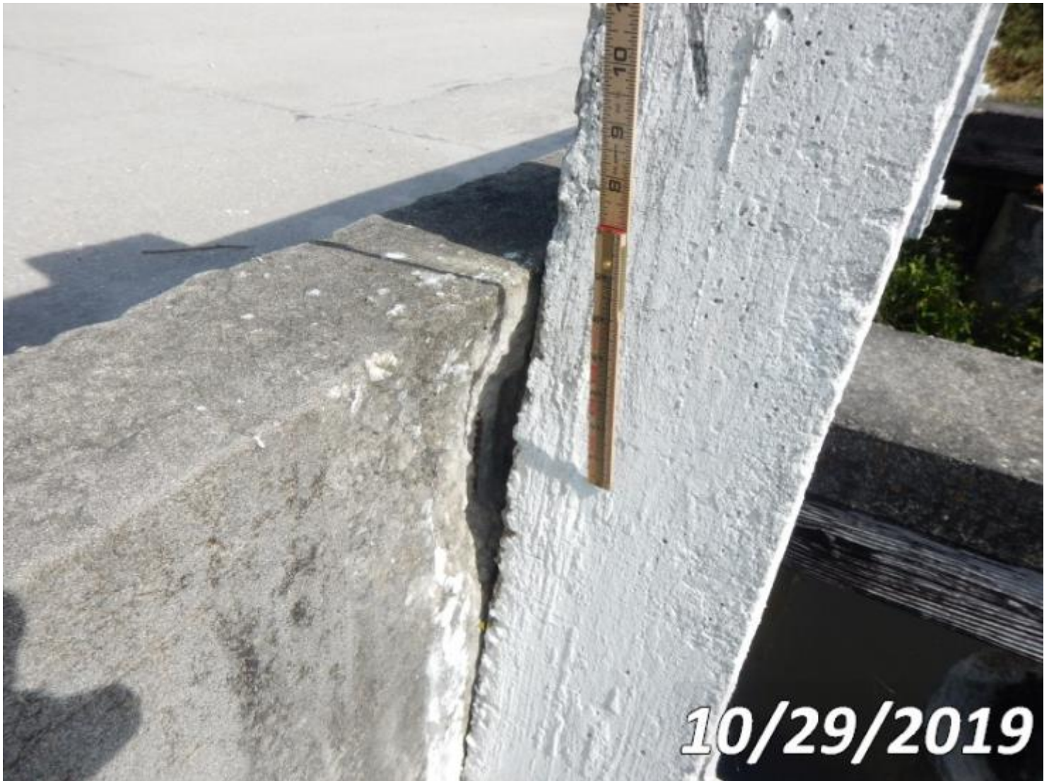
Photo 38-S03 (Unit 0: Re Concrete Slab)
