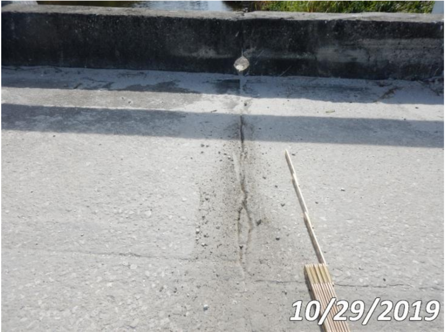
Photo 301-S01 (Unit 0: Pourable Joint Seal)
