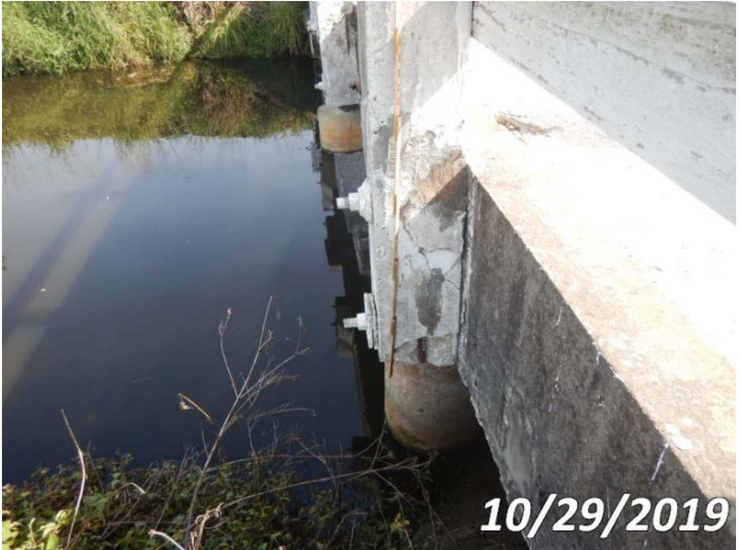
Photo 333-S03 (Unit 0: Other Bridge Railing)
