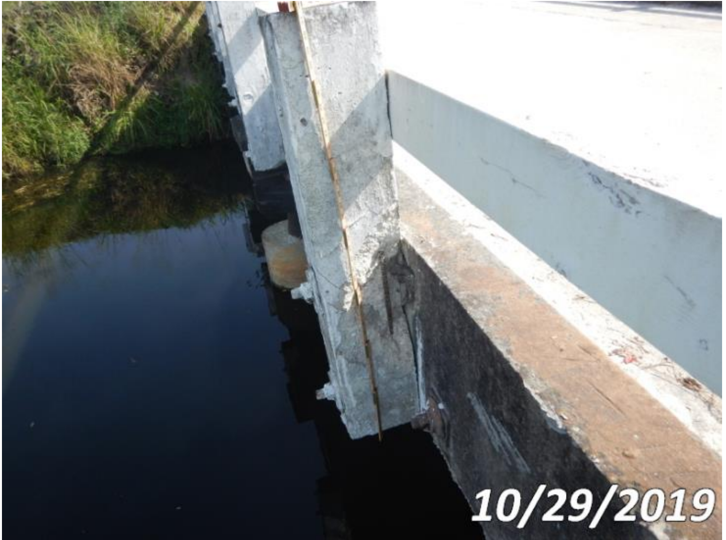
Photo 333-S05 (Unit 0: Other Bridge Railing)
