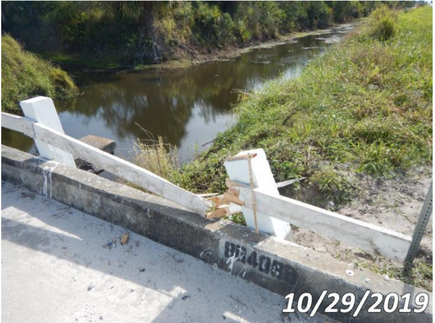
Photo 333-S02 (Unit 0: Other Bridge Railing)
