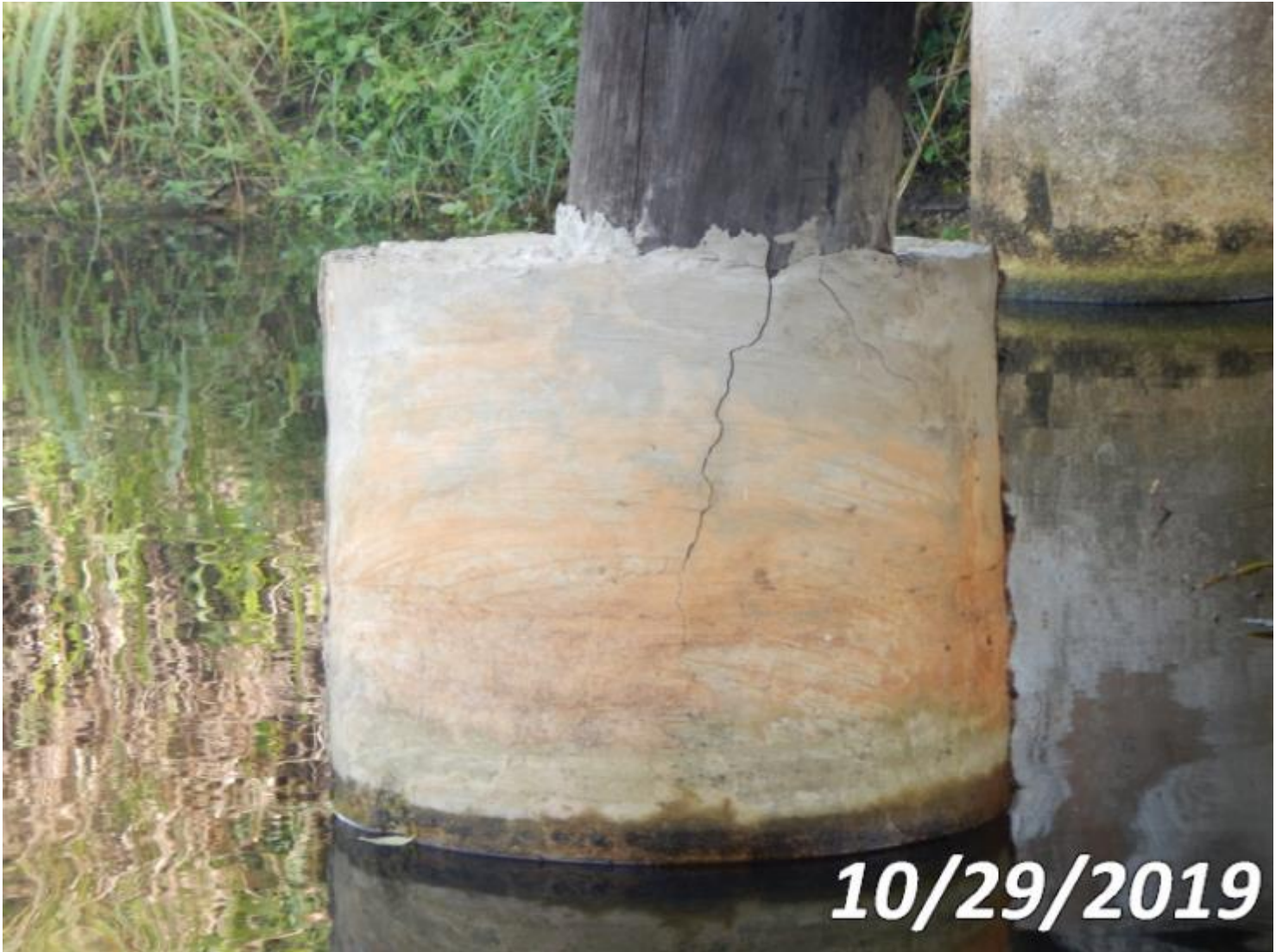
Photo 8298-S02 (Unit 0: Pile Jacket Bare)
