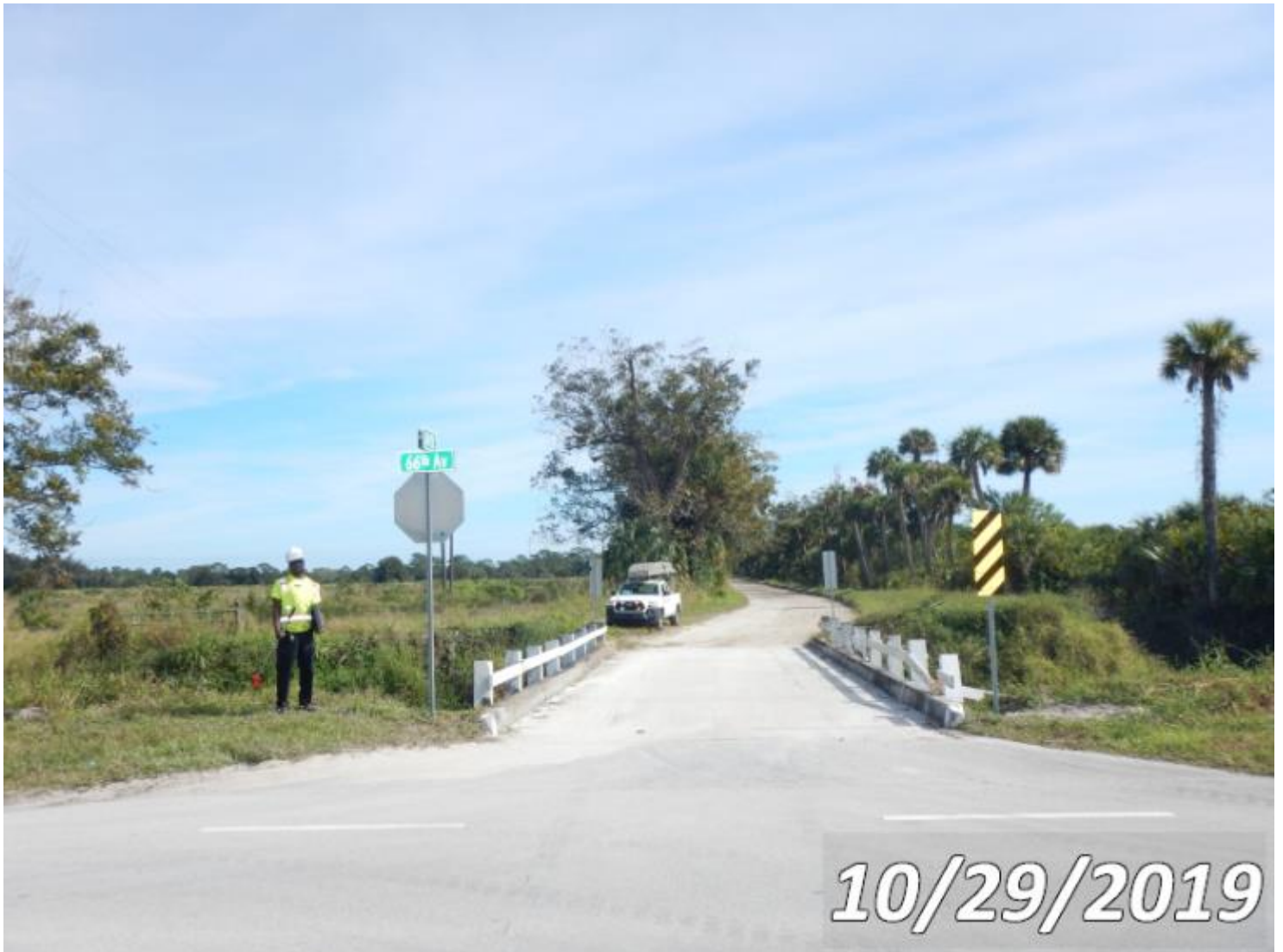
WEST APPROACH LOOKING EAST
