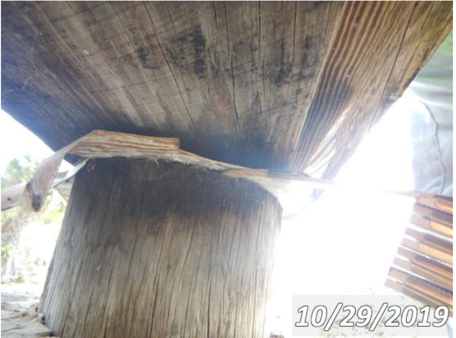
Photo 228-S02 (Unit 0: Timber Pile)
