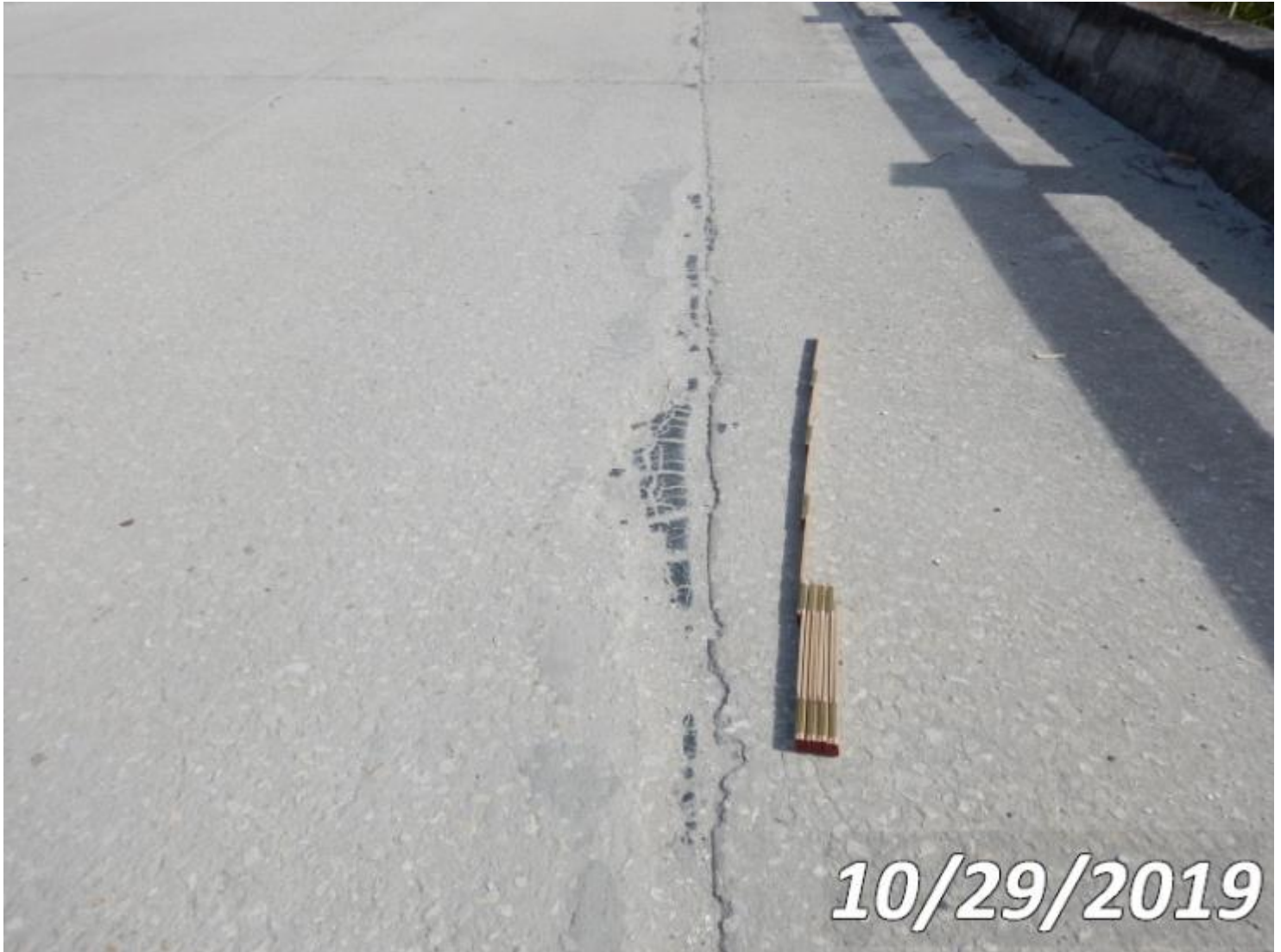
Photo 38-S01 (Unit 0: Re Concrete Slab)
