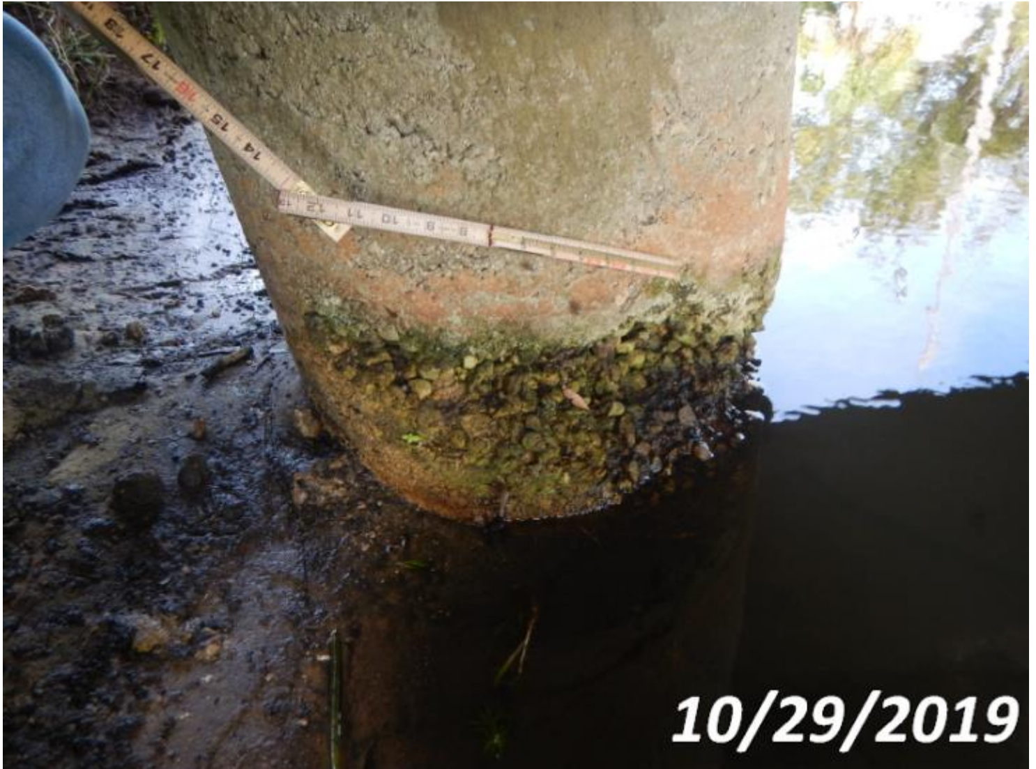
Photo 8298-S01 (Unit 0: Pile Jacket Bare)
