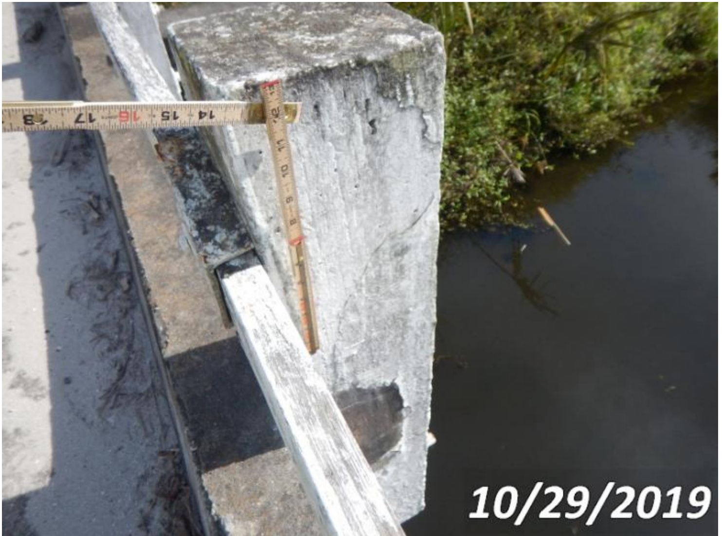
Photo 333-S06 (Unit 0: Other Bridge Railing)
