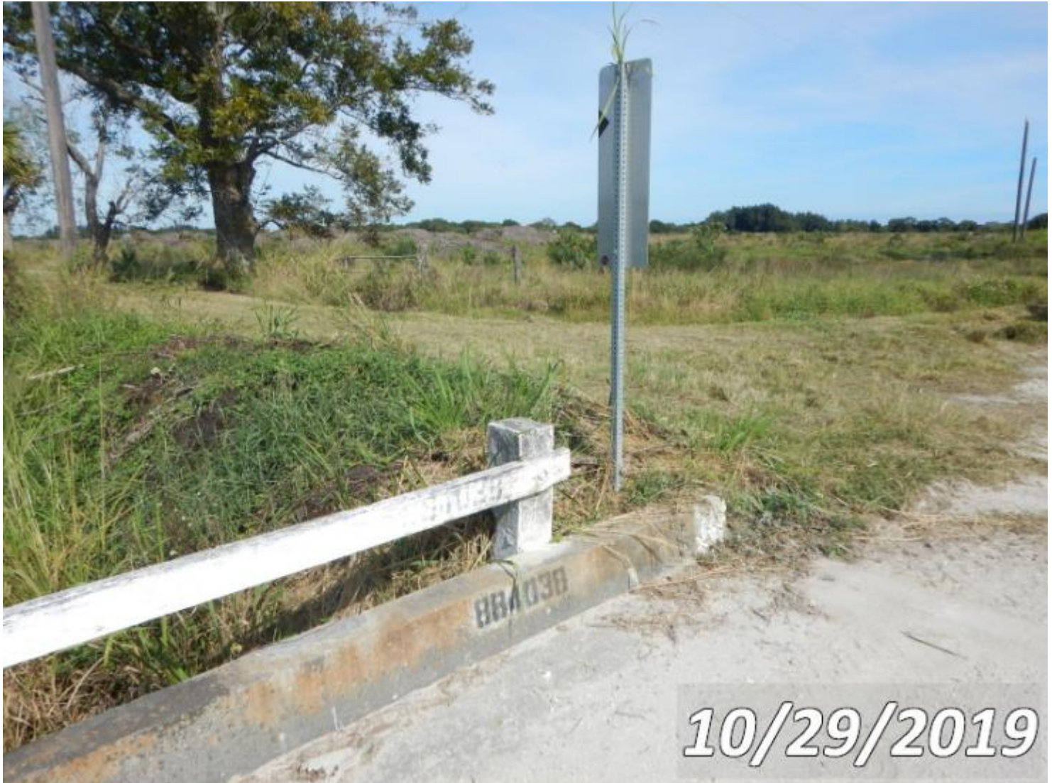
Photo 333-S07 (Unit 0: Other Bridge Railing)
