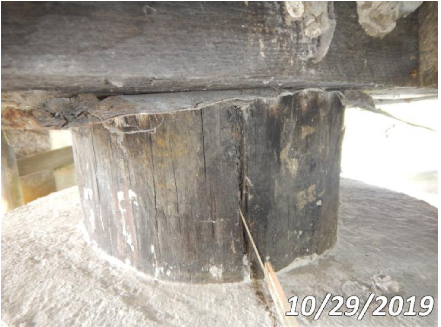
Photo 228-S01 (Unit 0: Timber Pile)
