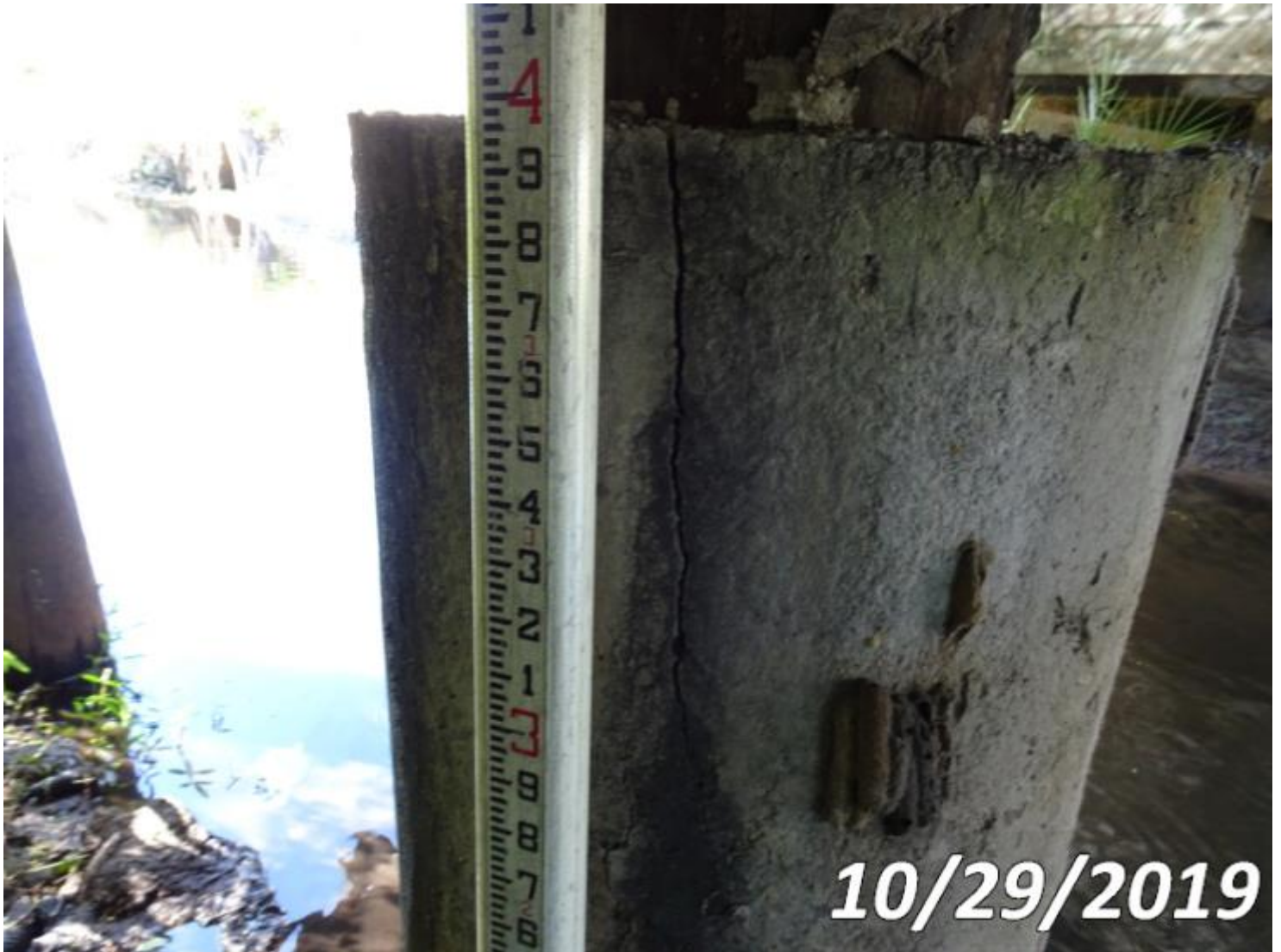
Photo 8298-S02 (Unit 0: Pile Jacket Bare)
