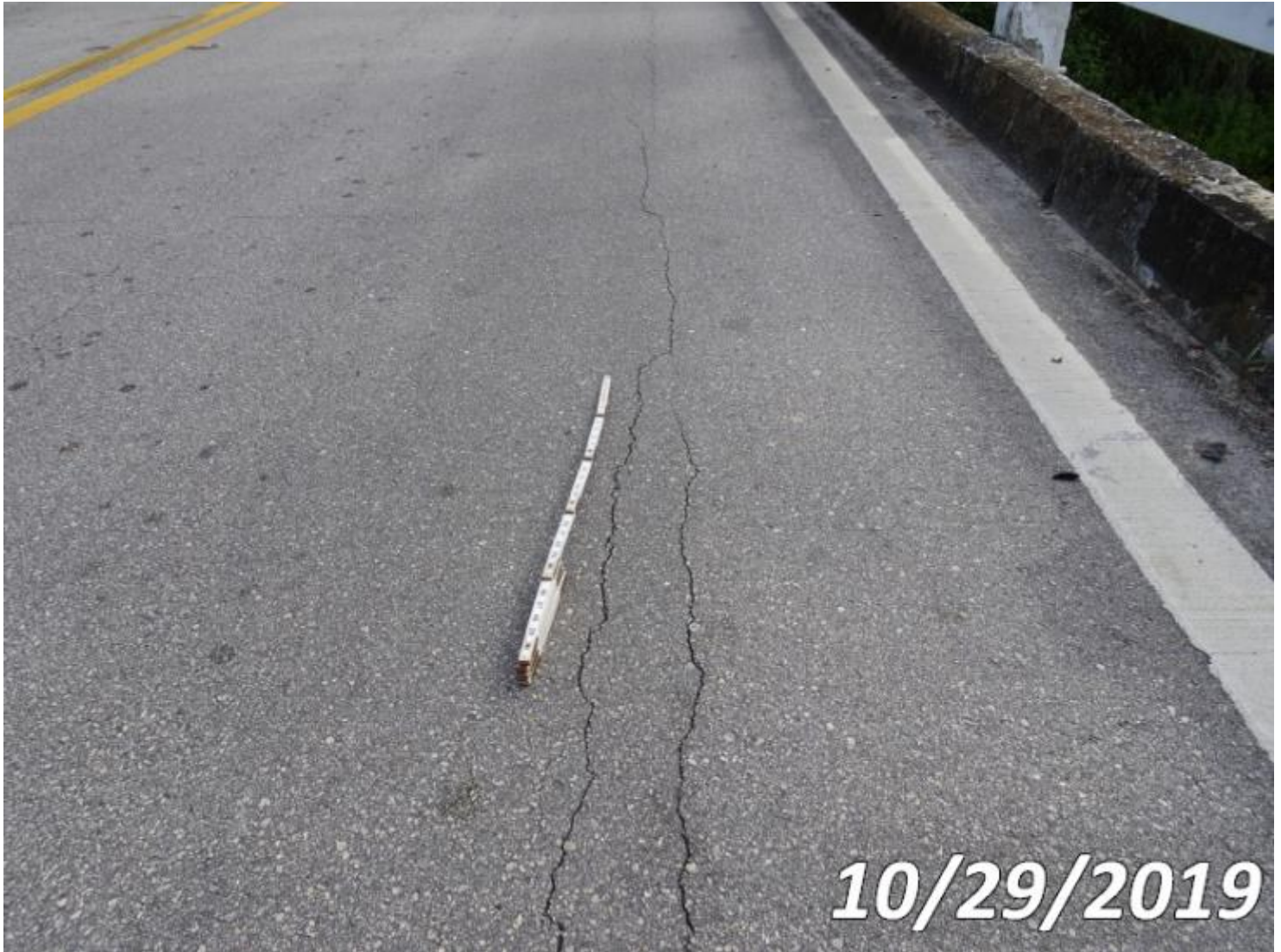
Photo 38-S07 (Unit 0: Re Concrete Slab)
