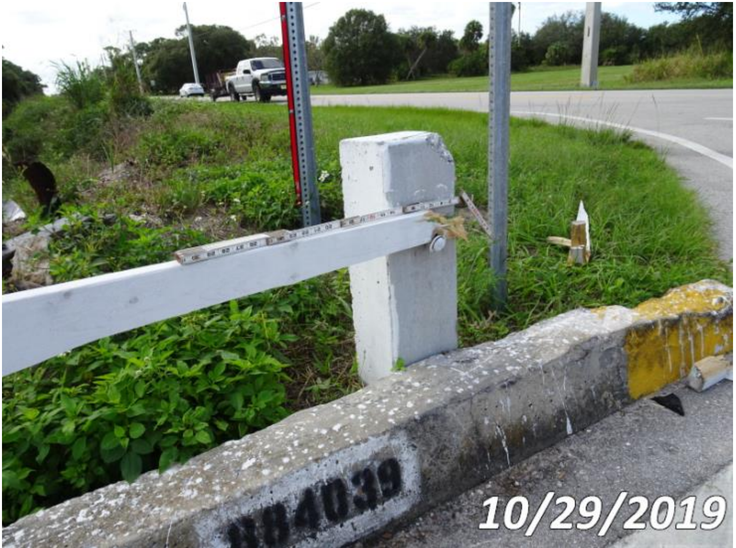
Photo 333-S02 (Unit 0: Other Bridge Railing)
