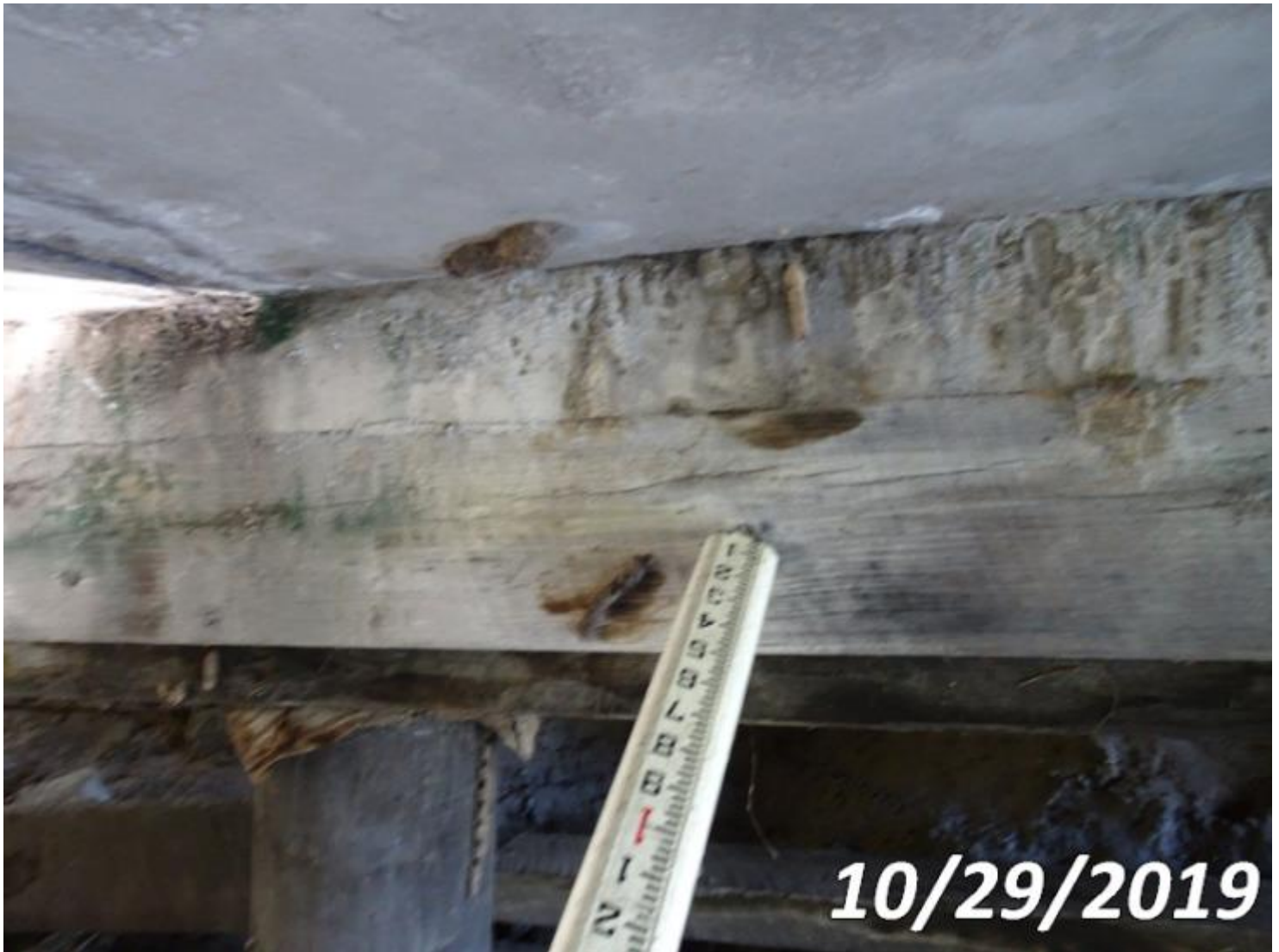
Photo 235-S01 (Unit 0: Timber Pier Cap)
