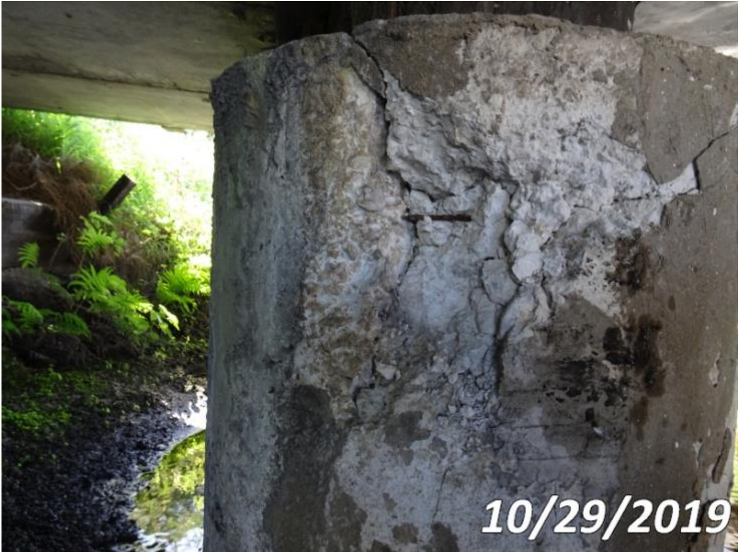
Photo 8298-S01 (Unit 0: Pile Jacket Bare)
