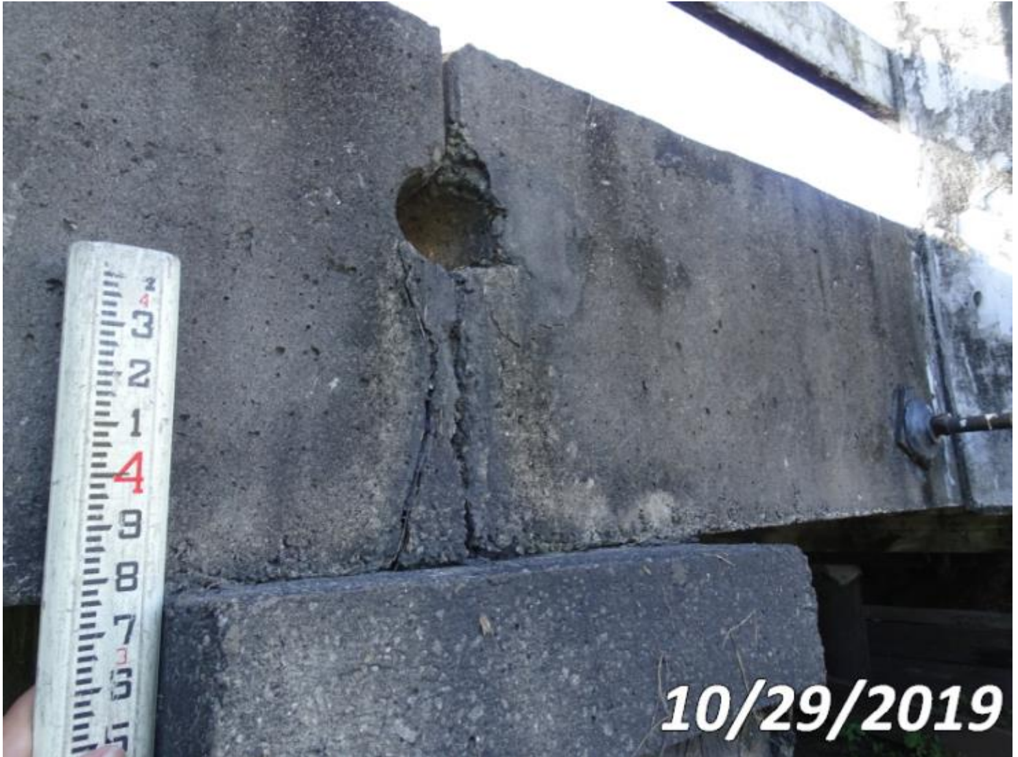
Photo 38-S06 (Unit 0: Re Concrete Slab)
