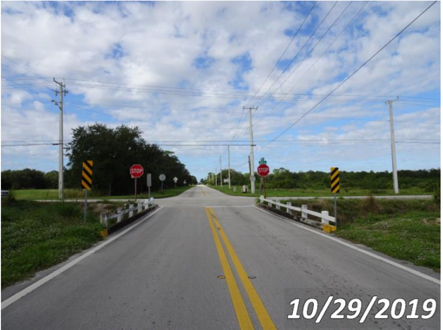
Photo 333-S03 (Unit 0: Other Bridge Railing)
