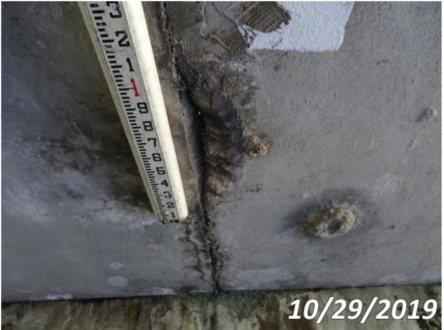
Photo 38-S02 (Unit 0: Re Concrete Slab)
