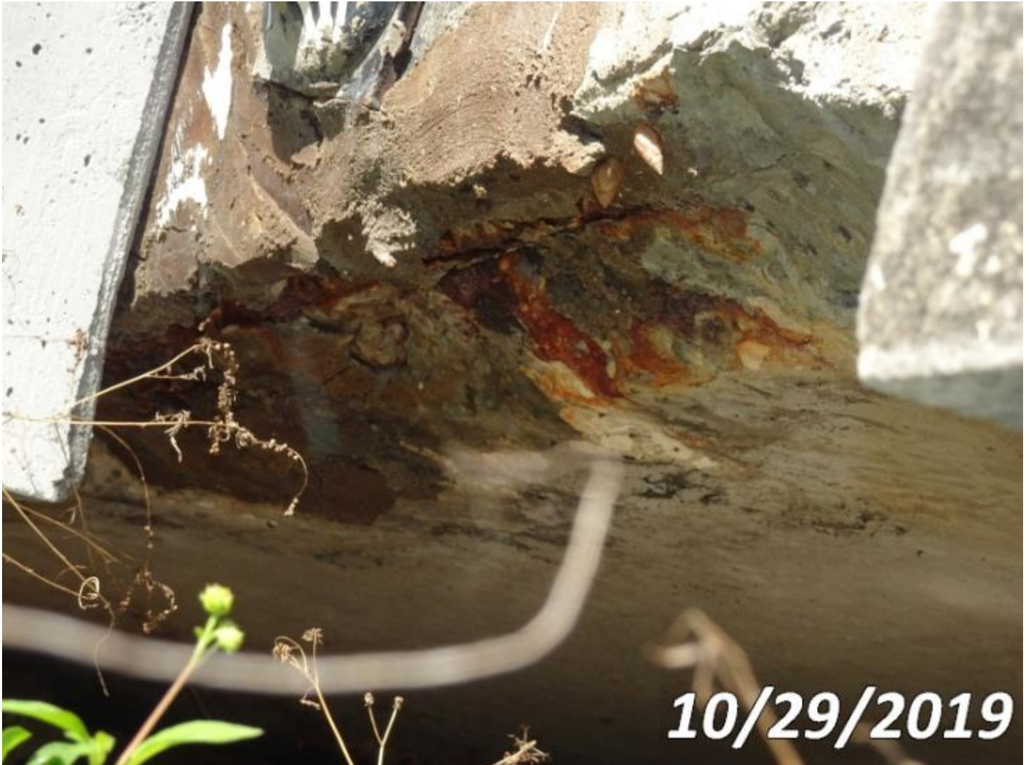
Photo 38-S01 (Unit 0: Re Concrete Slab)
