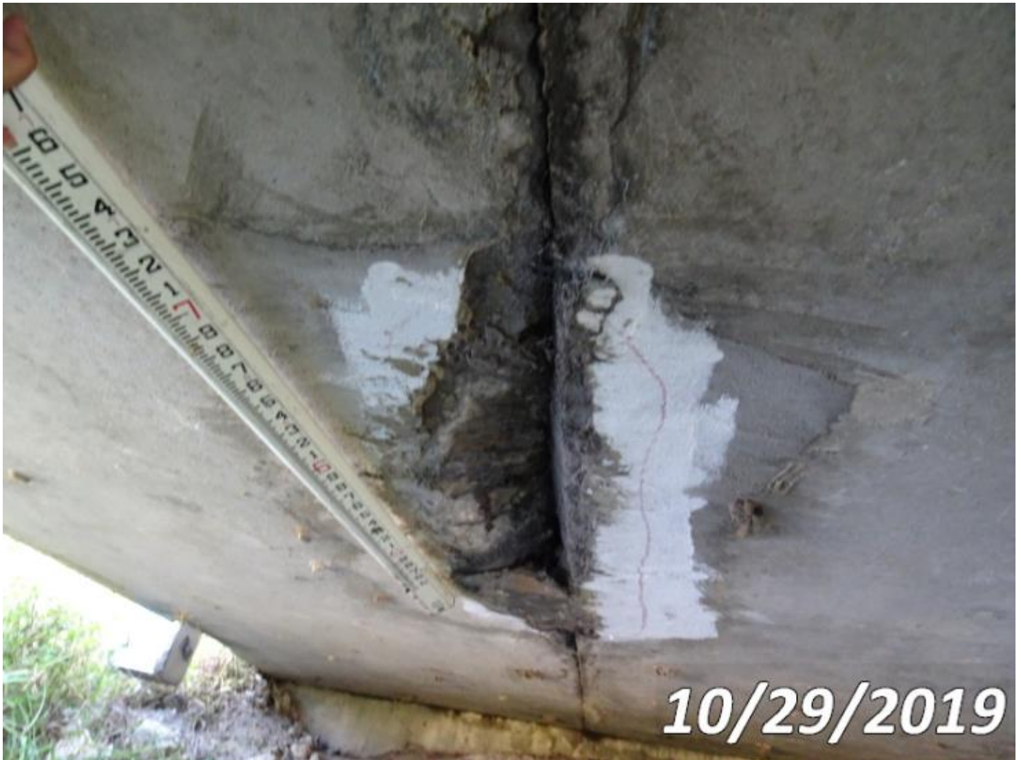
Photo 38-S04 (Unit 0: Re Concrete Slab)
