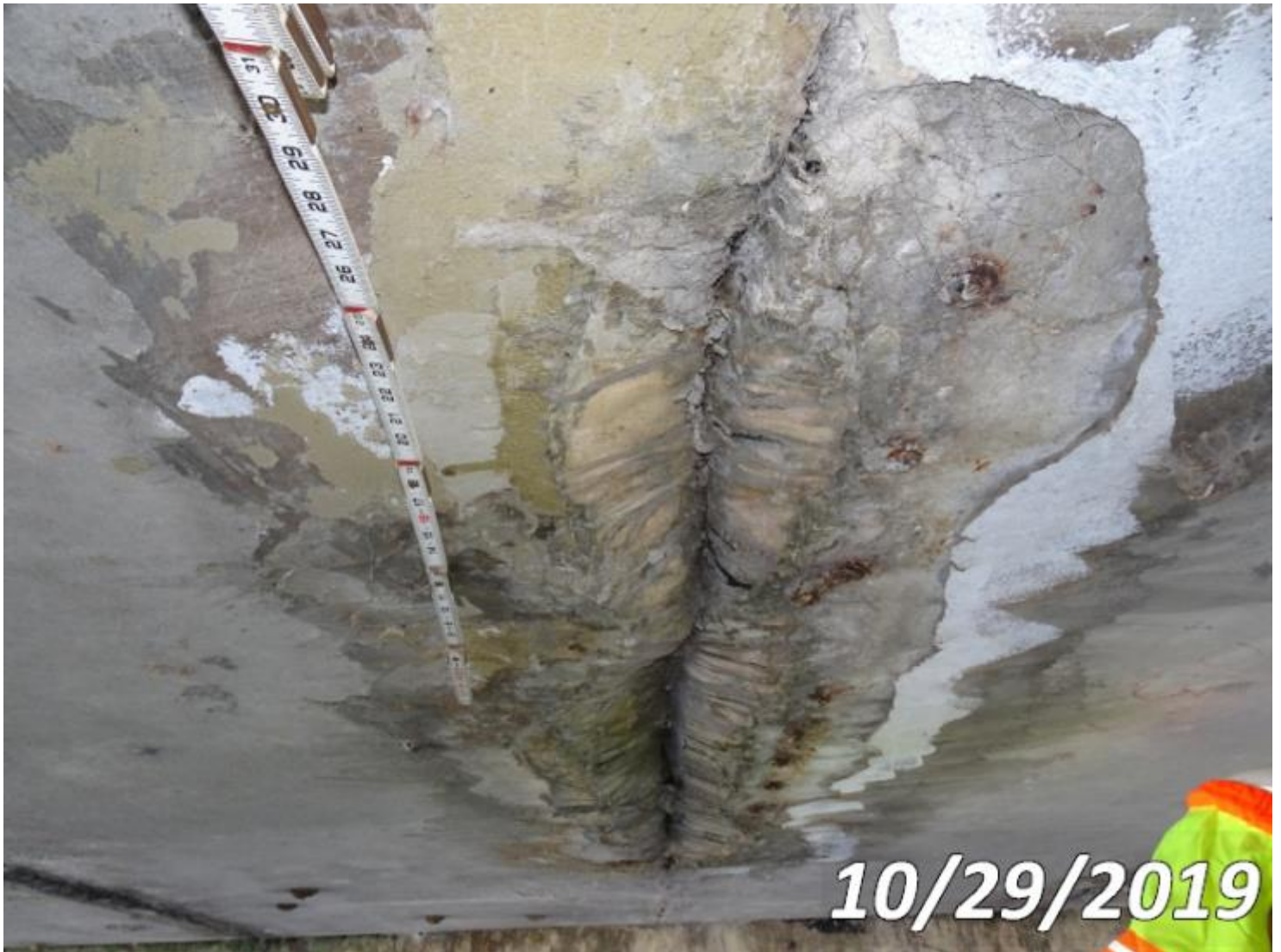
Photo 38-S05 (Unit 0: Re Concrete Slab)
