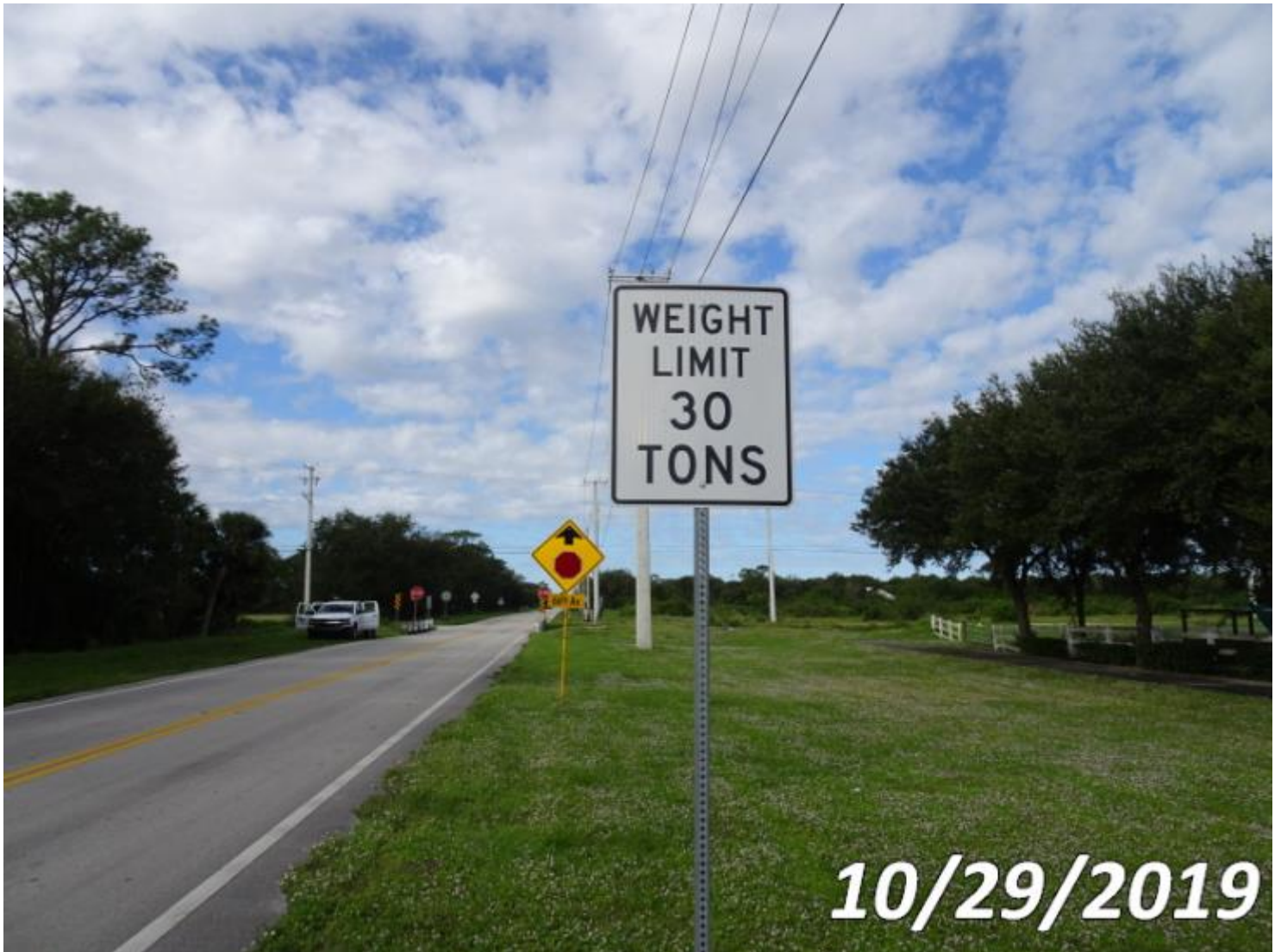
WEIGHT LIMIT SIGN AT THE EAST APPROACH
