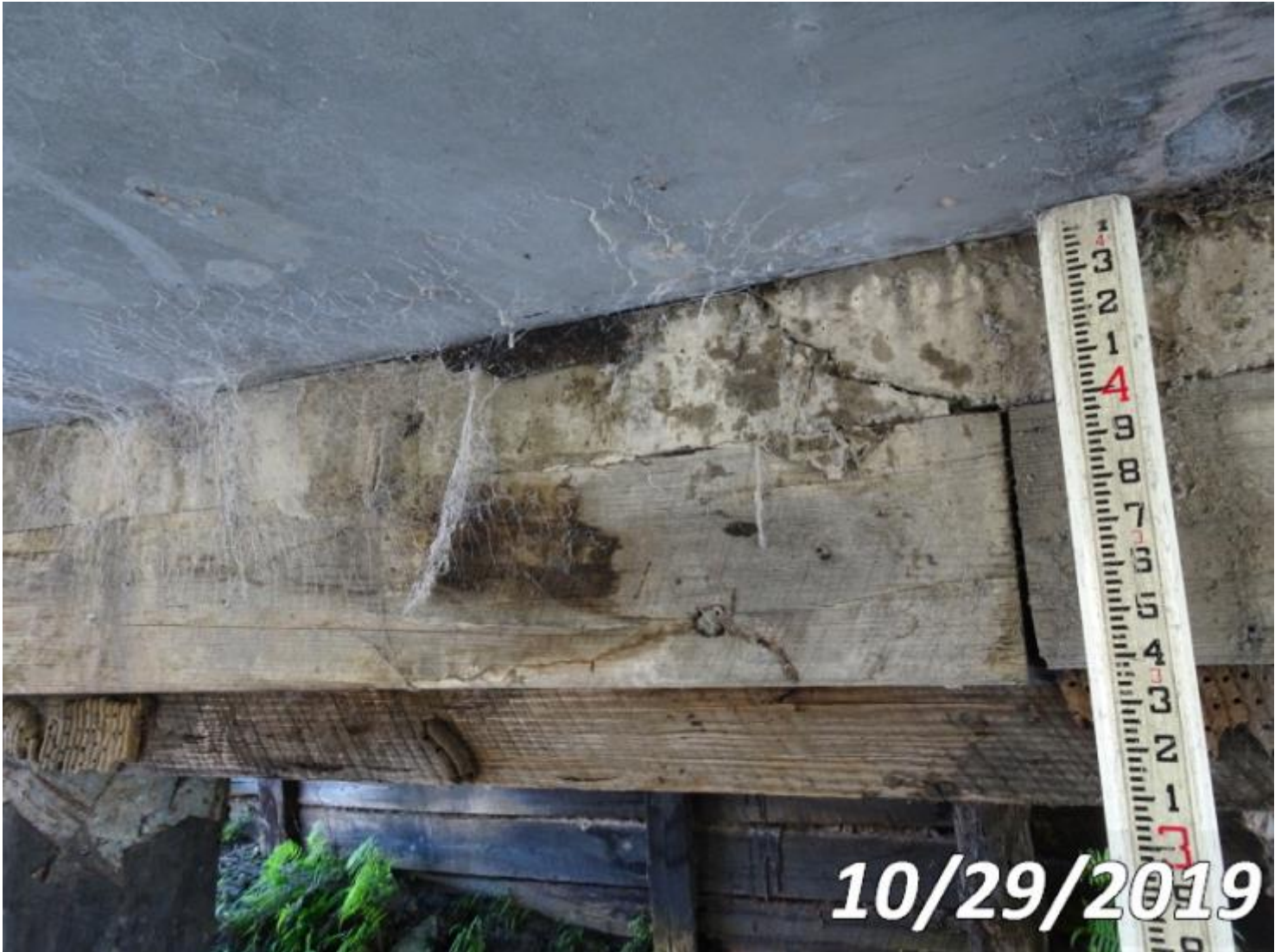
Photo 234-S01 (Unit 0: Re Conc Pier Cap)
