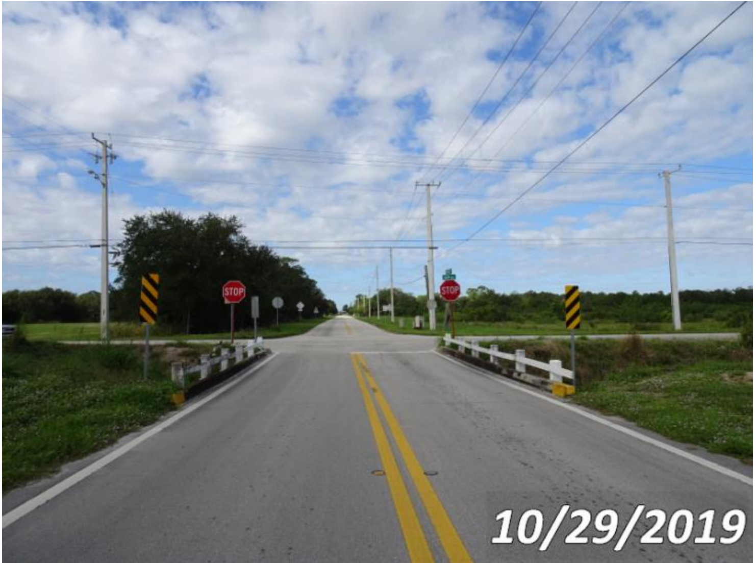
EAST APPROACH LOOKING WEST
