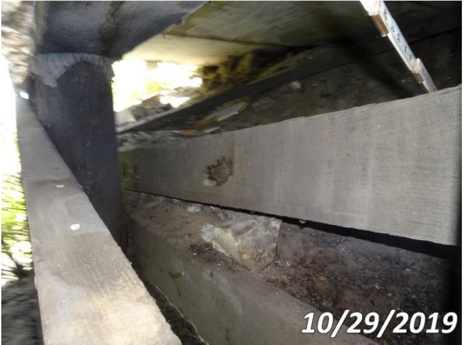
Photo 8476-S02 (Unit 0: Timber Walls)
