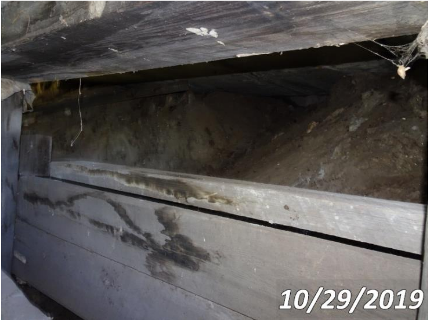
Photo 8476-S01 (Unit 0: Timber Walls)
