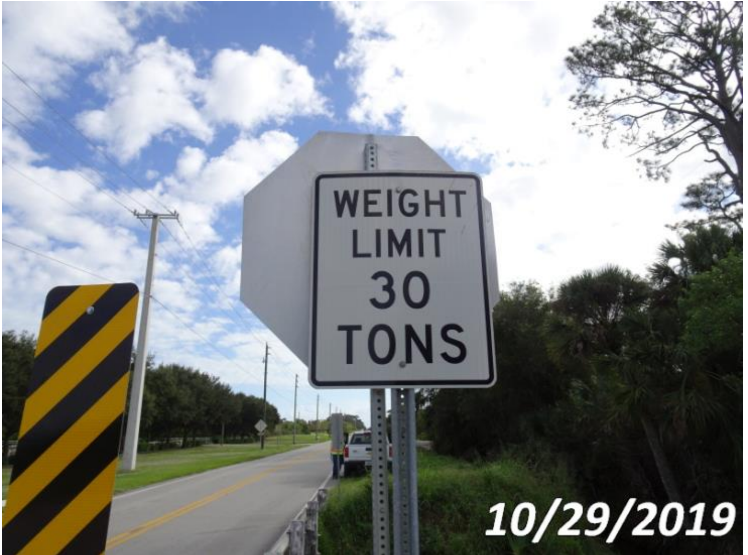
WEIGHT LIMIT SIGN AT THE WEST APPROACH
