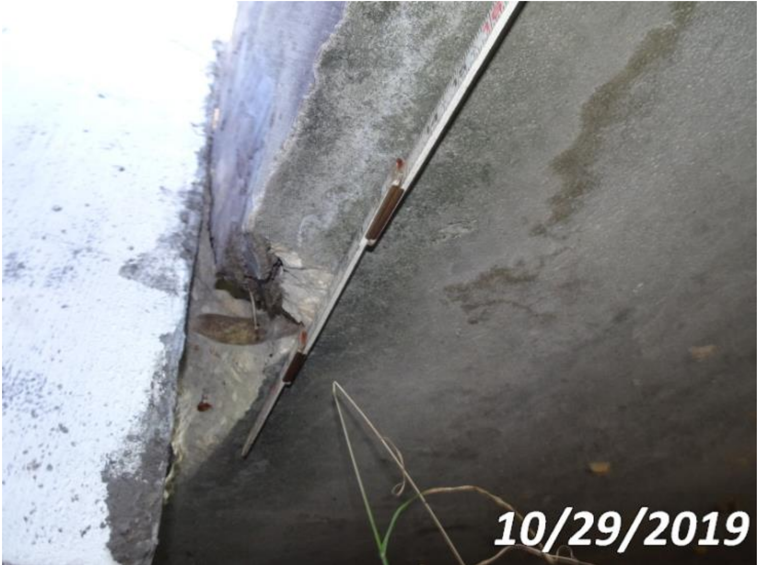
Photo 38-S03 (Unit 0: Re Concrete Slab)
