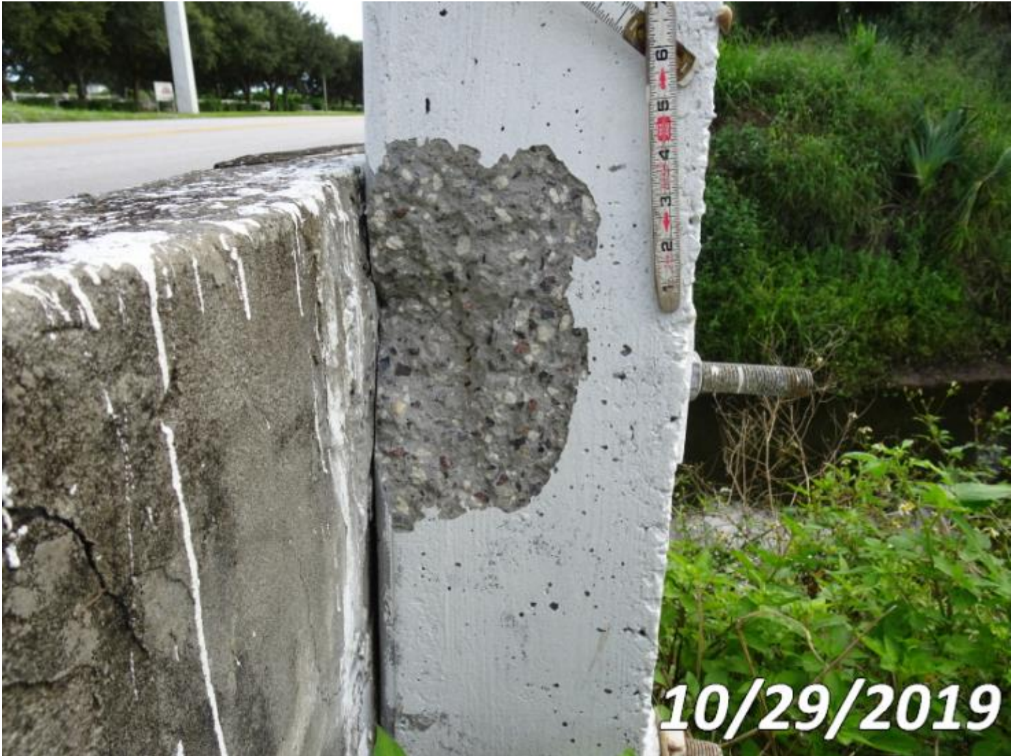
Photo 333-S01 (Unit 0: Other Bridge Railing)
