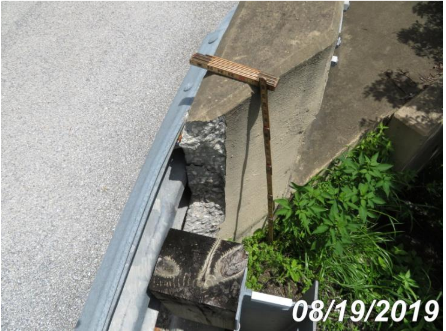
Photo 321-S01 (Unit 0: Re Conc Approach Slab)
