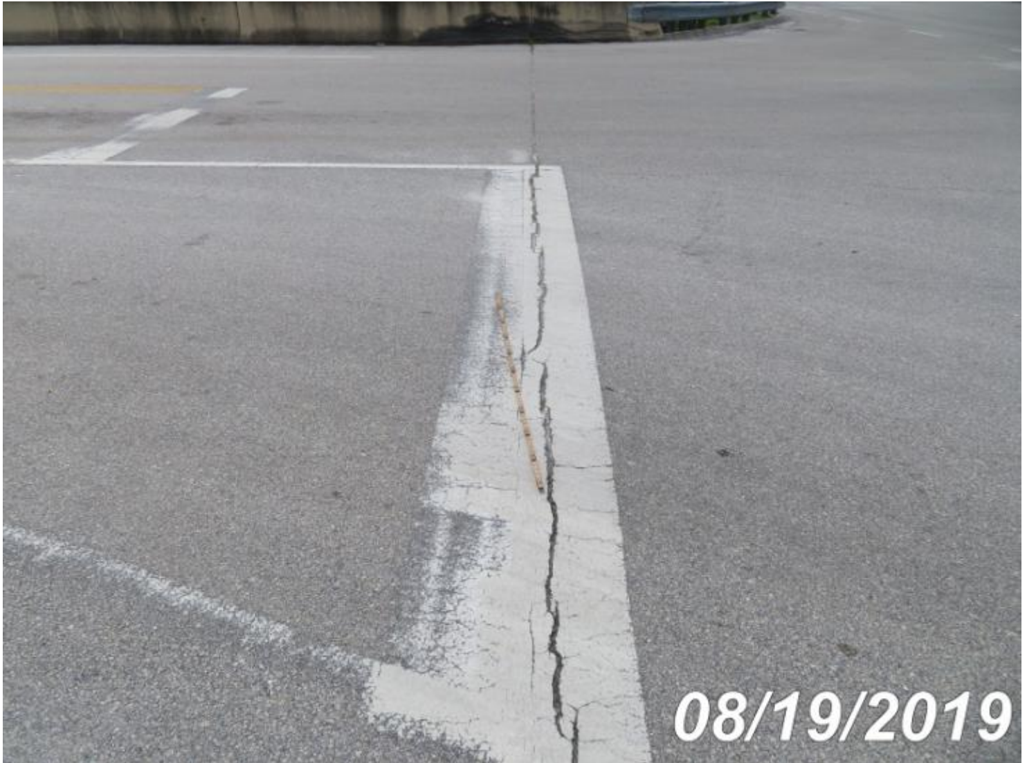
Photo 8099-S01 (Unit 0: PS Conc Slab (Sonovoid))
