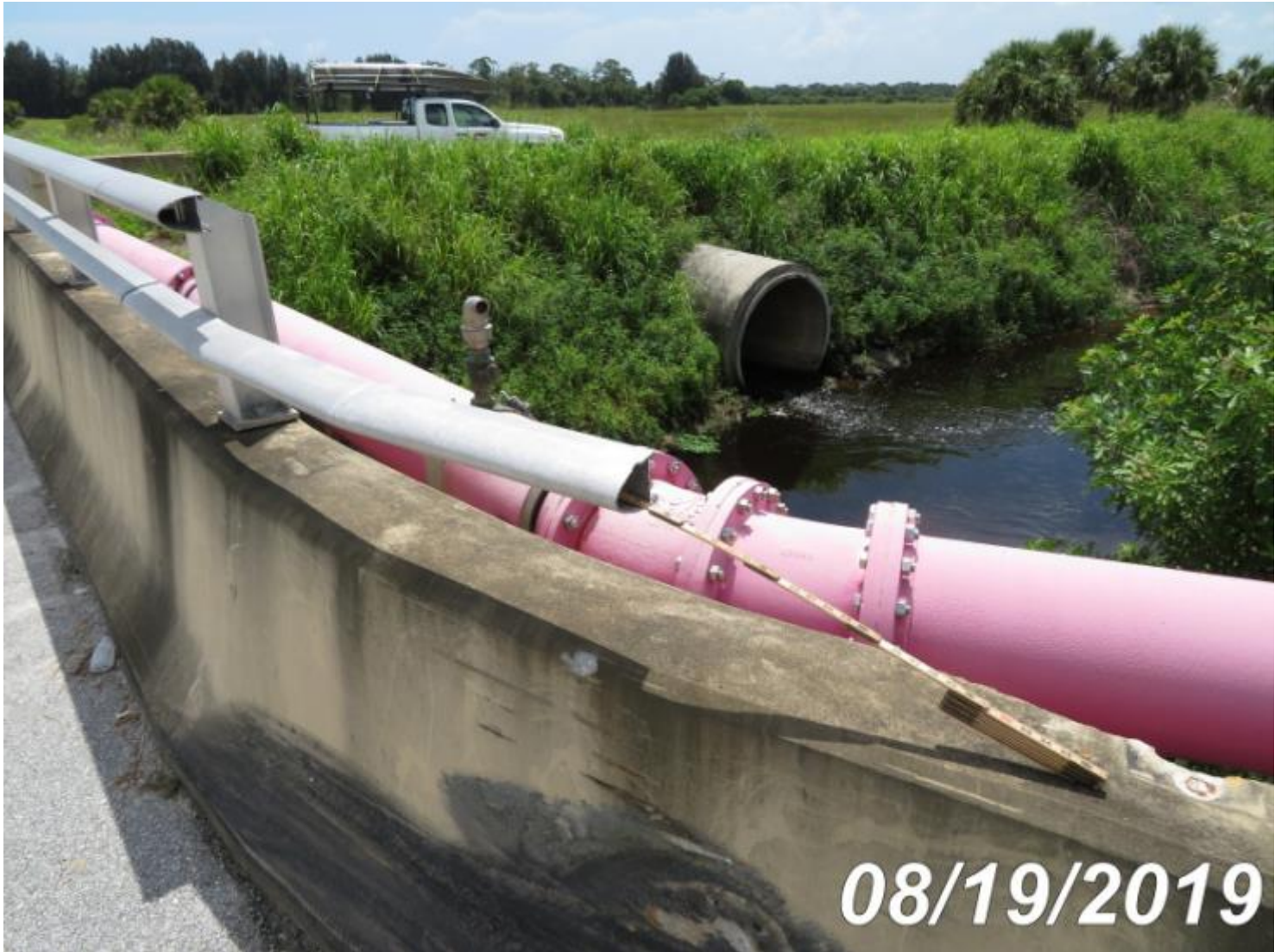
Photo 333-S01 (Unit 0: Other Bridge Railing)
