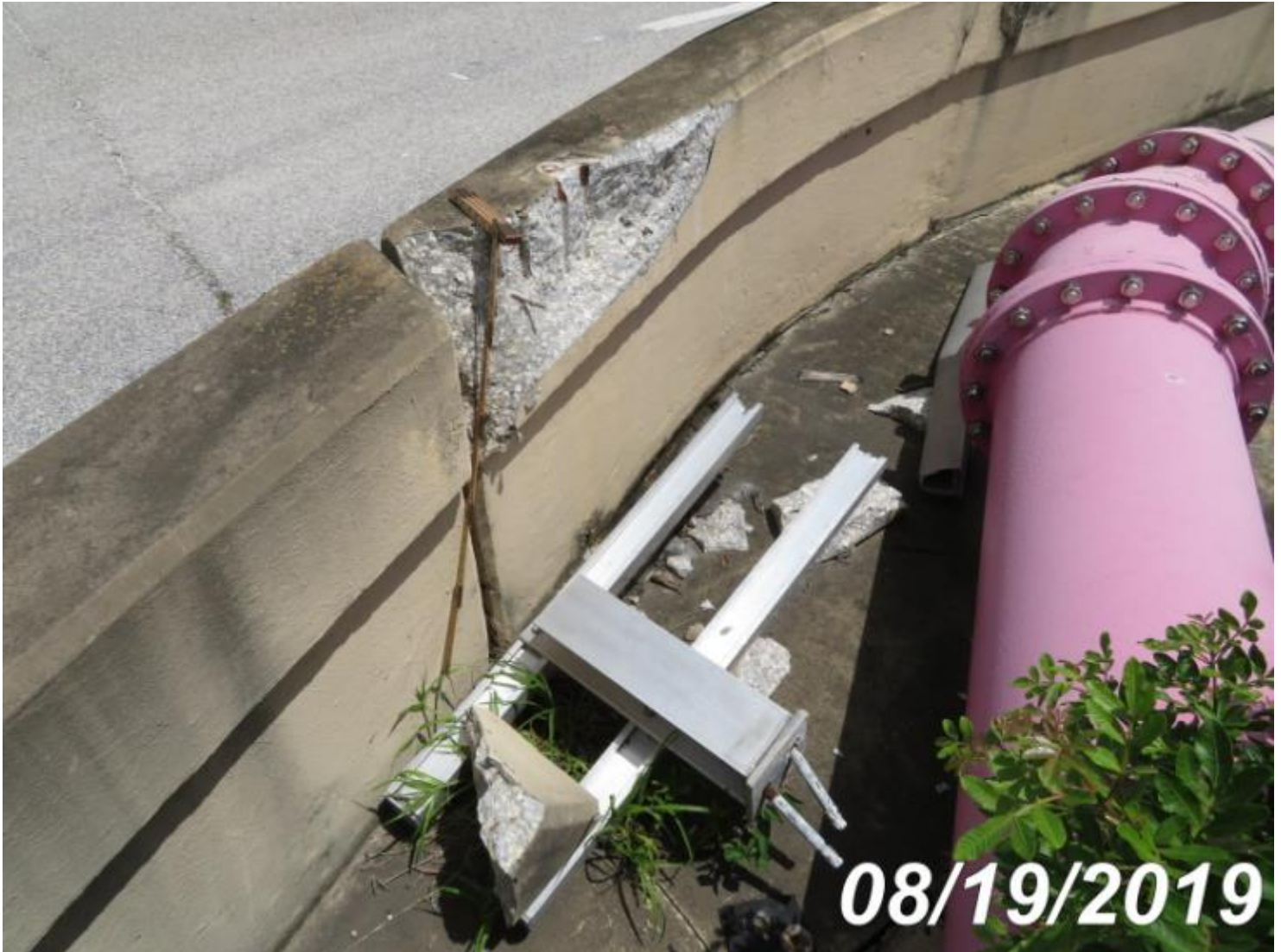
Photo 333-S02 (Unit 0: Other Bridge Railing)
