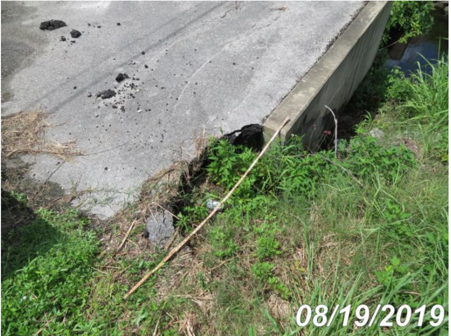
Photo 8475-S02 (Unit 0: R/Conc Walls)
