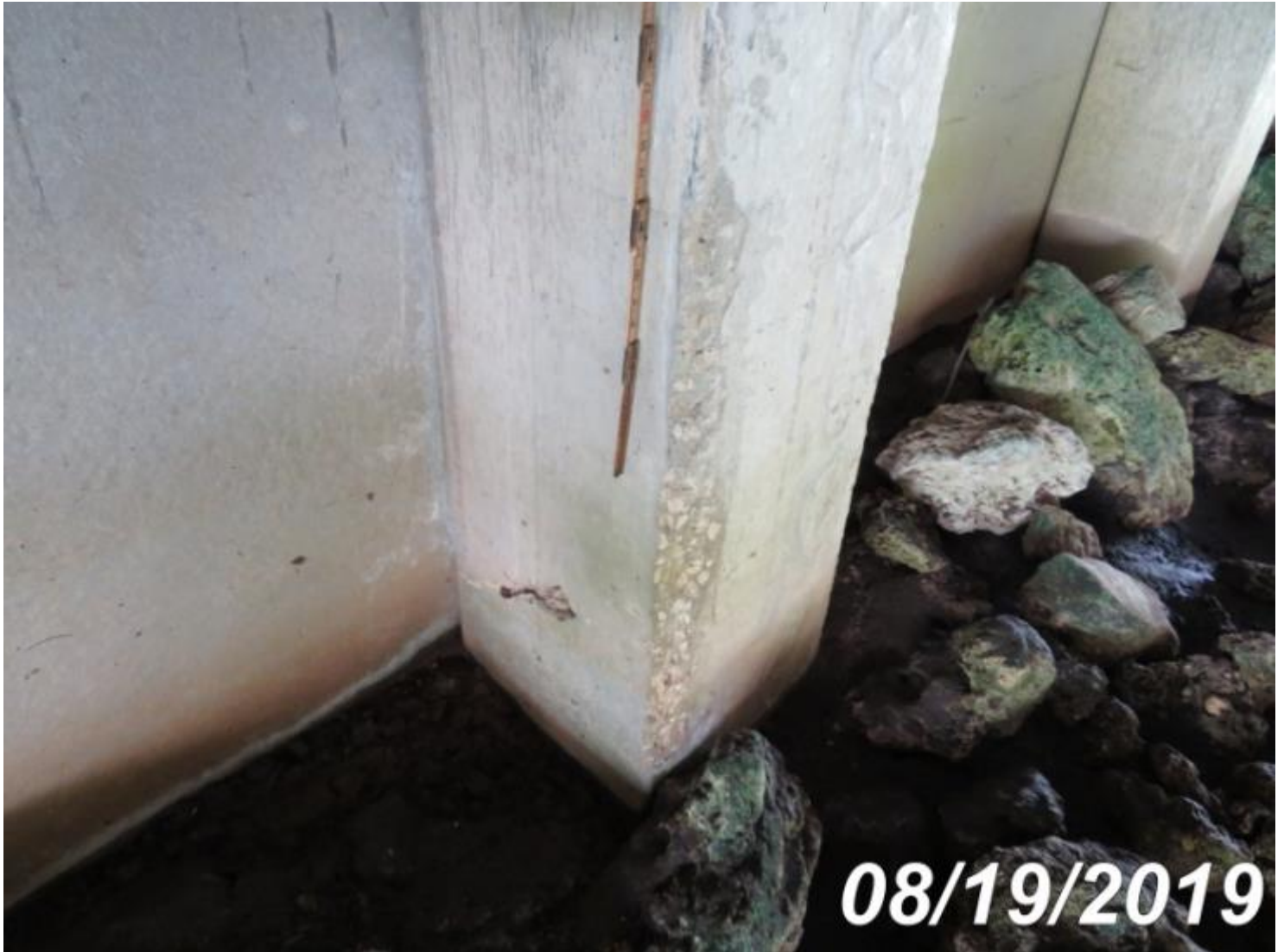
Photo 226-S01 (Unit 0: Pre Conc Pile)
