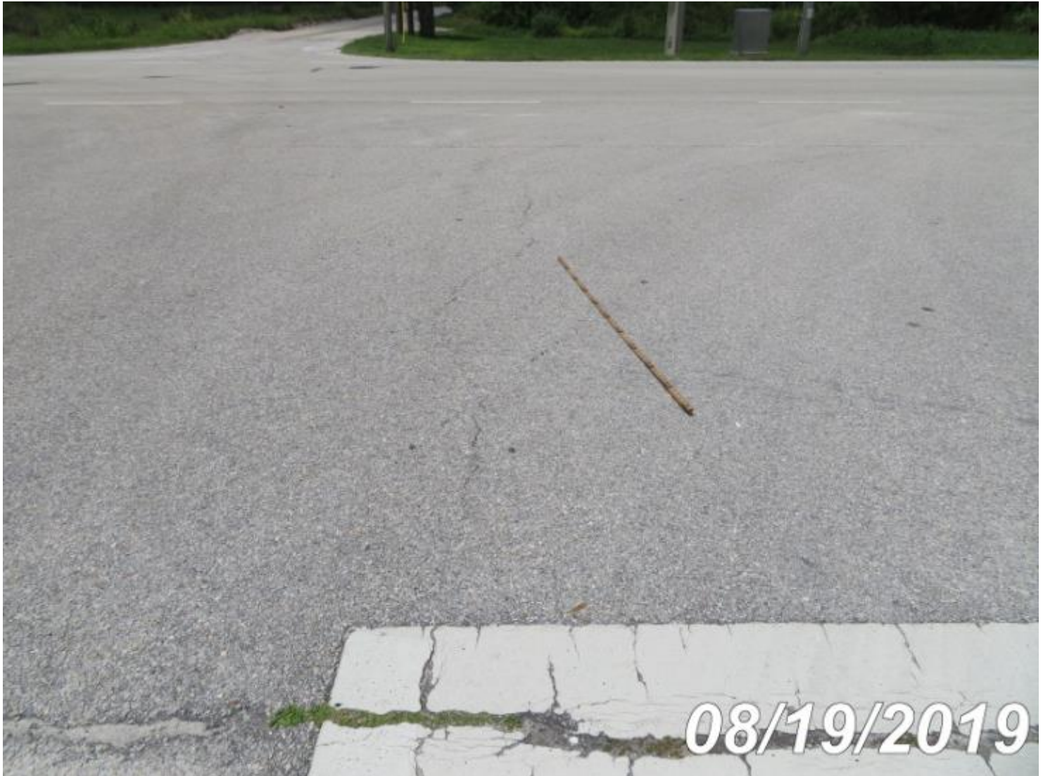
Photo 321-S02 (Unit 0: Re Conc Approach Slab)
