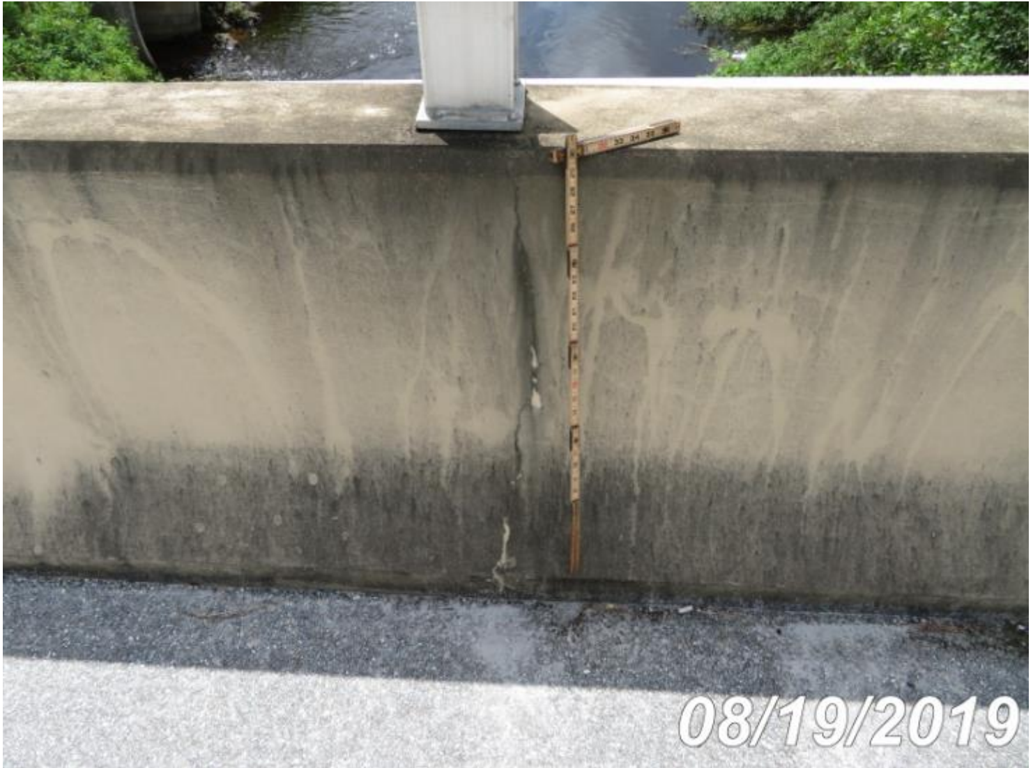
Photo 333-S03 (Unit 0: Other Bridge Railing)
