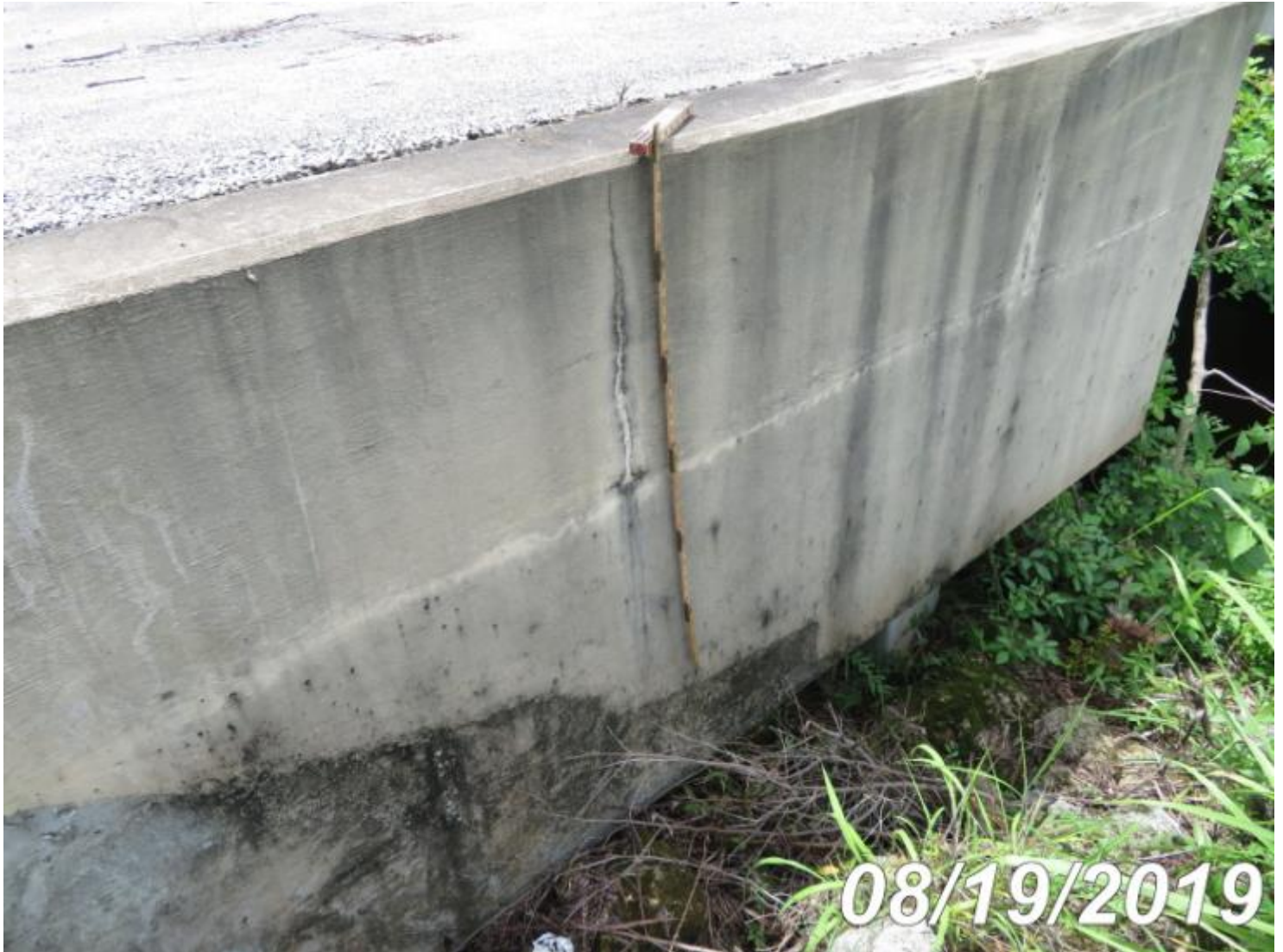
Photo 8475-S01 (Unit 0: R/Conc Walls)
