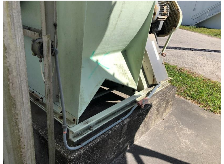
10. View of outside housing and frame– Samples 14 & 15 – (Green Paint)
