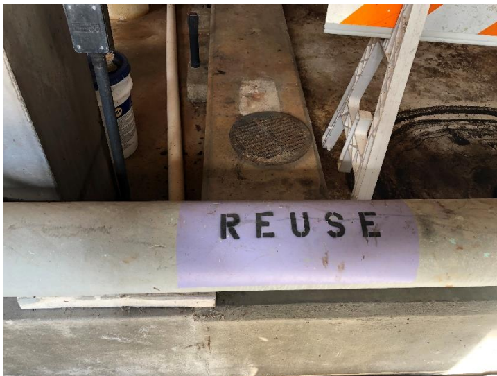
7. View of reuse pipe– Sample 11– (Grey Paint)
