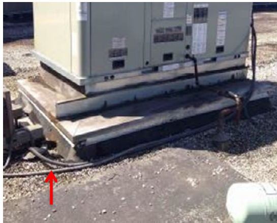
Electrical conduit is resting on the roof.
