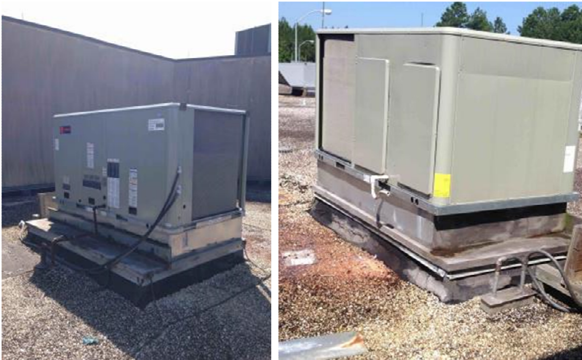
RTU-3 was placed on the existing roof curb.
