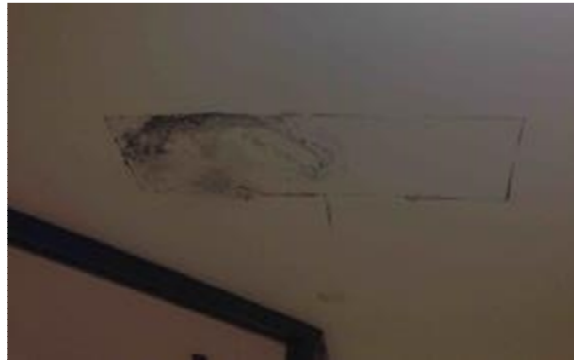
The ceiling in Intake 103 in the booking area shown above has microbial growth.
