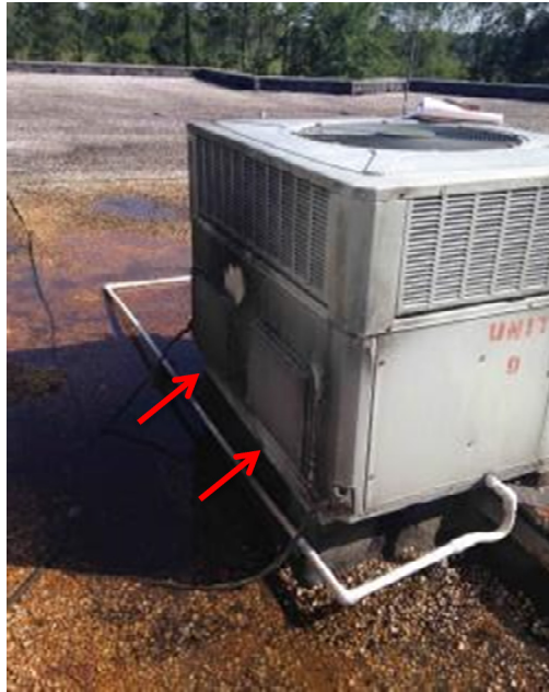
No outside air is entering RTU-8.
