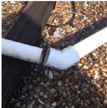
Condensate piping is disconnected.
