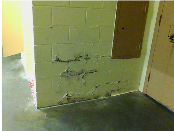
Paint is delaminating.
