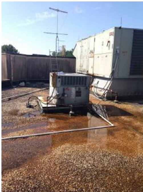
RTU-8 is surrounded by standing water.
