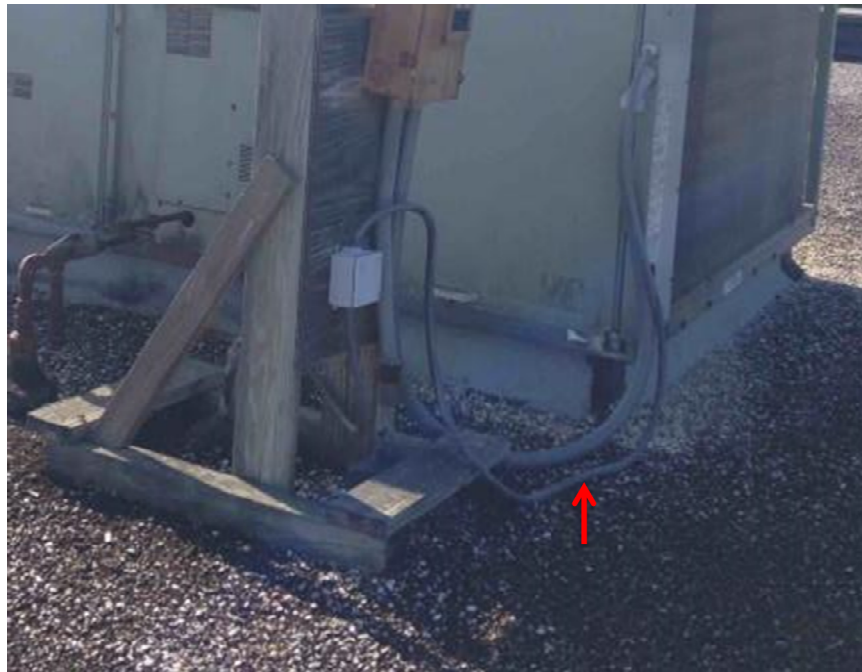
Electrical conduit is resting on the roof.
