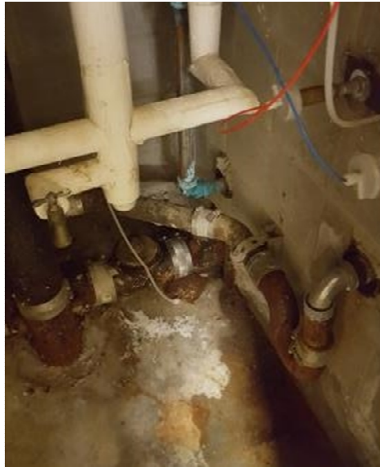
There is surface rust on cast iron piping in the housing unit chases.
