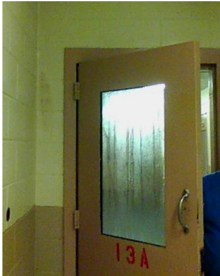
The glass is sweating in the door of the corridor connecting to the kitchen.
