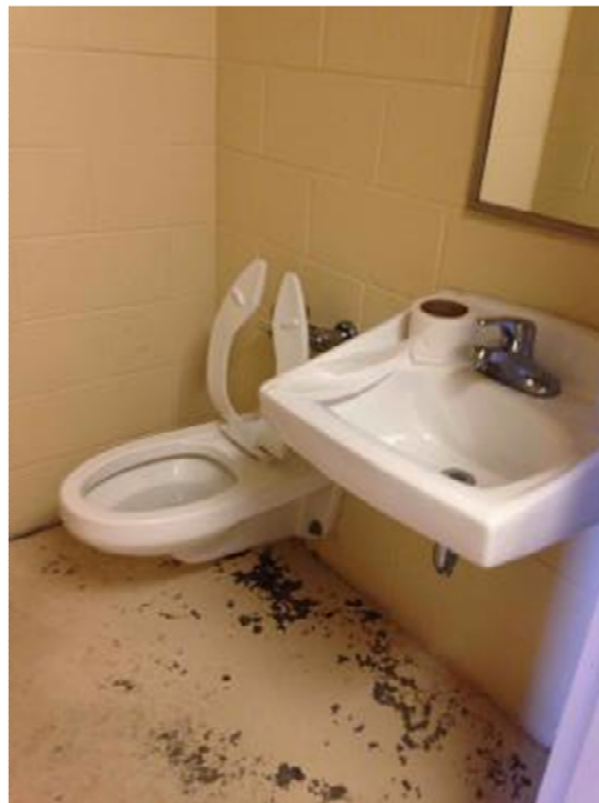
The staff toilet next to the juvenile holding room does not have ADA compliant fixtures or ADA compliant insulation on the piping below the lavatory.
