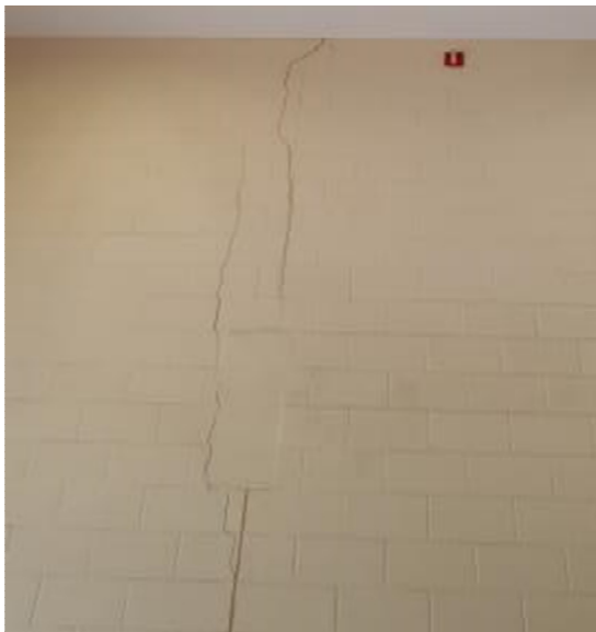
There is a crack in Multipurpose Room A100.
