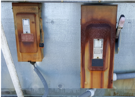
Square D Safety Switches (RTU-2) – Poor Condition
