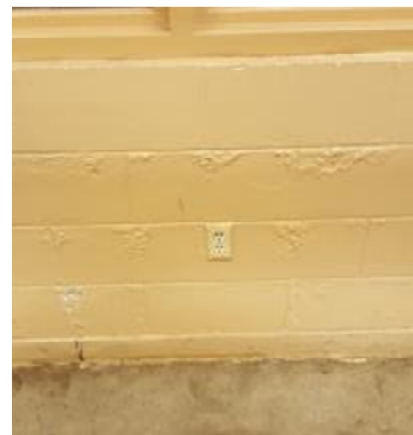
The paint is delaminating due to apparent migration moisture from the CMU block.
