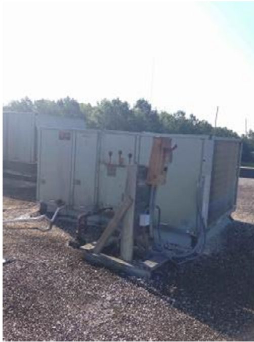
RTU-6 has rust and microbial growth.
