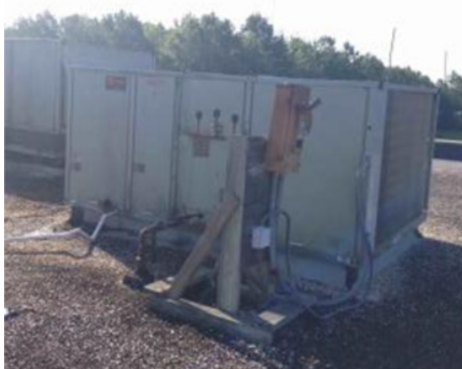
This rooftop unit has a rusted safety switch that is mounted on wood.
