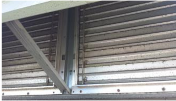
Pictured above are closed louvers to RTU-4.
