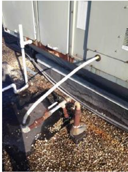
The pitch pocket is damaged.
