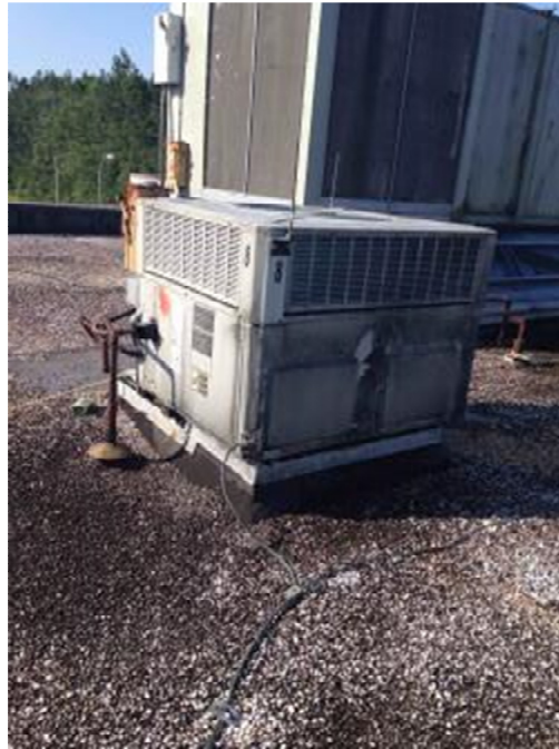
RTU-9 has rust and microbial growth.
