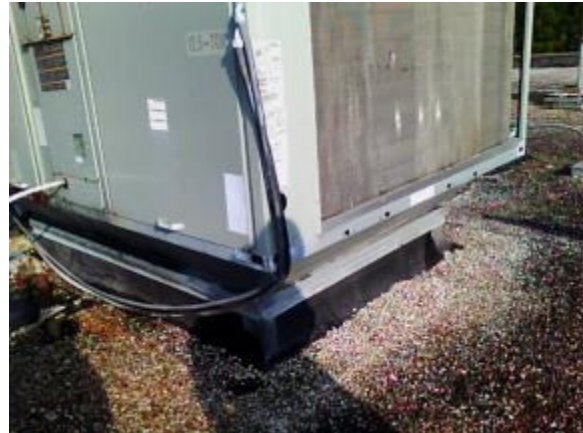
The roof curb temperature is about 120°F.
