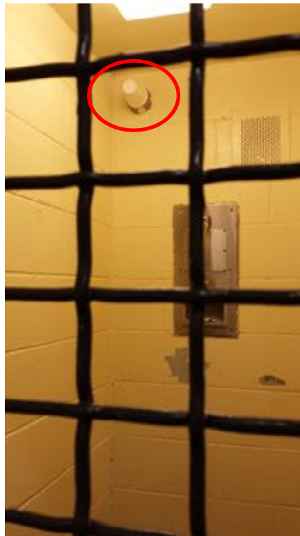
The sprinkler head in the shower stall above is currently covered with a cup.
