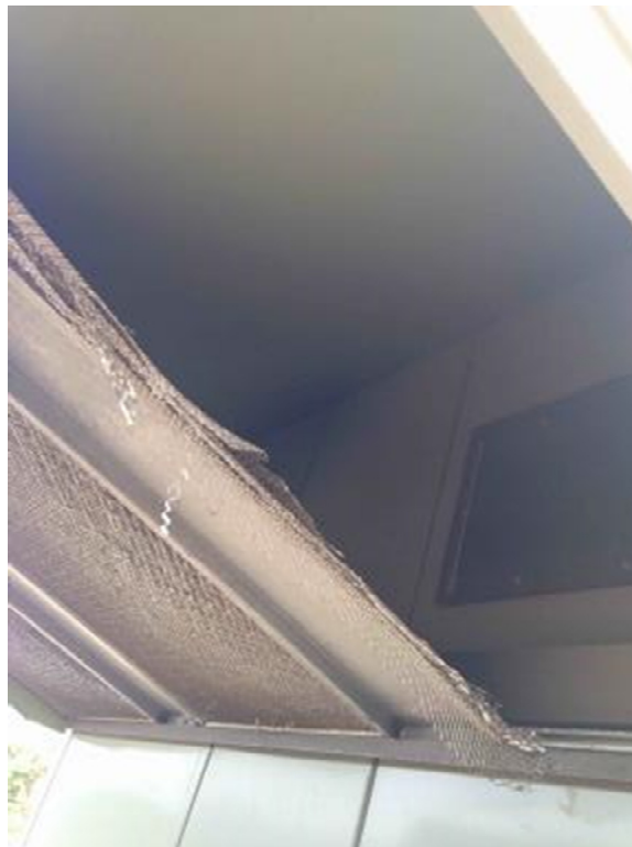
The bird screen is torn on the intake side of the unit.
