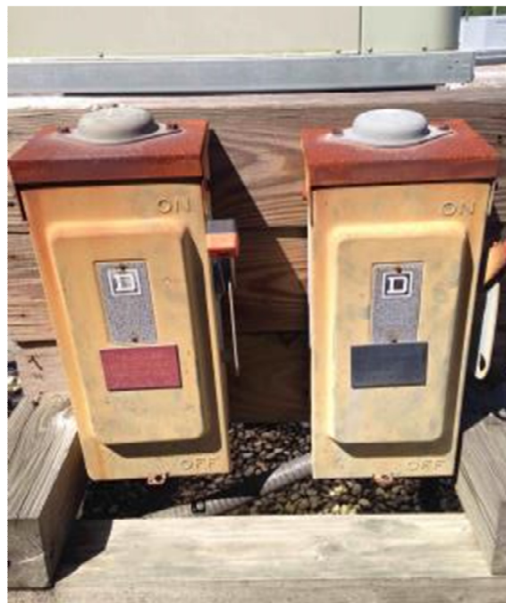
The corroded disconnects are mounted to wood.
