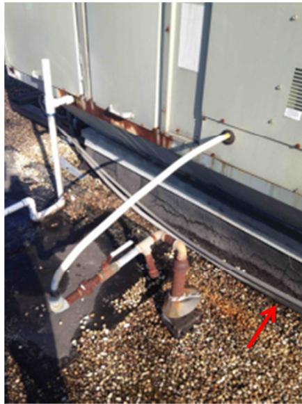
Electrical conduit is resting on the roof.
