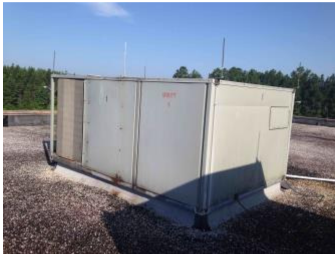
There is visible rust on the RTU-6 roof curb.
