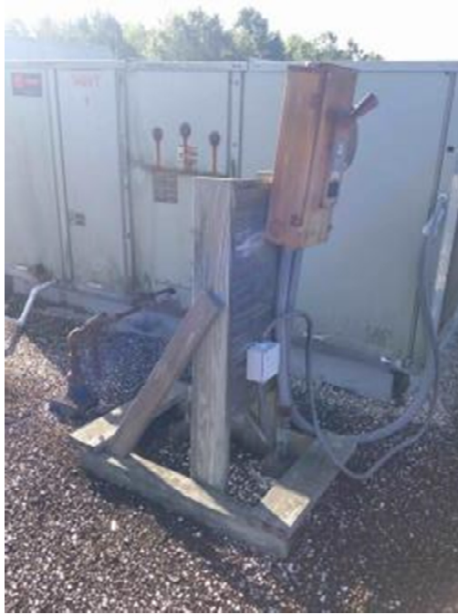
The corroded disconnect is mounted to wood.
