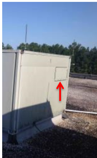
No outside air is entering RTU-6.
