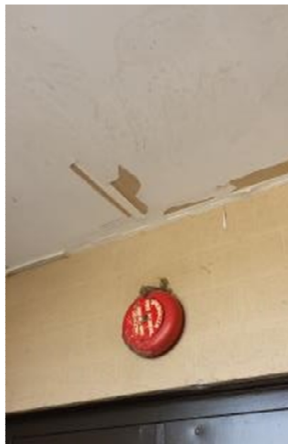
The paint is coming off the drywall at the boiler room entrance.
