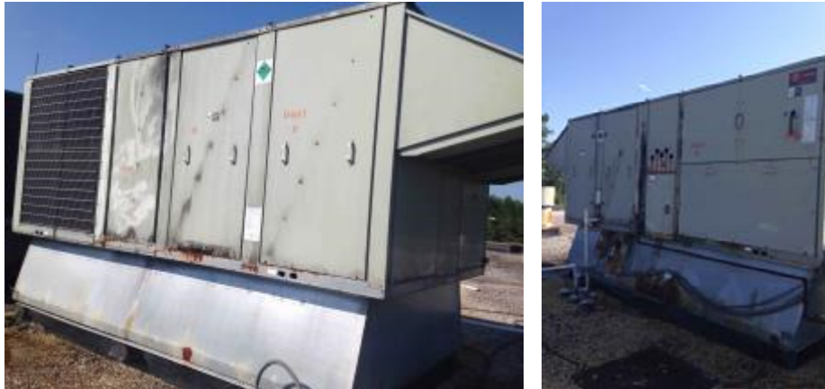
RTU-2 has rust and microbial growth.
