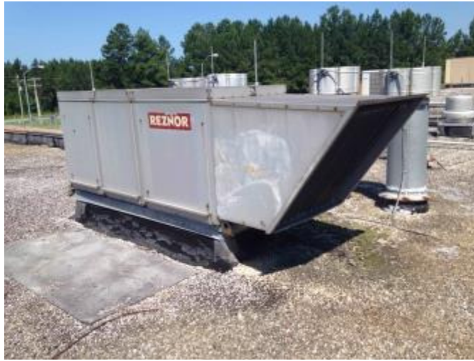
MAU-1 has rust on the exterior of the unit.
