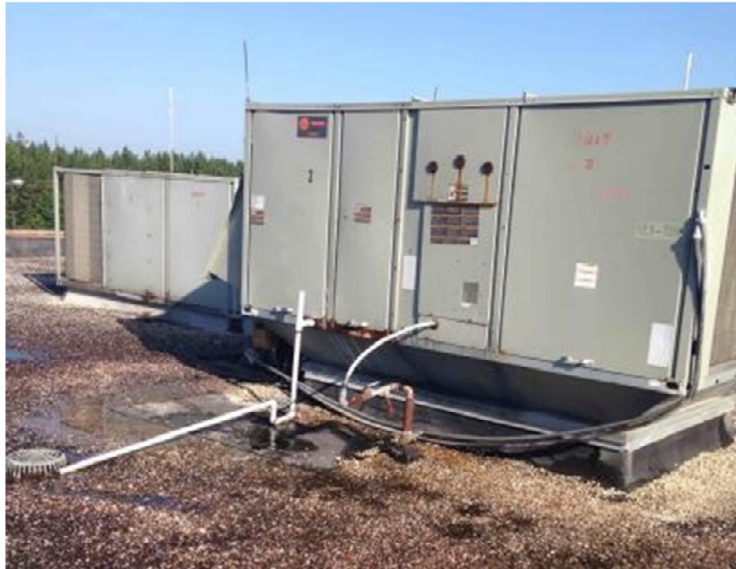
RTU-5 has rust and microbial growth.
