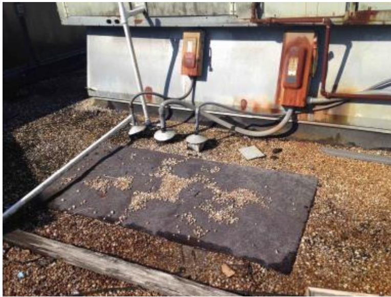
There is visible rust on the RTU-1 roof curb.
