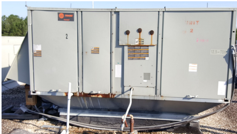
Electrical conduit not supported (RTU-5)
