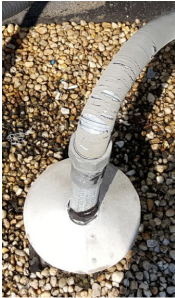
Deteriorated sunlight-resistant jacket (RTU-1)
