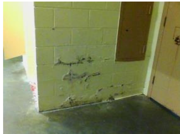
The paint is delaminating due to apparent migration moisture from the CMU block. Temperatures at this wall are as low as 54.5°F.
