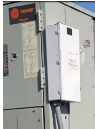
Eaton Safety Switch (RTU-4) – Good Condition
