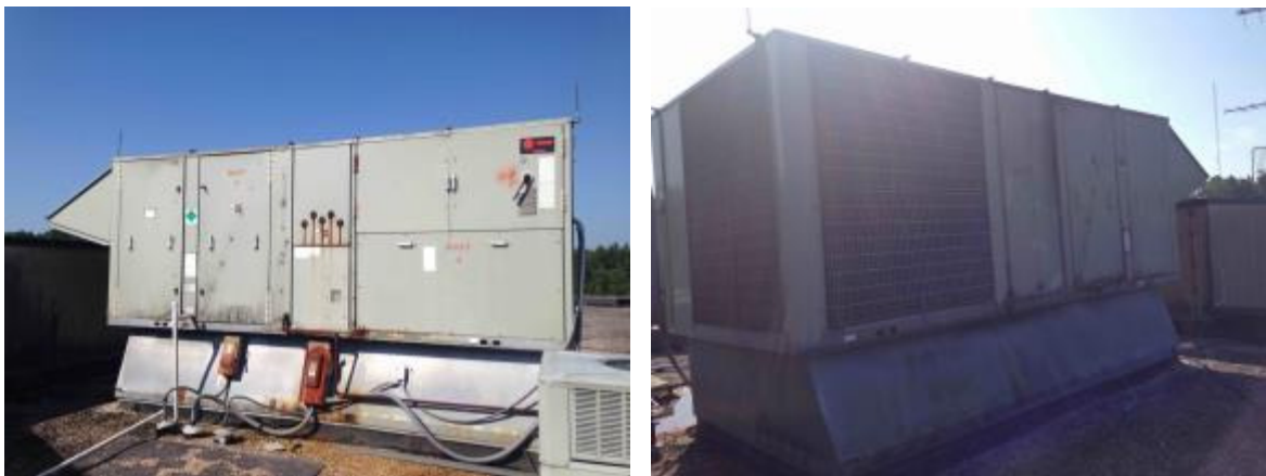
RTU-1 has rust and microbial growth.
