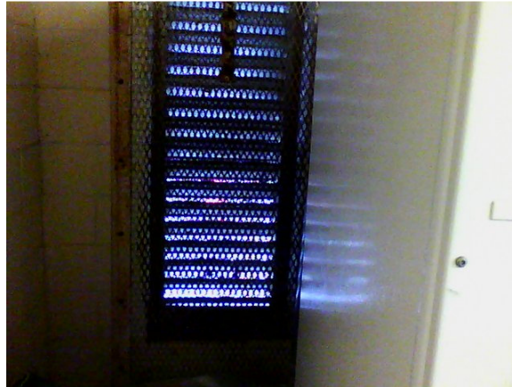
Typical louver allowing outside air to be pulled directly into the building when the exhaust system is running.
