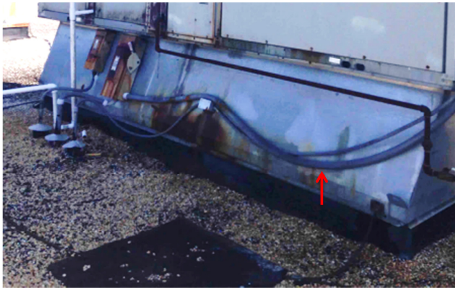
There is visible rust on the RTU-2 roof curb and conduit is not properly supported.
