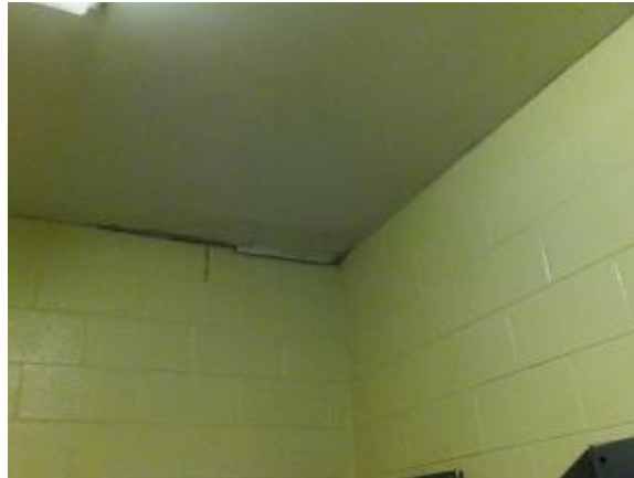
There is a gap between the wall and ceiling in Shower F103.
