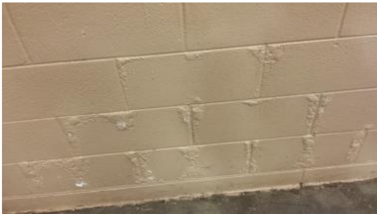
The paint is delaminating due to apparent migration moisture from the CMU block.
