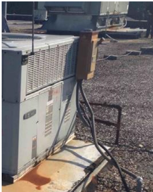
The corroded disconnect is attached to the rooftop unit.
