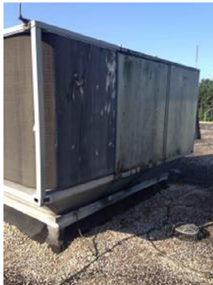
The fins are torn and delaminating.
