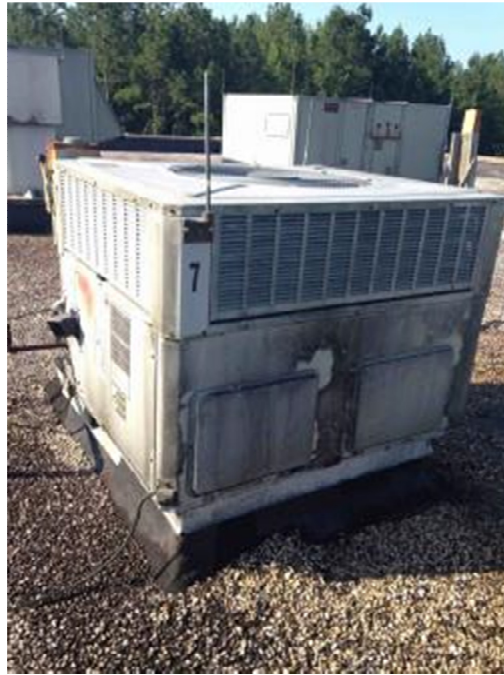
RTU-7 has rust and microbial growth.
