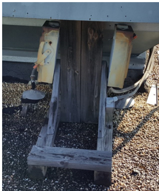
This rooftop unit supply fan safety switch is in the OFF position.
