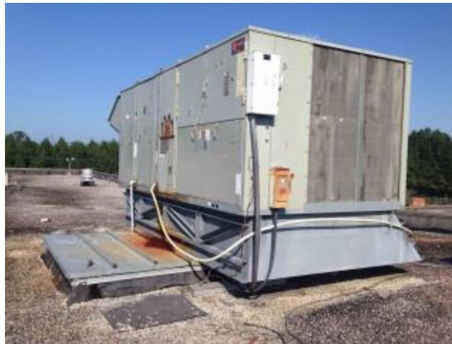
RTU-4 has rust and microbial growth.
