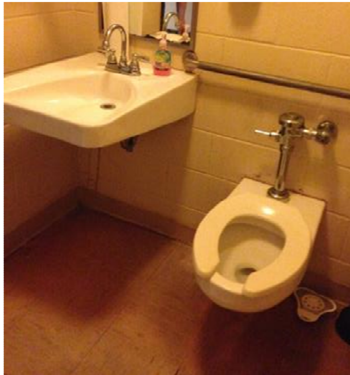
The lavatory does not have ADA compliant insulation on the piping below the lavatory in Room 113.
