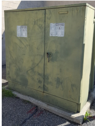
Pad mounted utility transformer
