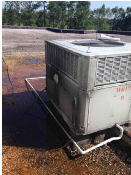
RTU-8 has rust and microbial growth.
