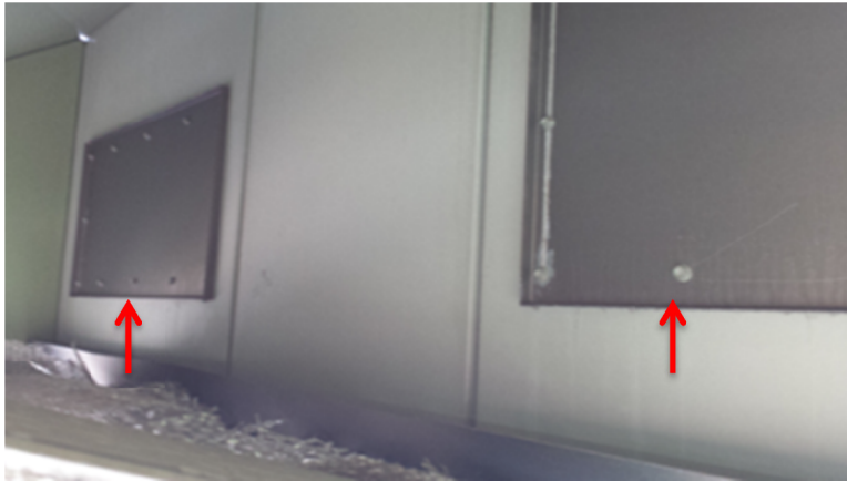
Pictured above are blanked-off louvers to RTU-1.
