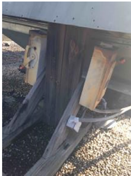
The corroded disconnects are mounted to wood.
