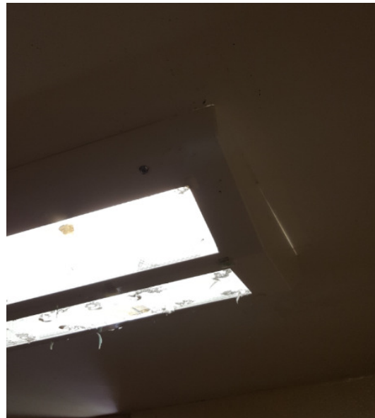
Light Fixtures in Cell Block D & H not flush with ceiling. Note gap where light is leaking out from behind the fixture.
