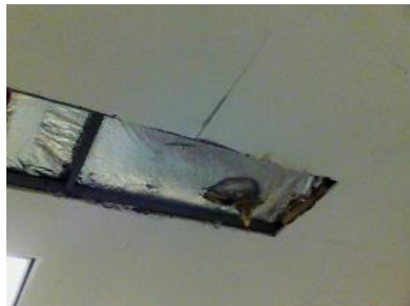
The drywall is being replaced due to condensation. The ductwork also has microbial growth.
