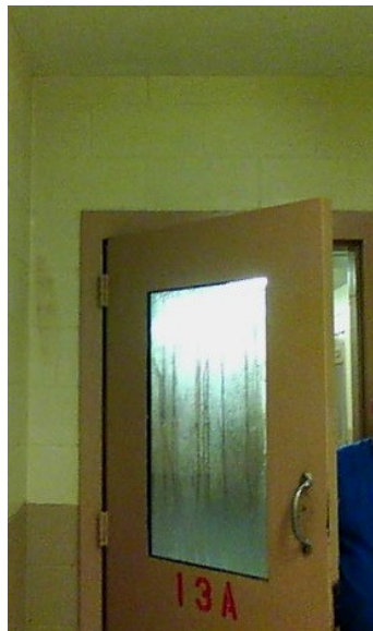
Moisture visible on the door suggests there may be moisture above the ceiling as well.
