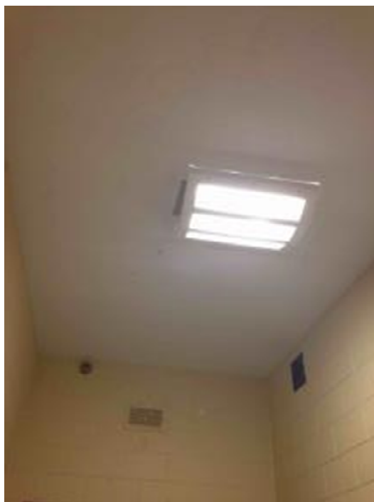
Light fixture is not penal type in Juvenile Holding 112.
