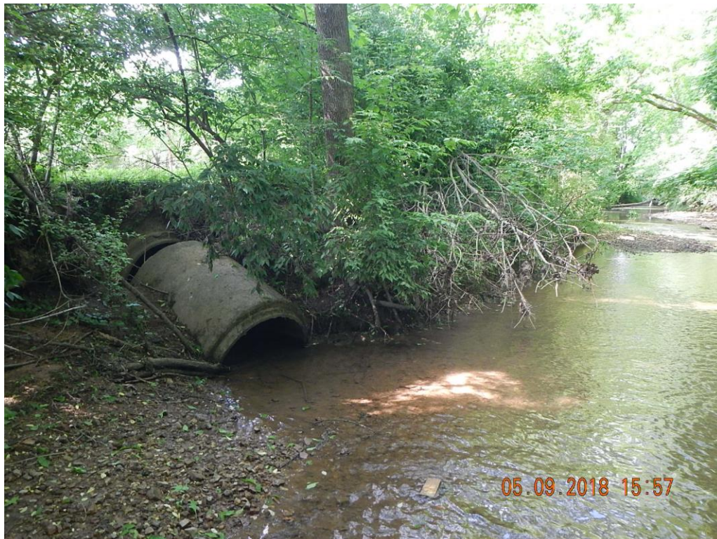
Figure 1 Start of project at outfall repair
