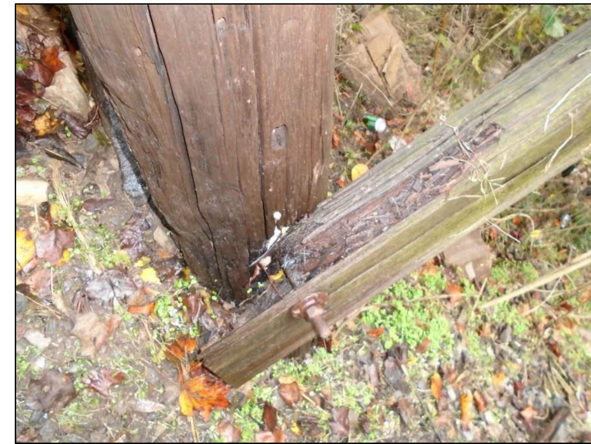
6 REPAIR PHOTO SCALE: NOT TO SCALE
