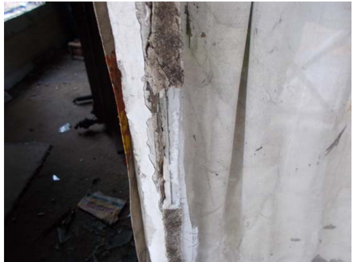
Photo 8 – Window glazing on wooden windows.
