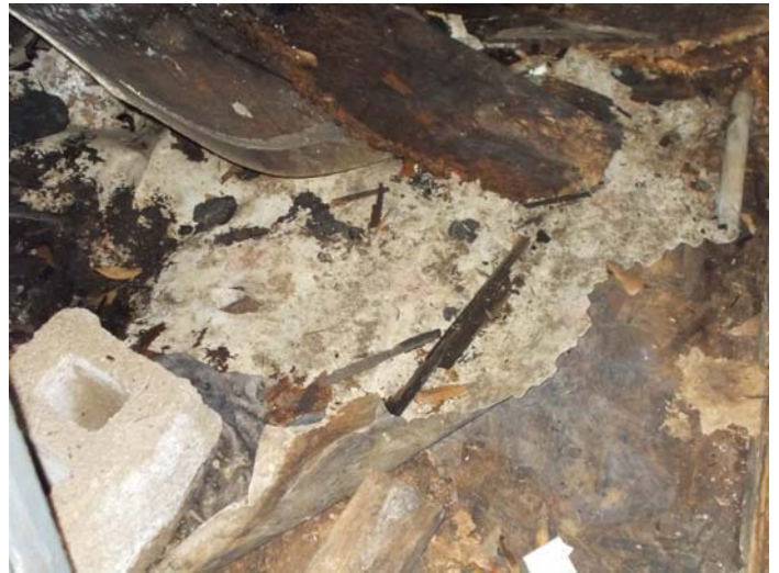
Photo 20 – Tan pattern vinyl flooring with mastic throughout bathroom.
