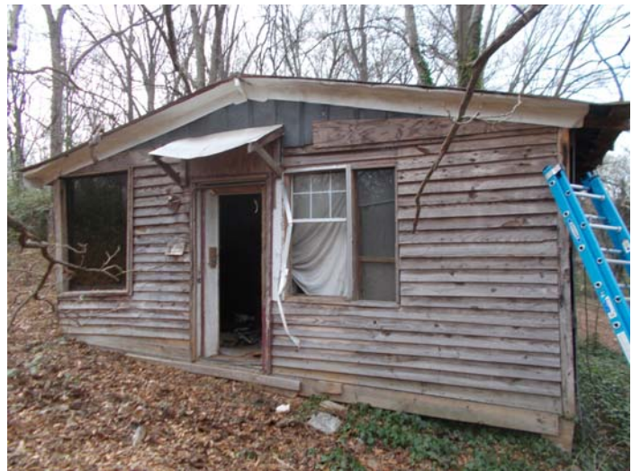
Photo 4 – Exterior rear shed.
