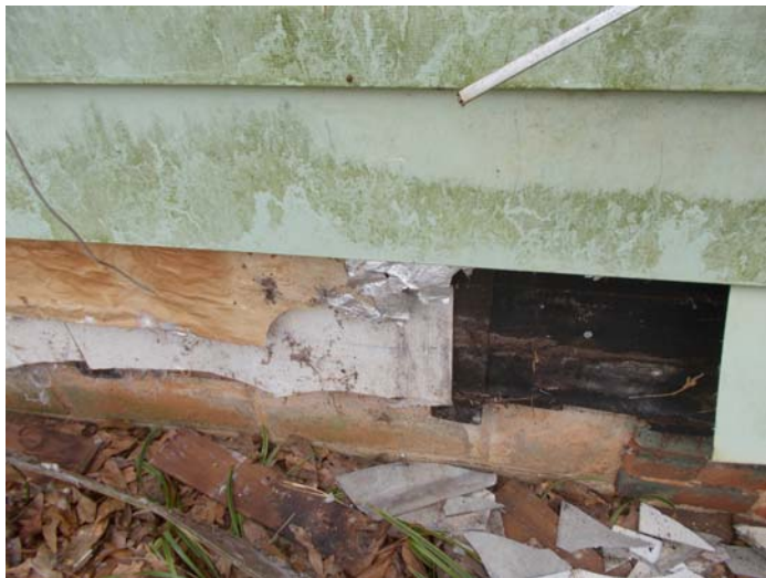
Photo 9 – Black felt paper beneath cement board siding. Brown siding paper under metal siding.
