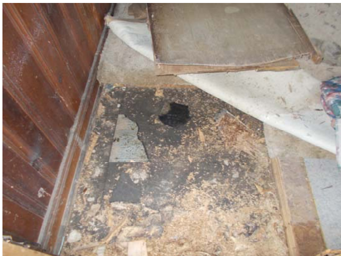
Photo 11 – Flooring felt in front right room.
