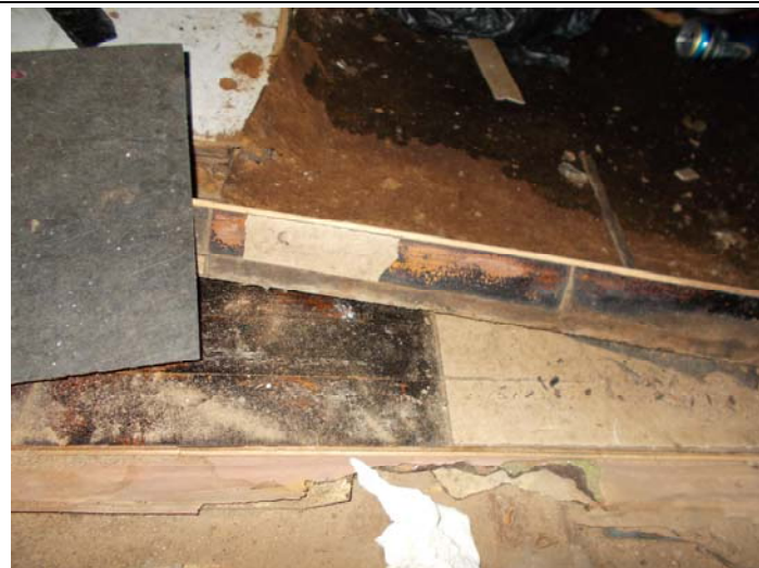
Photo 15 – Multiple layers of vinyl flooring with and without mastic in the large middle room in front of the kitchen.
