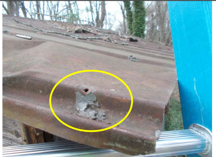
Photo 2 – Roof sealant on shed roof.
