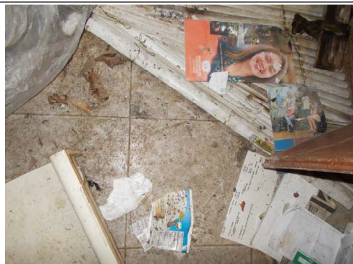
Photo 17 – Beige large square pattern vinyl flooring with no mastic in the kitchen.
