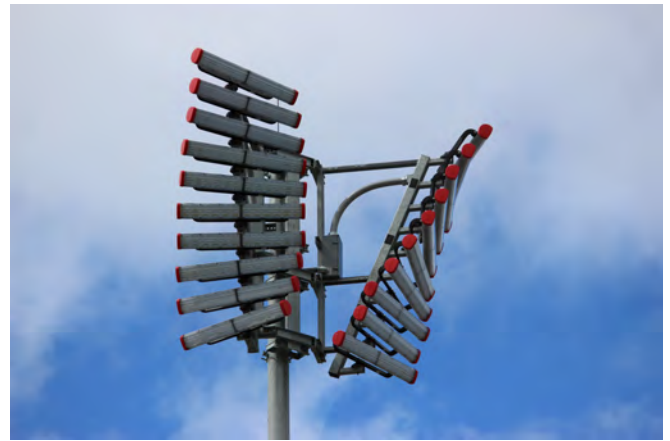
Installation at Northwest High School, Jackson, MI.
