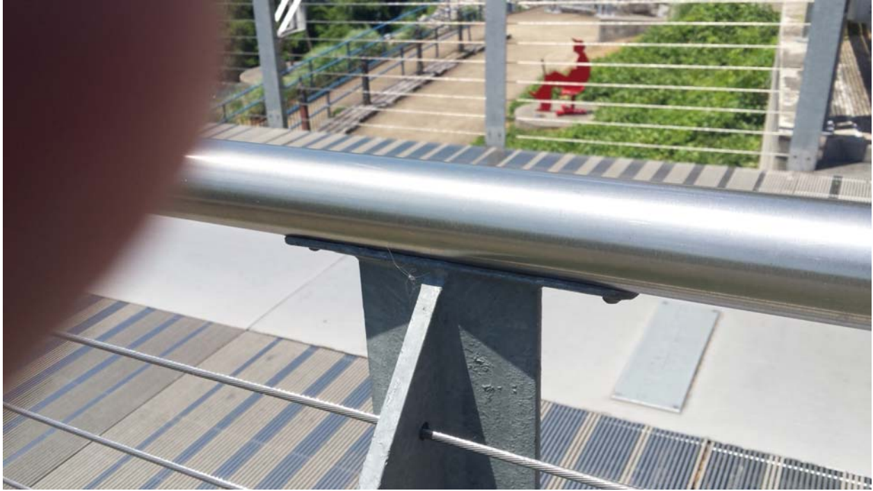
Photo of the top of the post bracket where the railing attaches:
