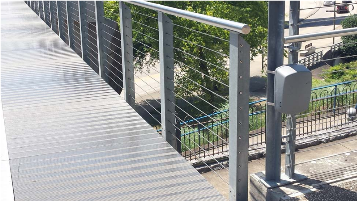
Photo of the railing, support post, and bridge deck:
