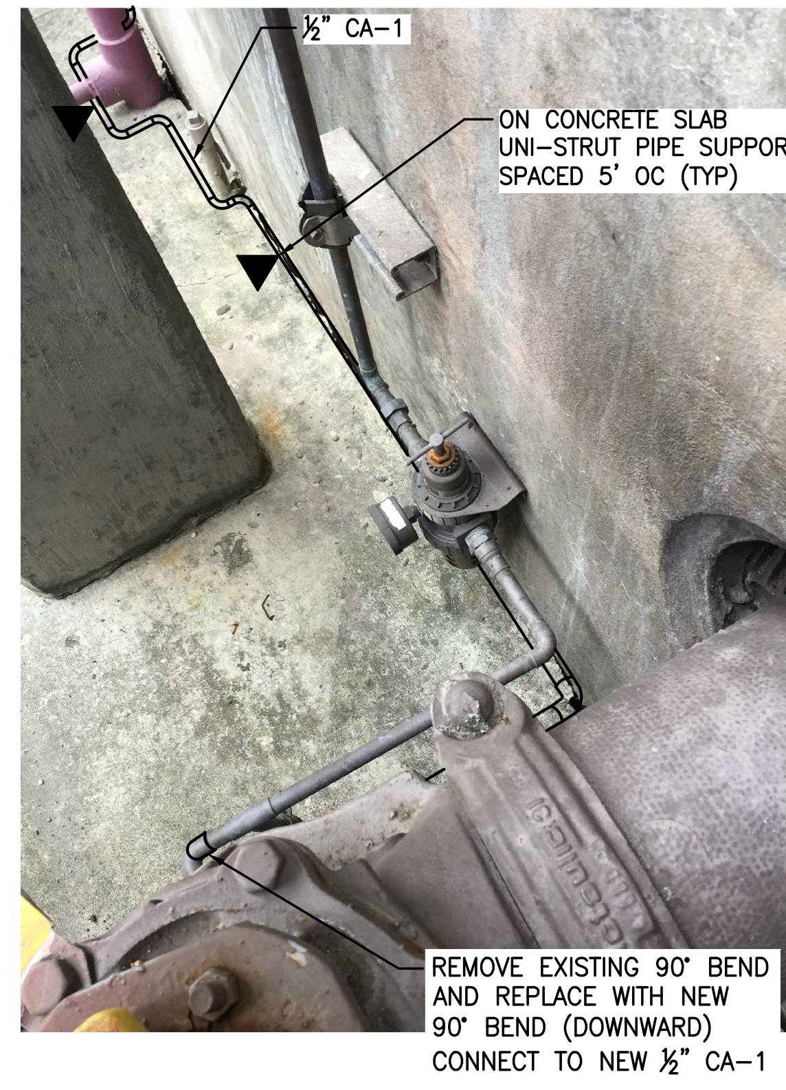
COMPRESSED AIR CONNECTION DETAIL 6 NOT TO SCALE
