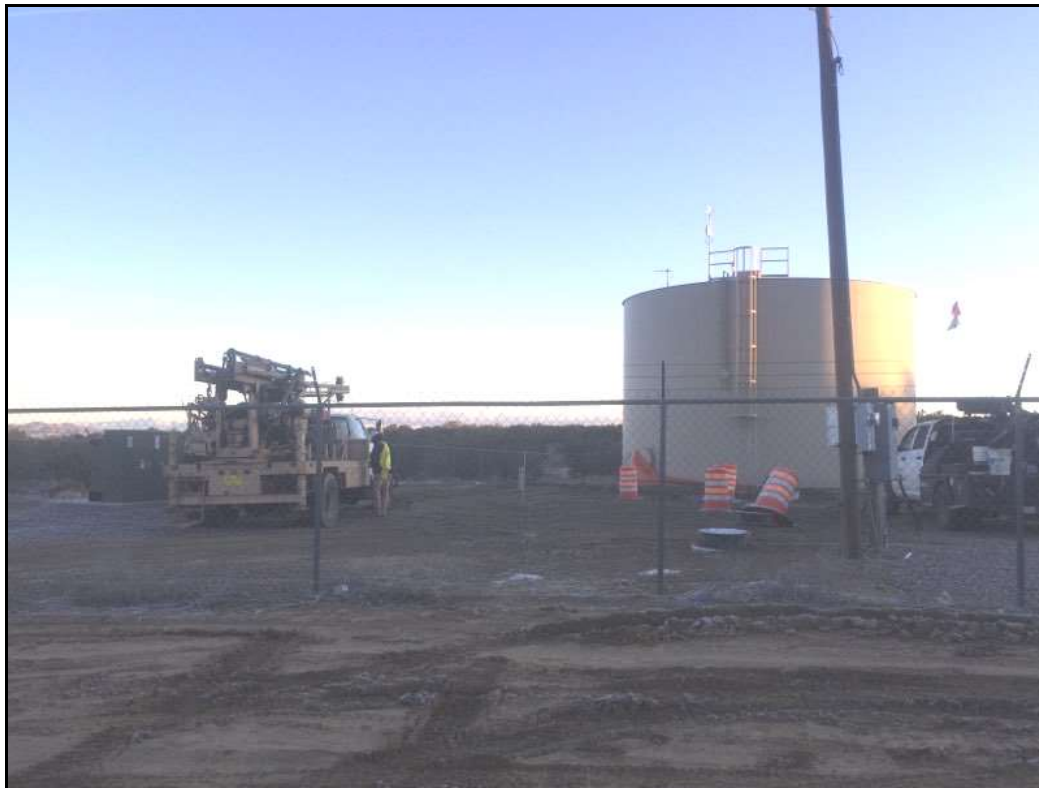
Drill Rig at Boring B-1 View to the North
