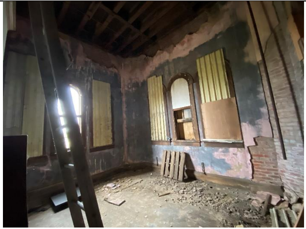
Interior NW Tower View
