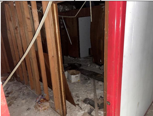
North Office Section of Facility
