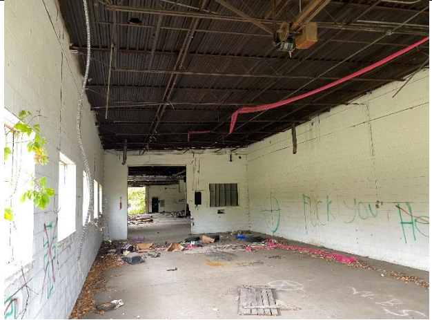
Former Car Wash Building – Interior View
