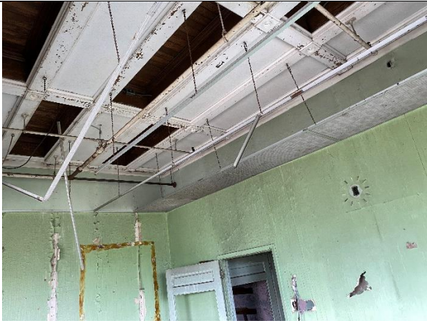
NW Office Section of Facility
