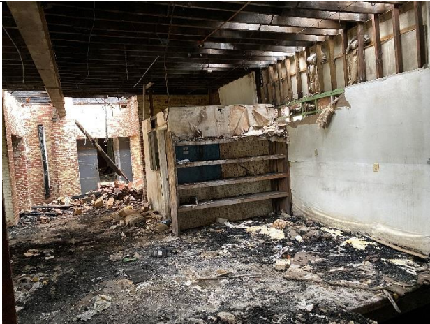
1 st Floor Office - East Section
