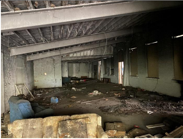
Northeast Bay of Facility
