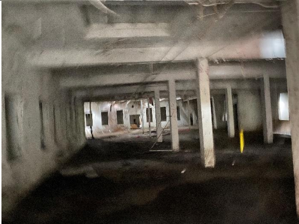
North Bay of Facility
