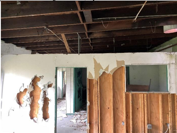
West Office Section of Facility
