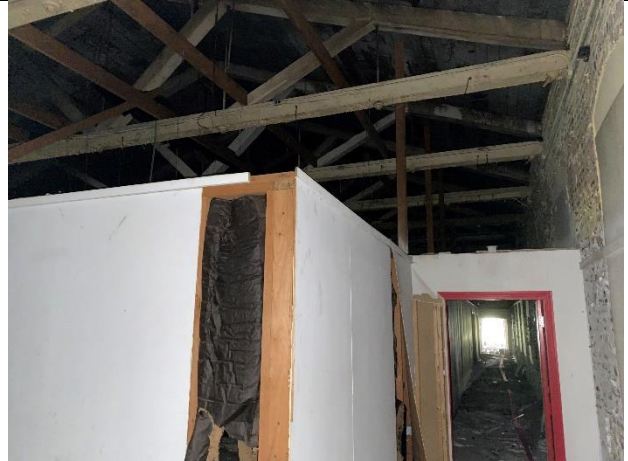
North Office Section of Facility
