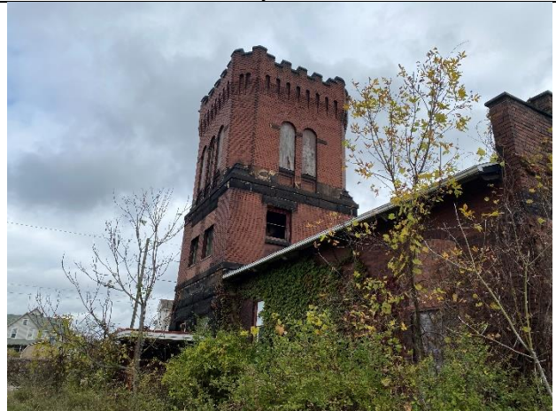
Exterior NW Tower View
