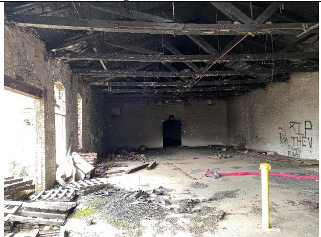
NW Bay of the Facility
