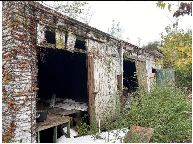
SE Storage Building associated with former car wash
