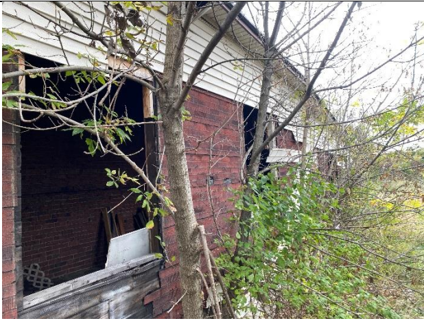
SE Section Exterior – Vinyl Siding over Asphalt Siding
