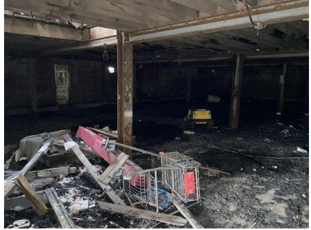
Basement View – Under East Section of Facility
