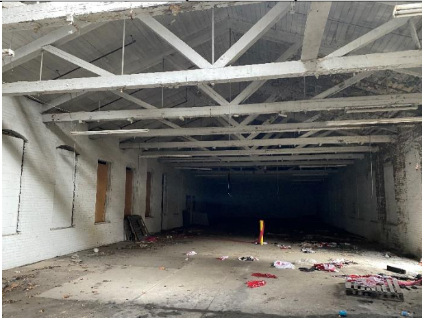
SW Bay of the Facility
