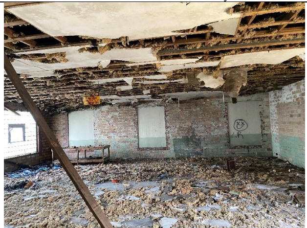
2 nd Floor – NE Section of Facility
