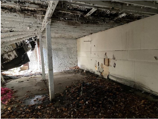
South Storage Section (Drywall Section Remains)
