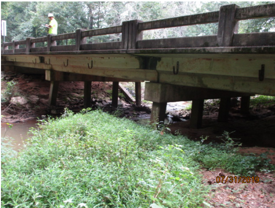
Upstream, Look North
