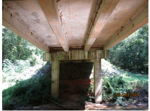
Look north at bent 3
