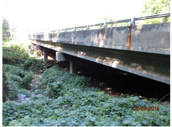
Downstream, Looking South
