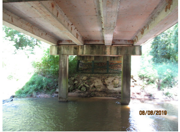
Looking South at bent 2
