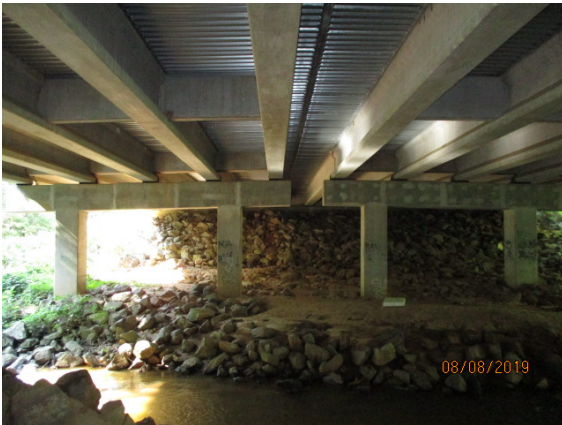
Looking South toward Bent 2
