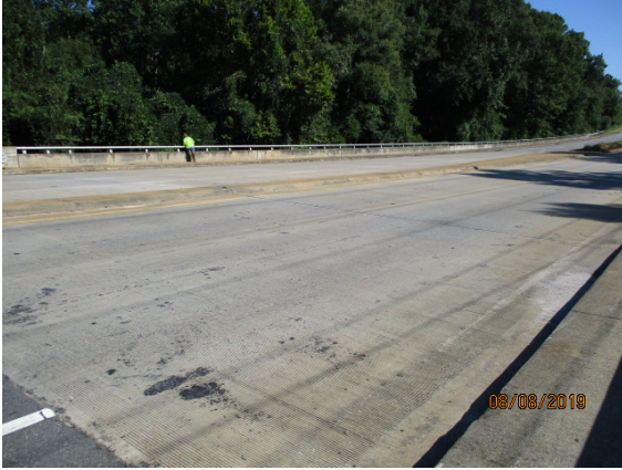
Typical of deck
