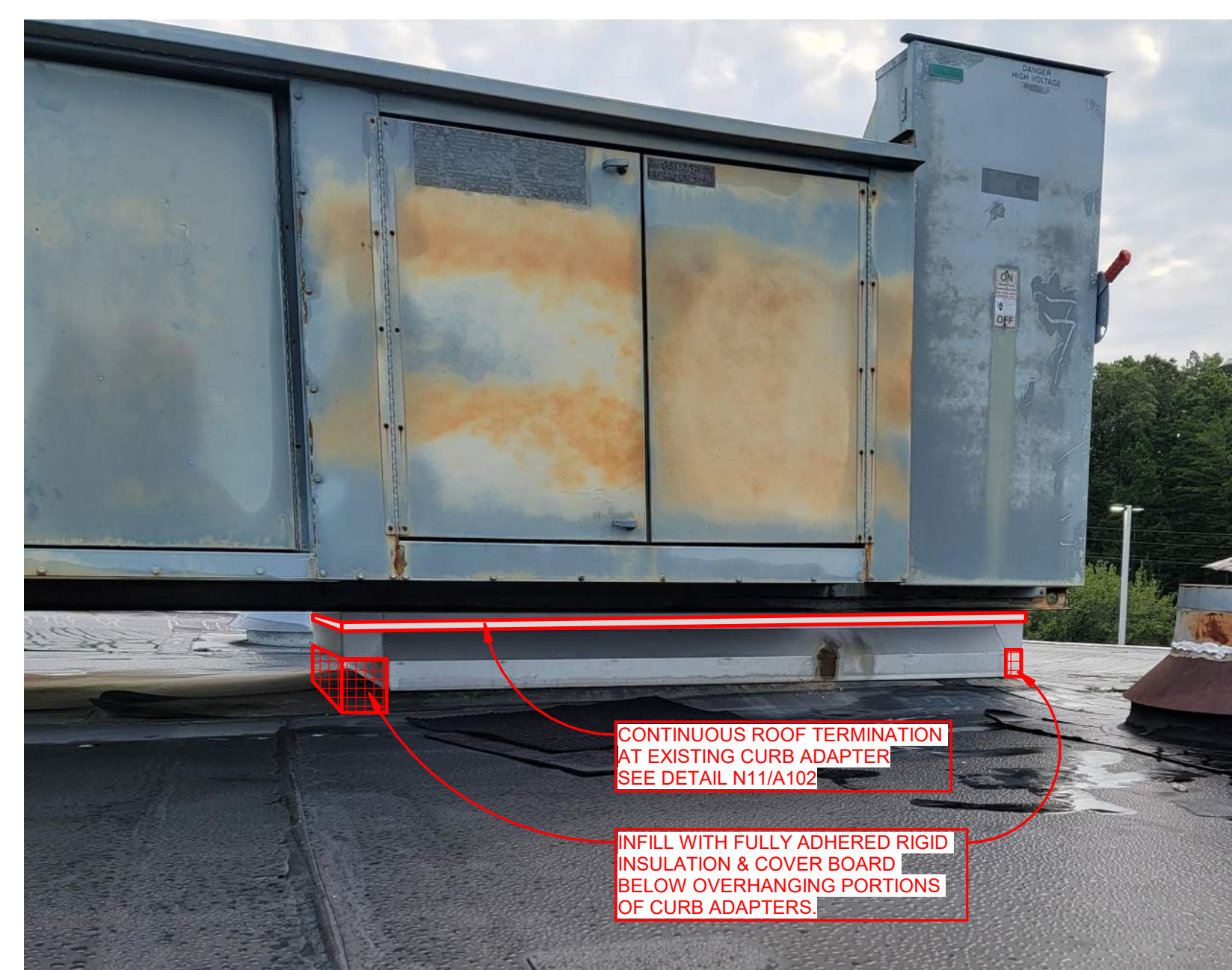
D10 Roof Detail - RTU-2 Curb Adapter A102 3' = 1'-0"
