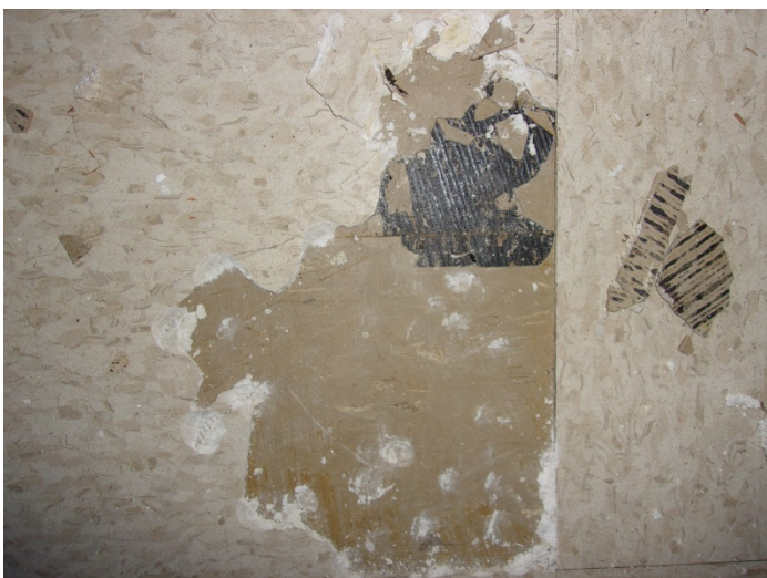
Photo 23 – Typical view of 12"x12" brown streaked floor tile and mastic (bottom layer) assumed positive in Buildings 7 to 35.
