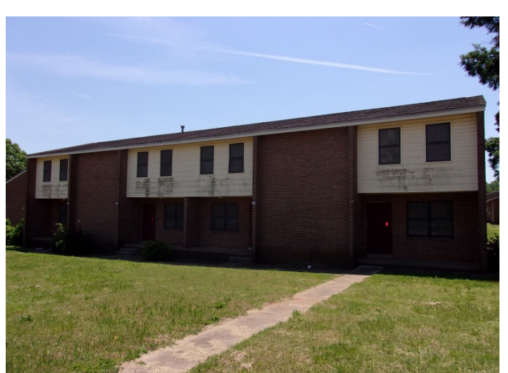
Photo 24 – Typical view of a 2-story, 4-unit building.
