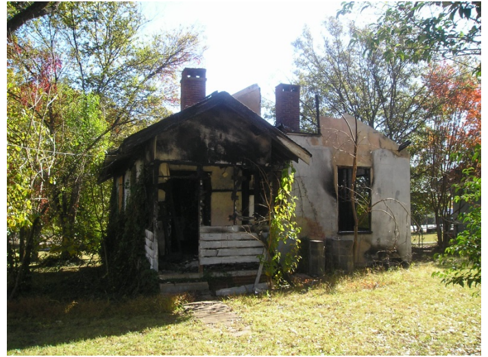
Photo 14 – Rear view of structure.
