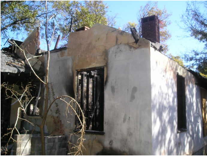
Photo 13 – Rear view of structure.
