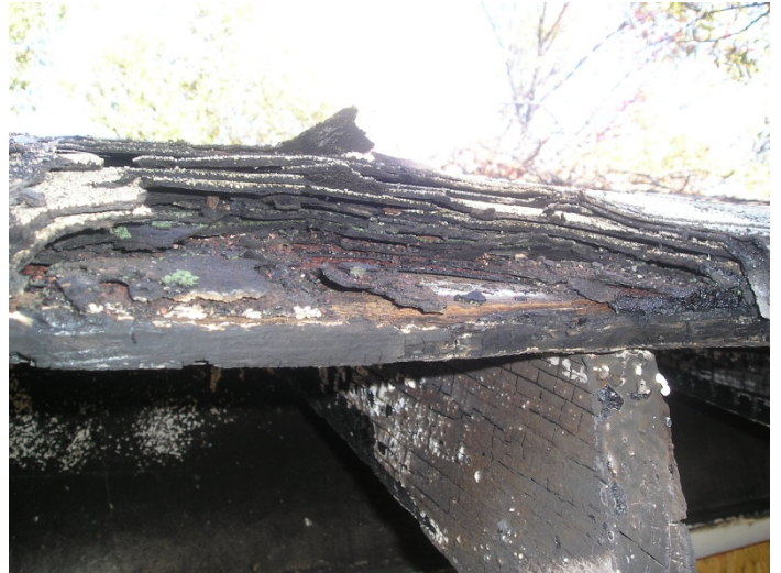
Photo 2 – Multi-layers of roof shingles.
