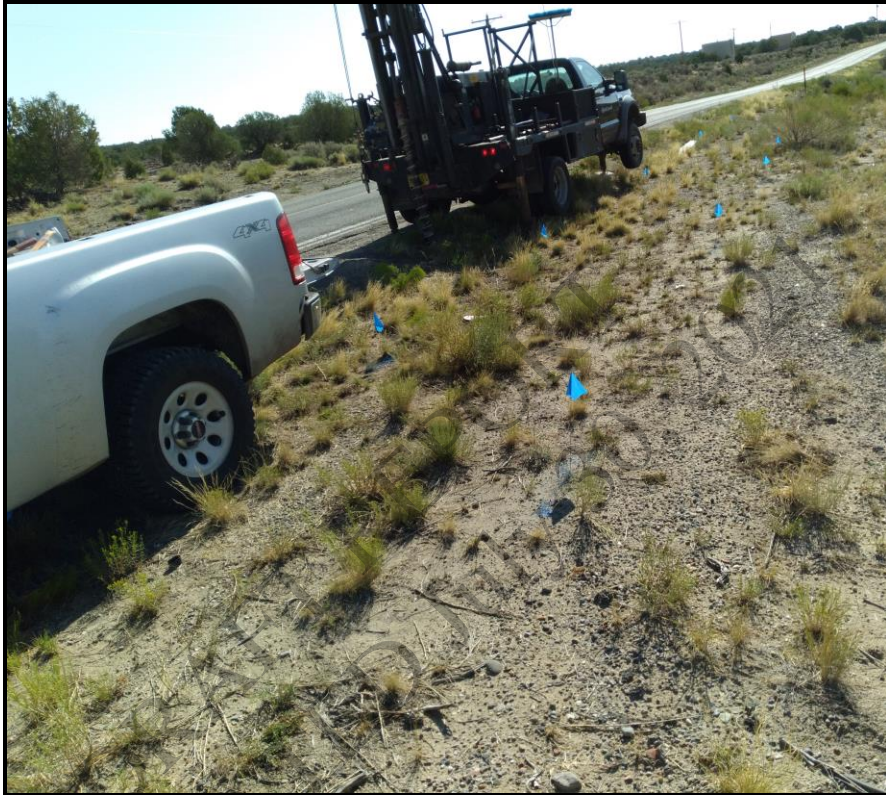
View of Drill Rig at Boring B-29 View to the East
