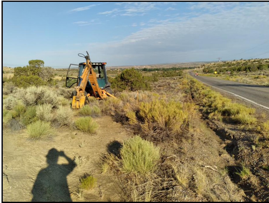
View of Backhoe at Boring TP-8 View to the West
