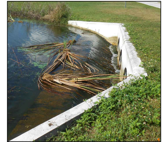
EXISTING CONCRETE HEADWALL AND WEIR
