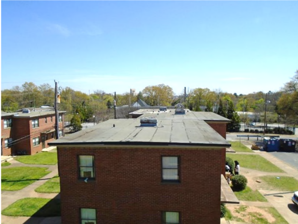
Photograph 13 - BLDG 3 – Overview of Modified Bitumen roof
