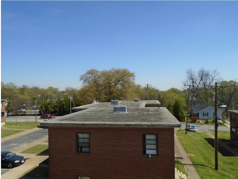
Photograph 15 - BLDG 4 – Overview looking east
