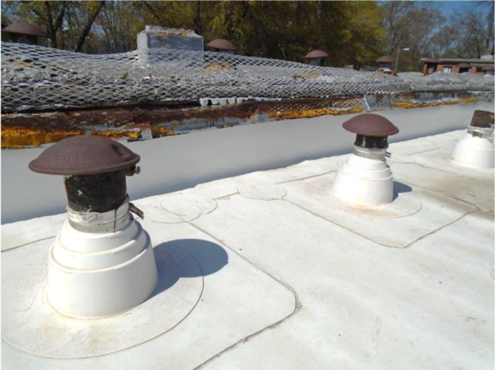
Photograph 22 - BLDG 5 – Vent pipe flashings in good condition
