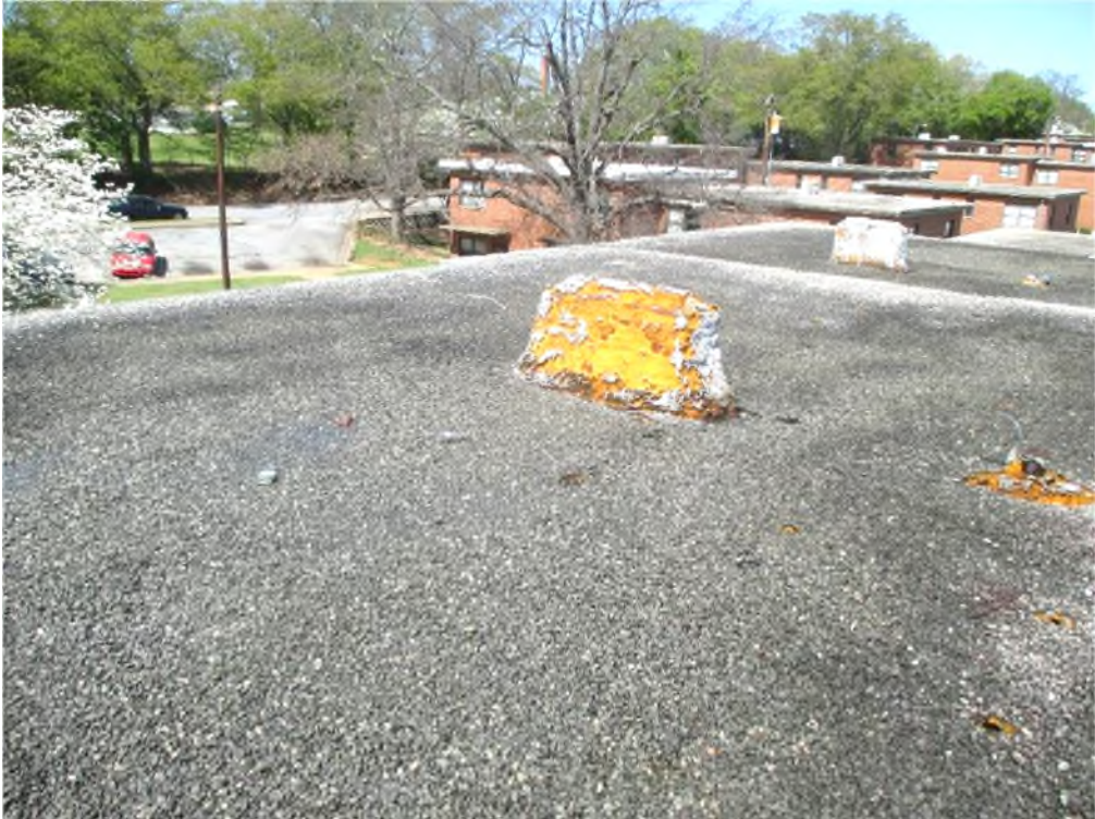
Photograph 29 - BLDG 8 – Overview looking west
