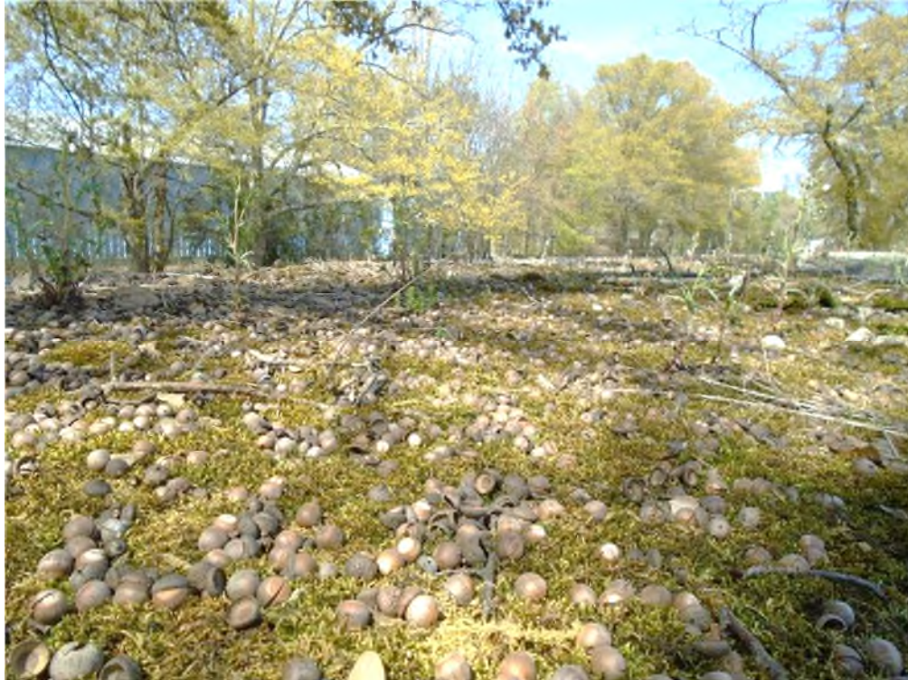
Photograph 19 - BLDG 5 – Vegetation growth
