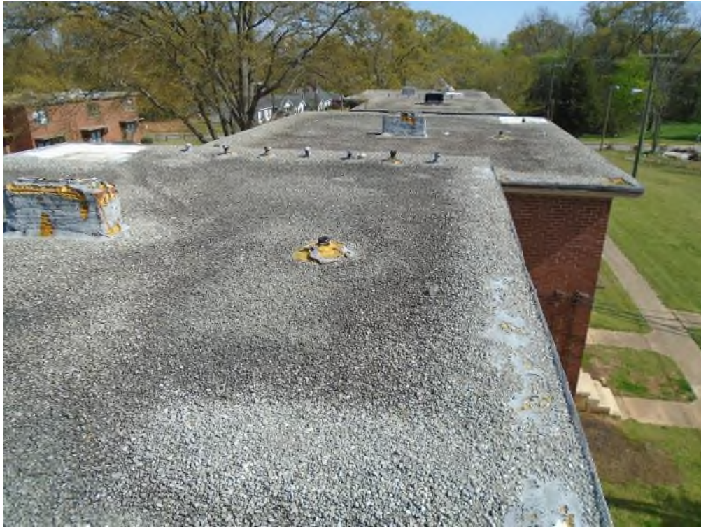
Photograph 43 - BLDG 13 – Overview looking east
