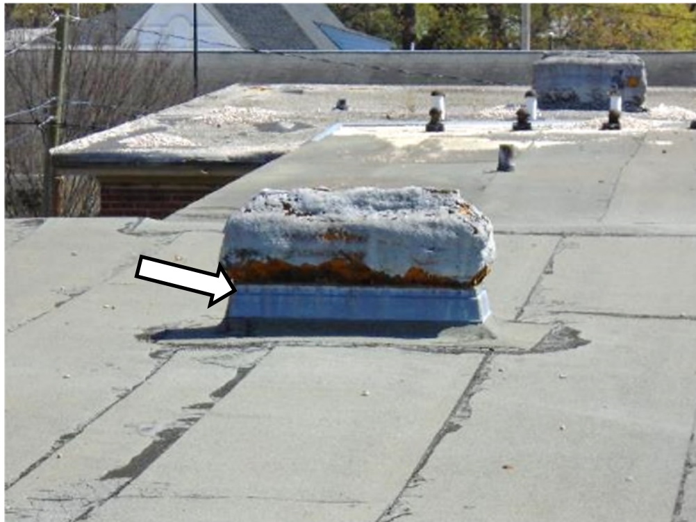
Photograph 14 - BLDG 3 – Counter flashing in fair condition
