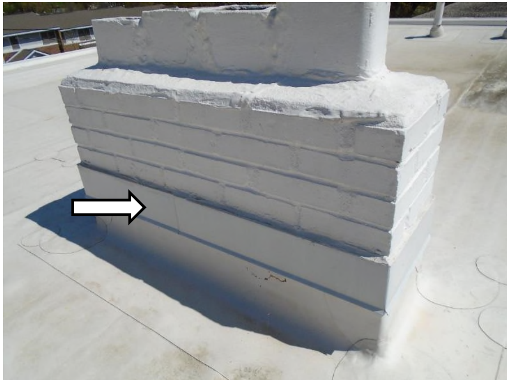
Photograph 10 - BLDG 2 - Chimney flashing and coating on TPO roof
