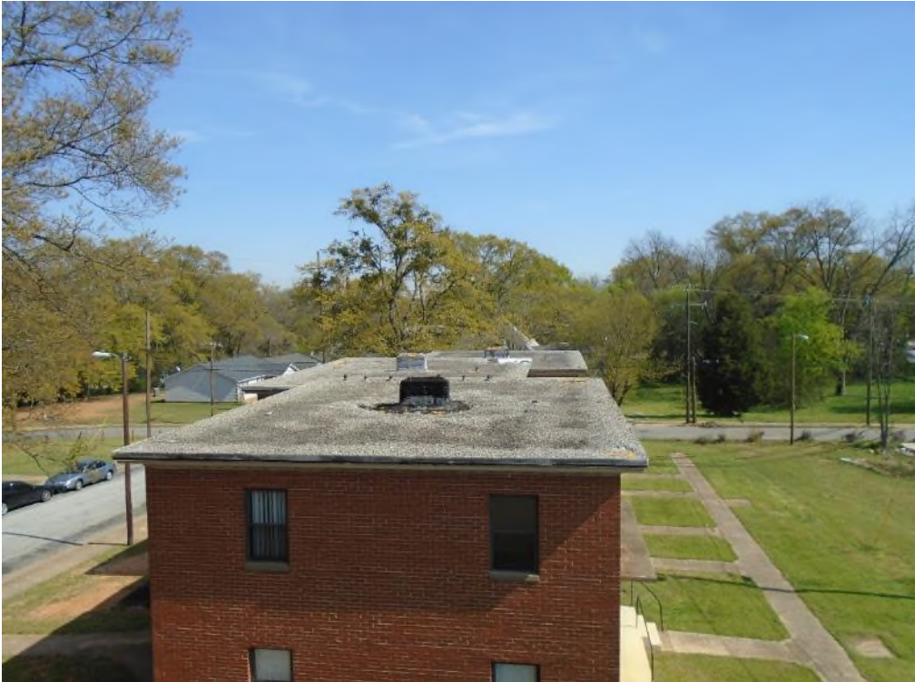
Photograph 41 - BLDG 12 – Overview looking east
