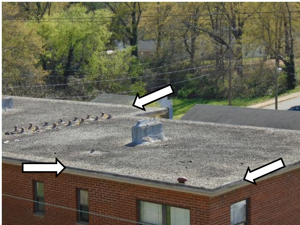
Photograph 24 - BLDG 6 – Wire mesh used as gravel stop
