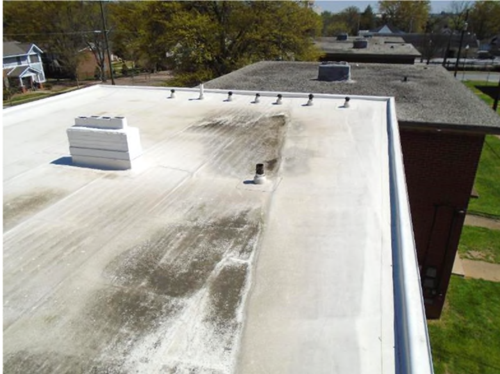
Photograph 9 - BLDG 2 - TPO roof overview
