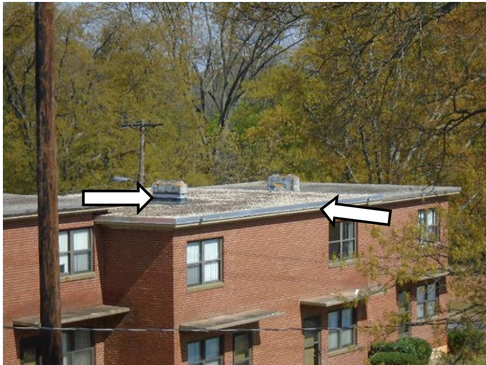
Photograph 36 - BLDG 10 - Metal flashing upgraded after roof installation
