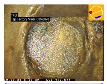
Distance: 472.5 ft. Grade: Condition: Tap Factory Made Defective
