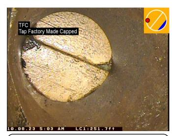
Distance: 251.6 ft. Condition: Tap Factory Made Capped Remarks: CAPPED WITH BRICK
