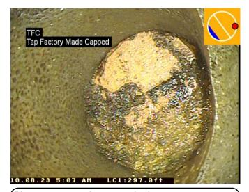
Distance:297.0 ft.Grade:0Condition:Tap Factory Made CappedRemarks:CAPPED WITH BRICK
