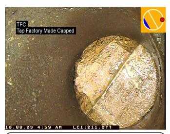
Distance: 211.1 ft. Condition: Tap Factory Made Capped Remarks: CAPPED WITH BRICK
