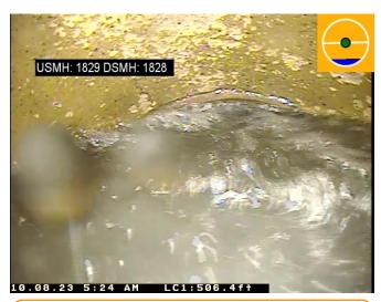
Distance:505.2 ft.Grade:4Condition:Joint Offset Large Defective
