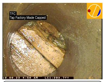
Distance: 203.6 ft. Grade: Condition: Tap Factory Made Capped Remarks: **CAPPED WITH BRICK**
