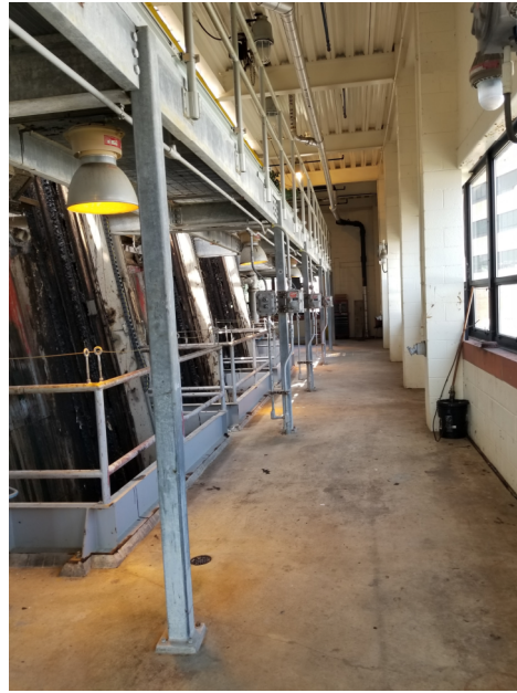
PTB Upgrades, (WPB2) Phase 9B
