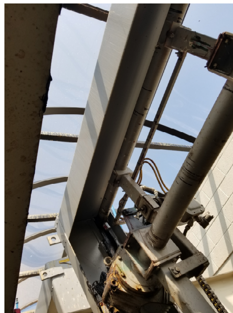
PTB Upgrades, (WPB2) Phase 9B
