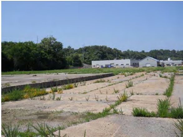
Photo #13 View of the building pad and the Chattanooga Bakery property located adjacent to the north.
