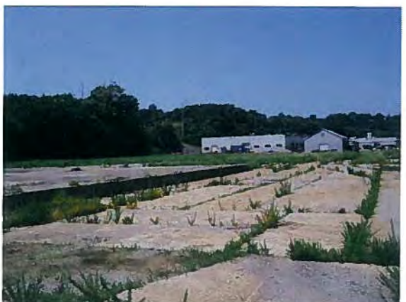
Photo #12 View of the building pad located at 155 Hamm Road.
