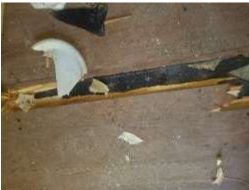
HOMOGENEOUS AREA 06 FLOOR FELT PAPER
