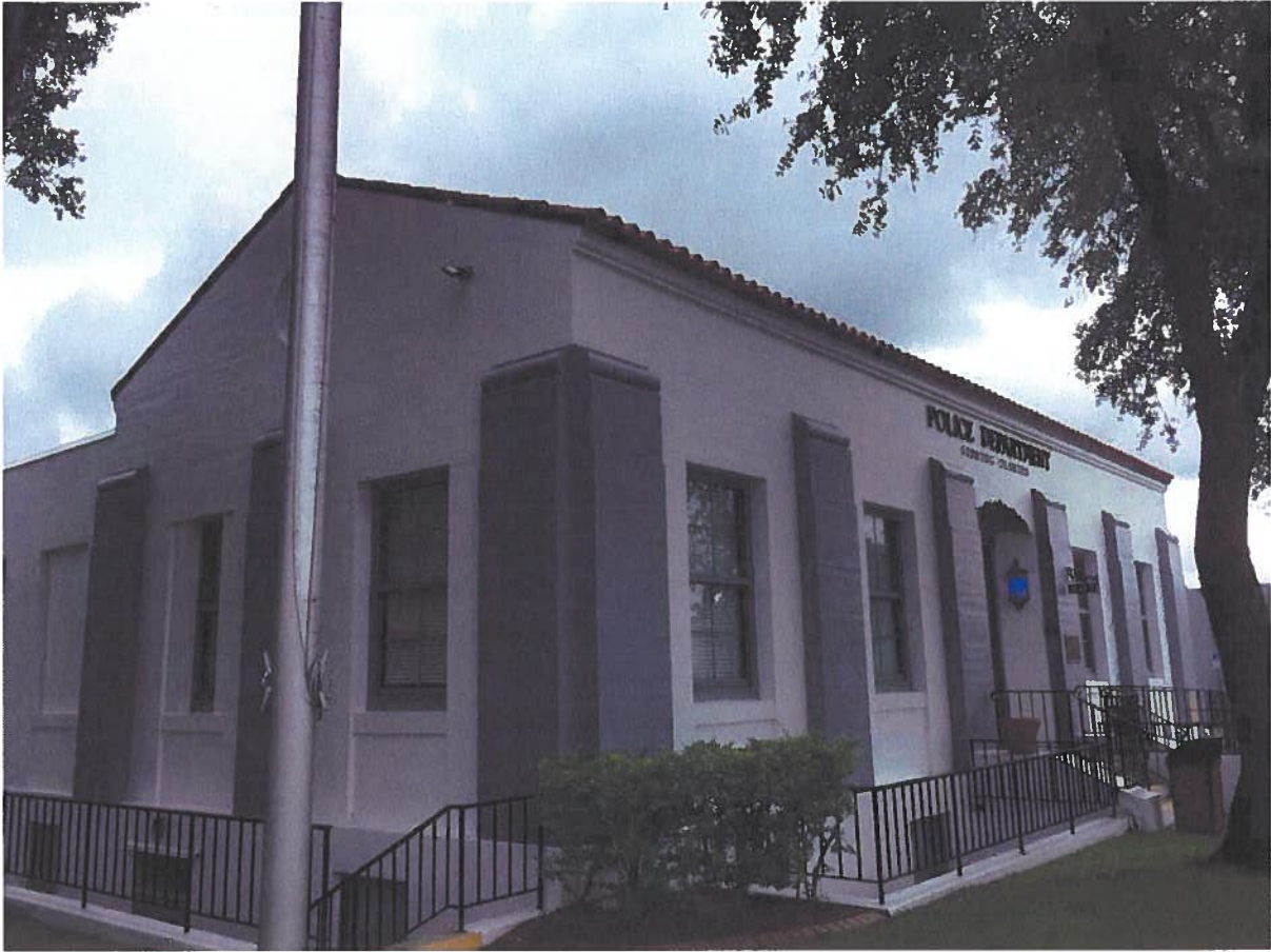
Photo 2: Police Station Roof (South/East Elevation)
