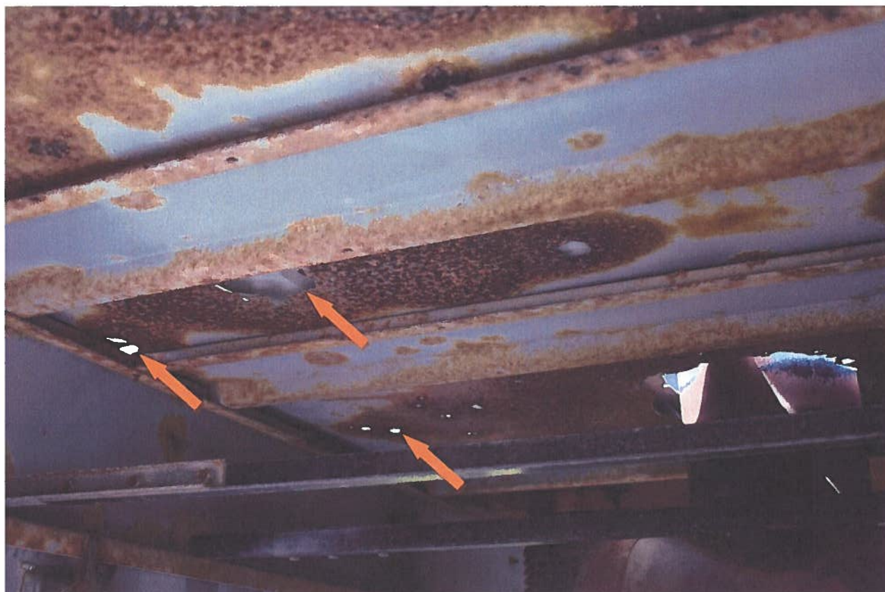
Photo 3 (corrugated metal on roof of steel enclosure )
