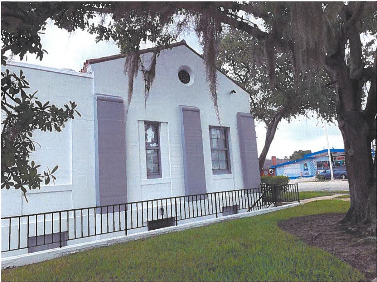
Photo 1: Police Station Roof (South Elevation)
