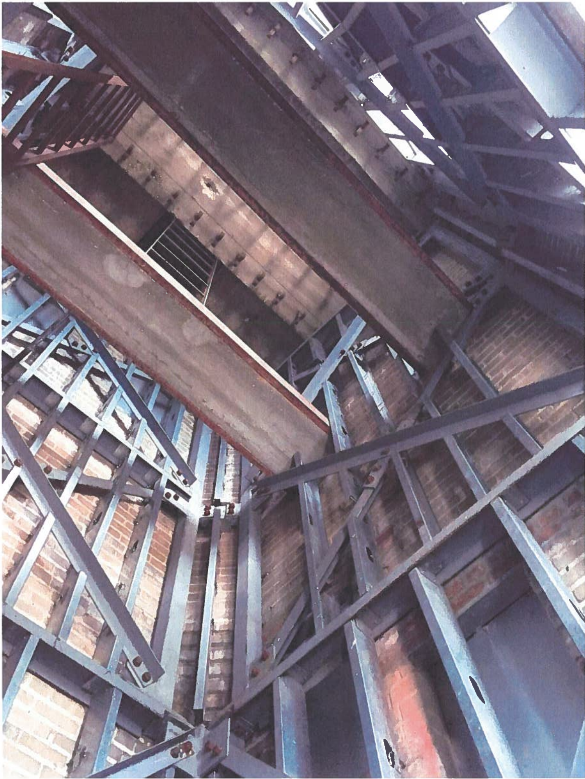
Photo 9: Hose Tower Supplemental Steel
