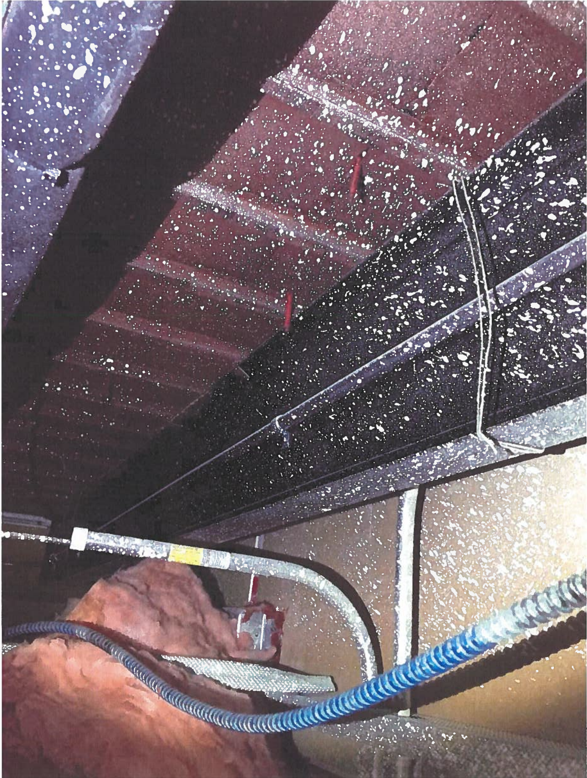
Photo 4: Metal Roof Deck
