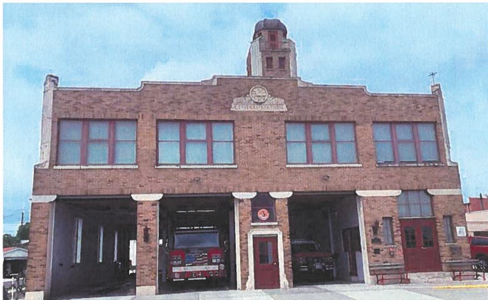
View of the front elevation of the Fire Station #14
