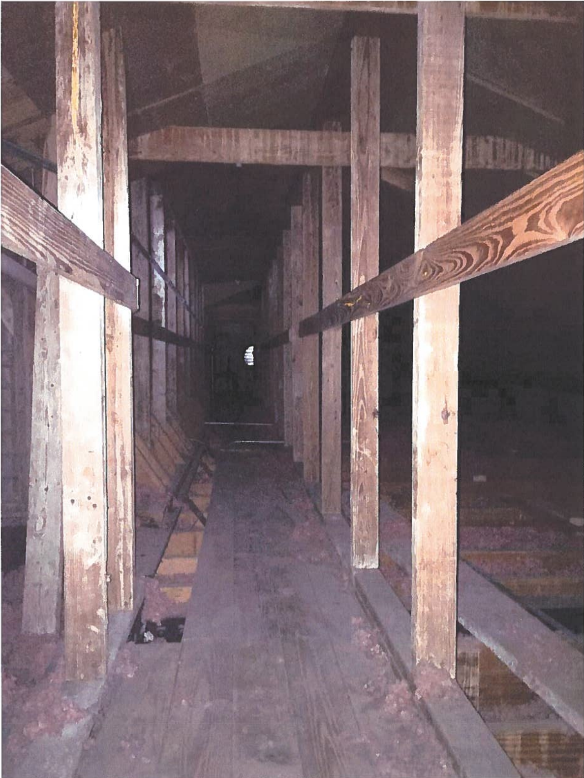
Photo 4: Gable Roof Ridge Beam Support
