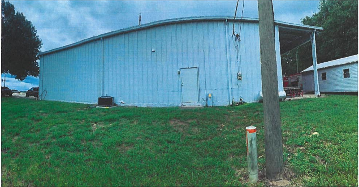
Photo 3: FS#15 West Elevation
