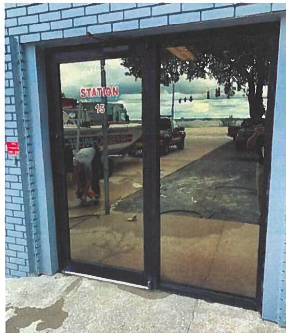
View of non-impact rated entry door and storefront window
