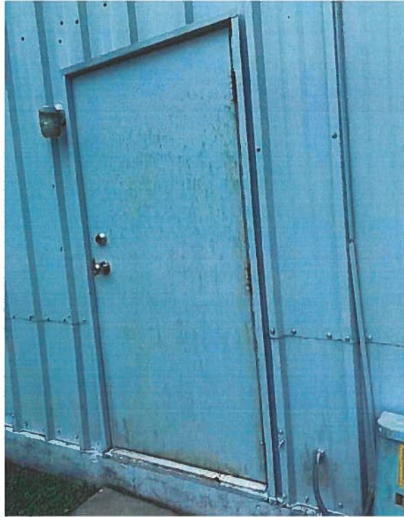
View of existing steel man door
