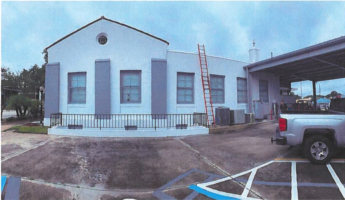
Photo 3: Police Station Roof (North Elevation)
