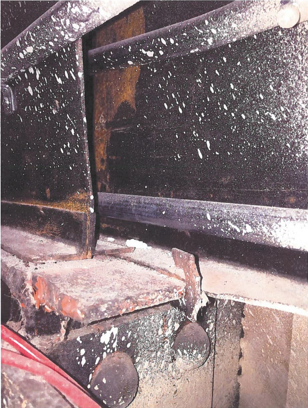
Photo 6: Steel Roof Joist
