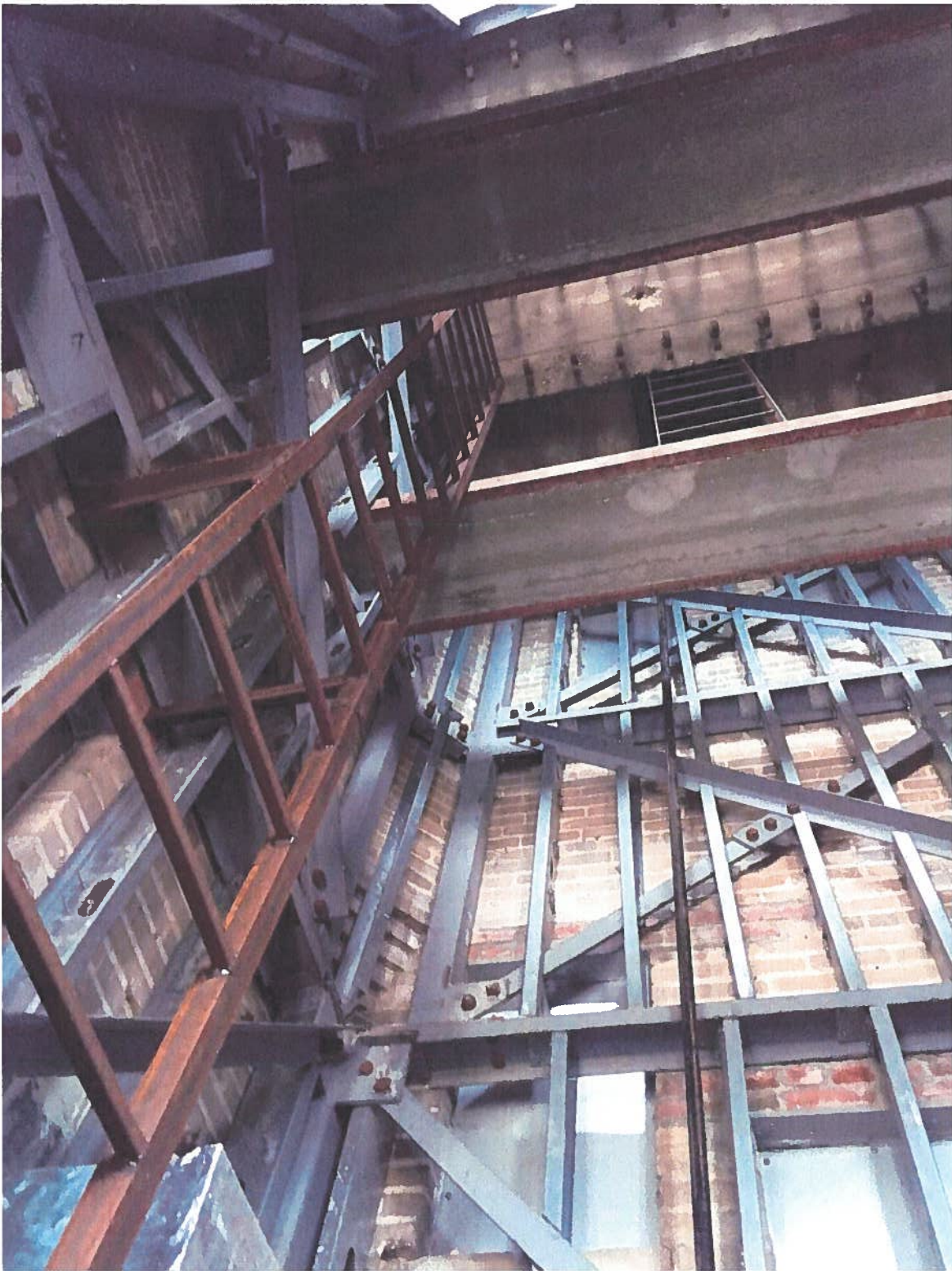
Photo 8: Hose Tower Supplemental Steel
