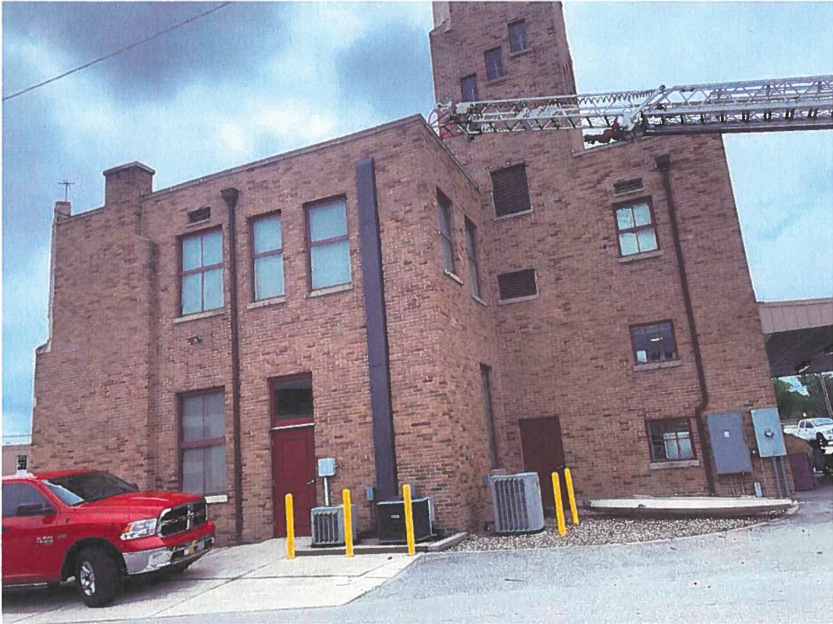
Photo 2: Fire Station #14 Elevation
