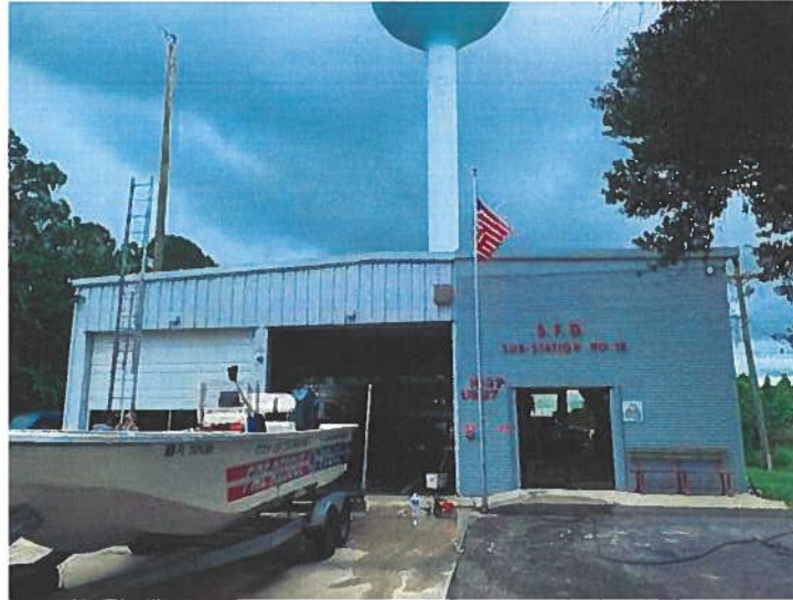
View of the front elevation of Fire Station #15
