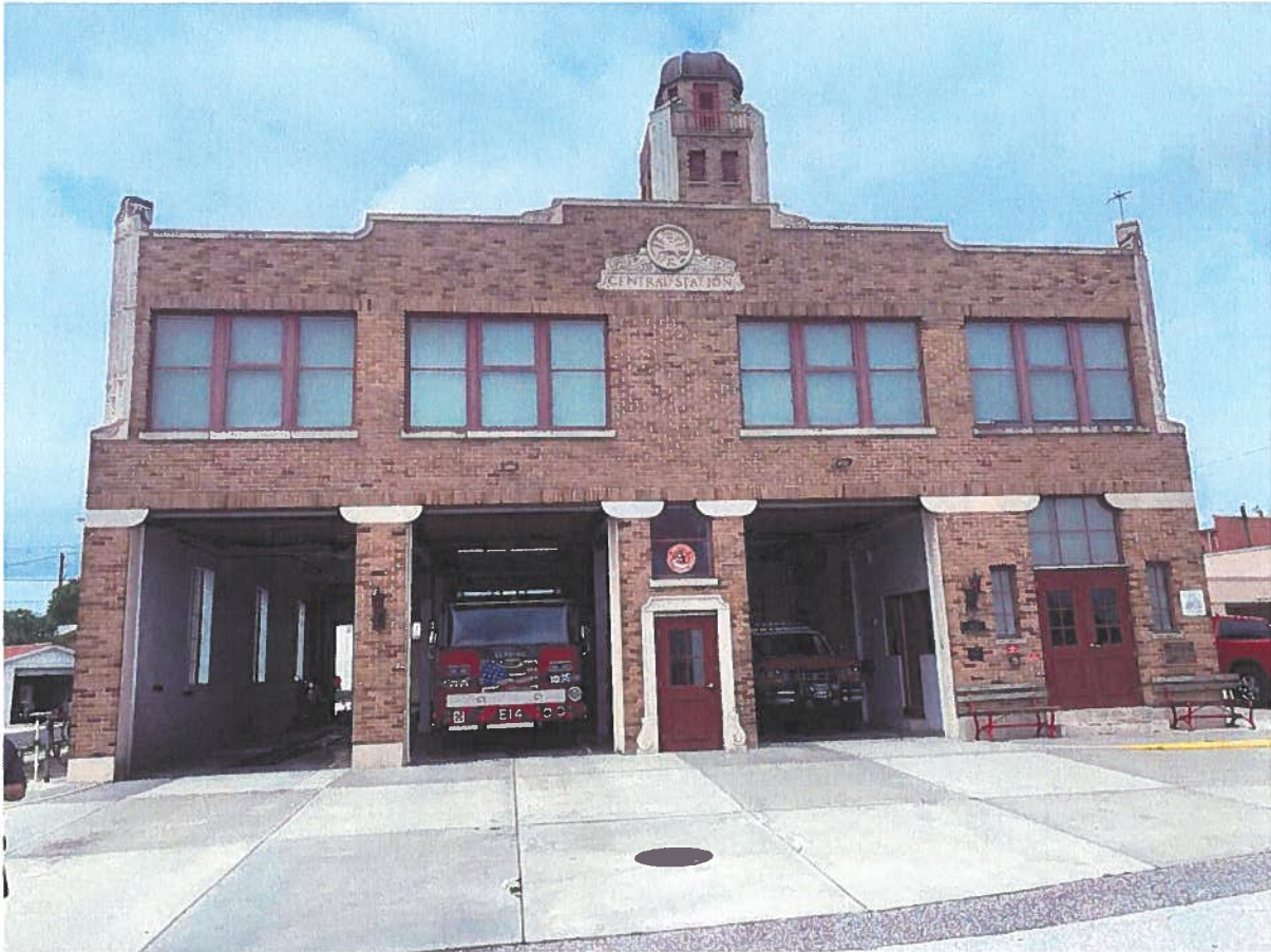
Photo 1: Fire Station #14 Elevation
