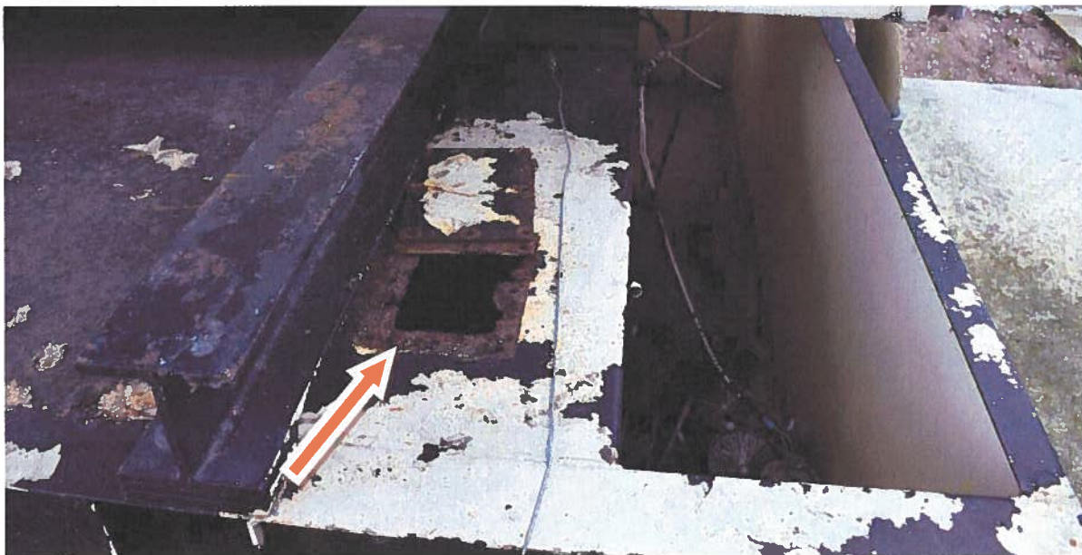
Photo 12 – top of tank inspection port of tank liner
