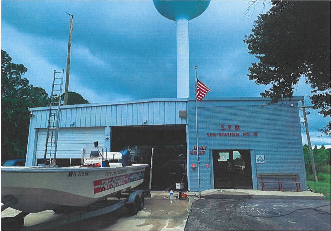
Photo 1: FS#15 North Elevation
