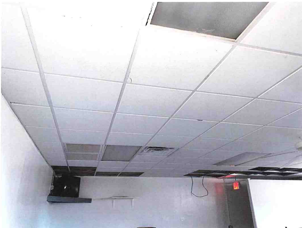
2' x 2' Ceiling Tile, Throughout Building
