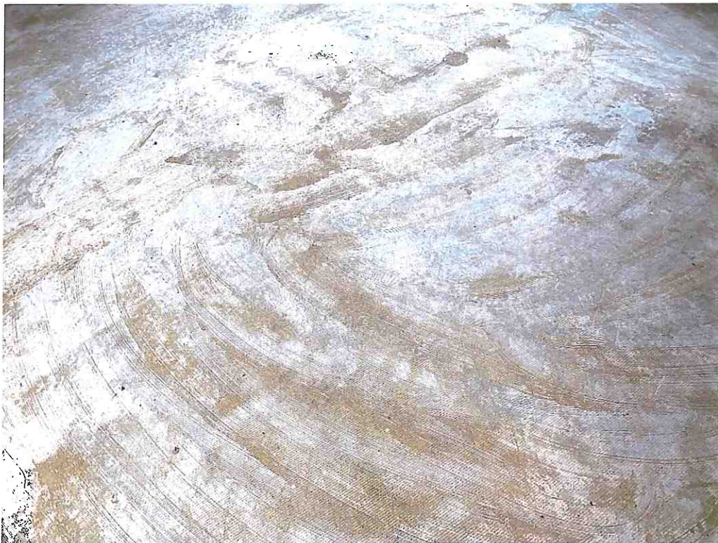
Floor Mastic (Yellow), North Section of Building
