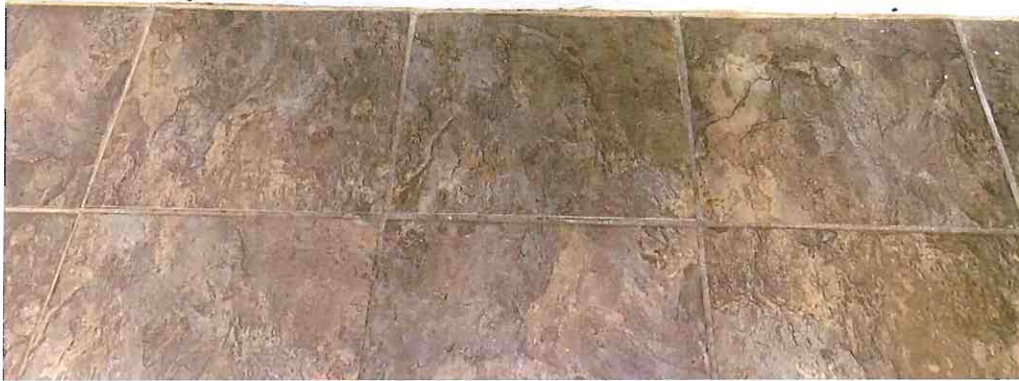
Baseboard and Marble Curb at Shower, South Section of Building
