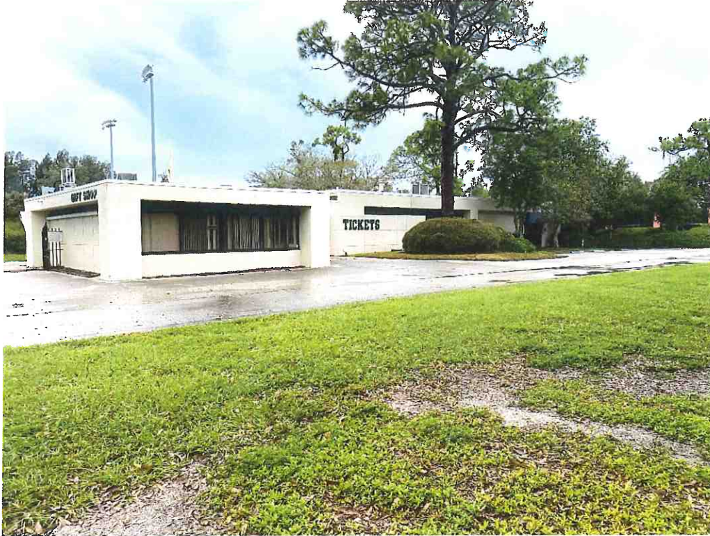
Looking Northwest at Building
