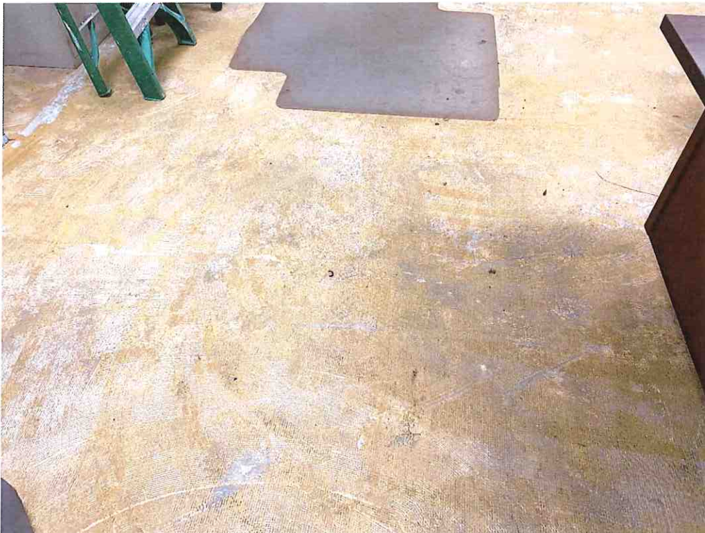
Floor Mastic (Yellow), South Section of Building
