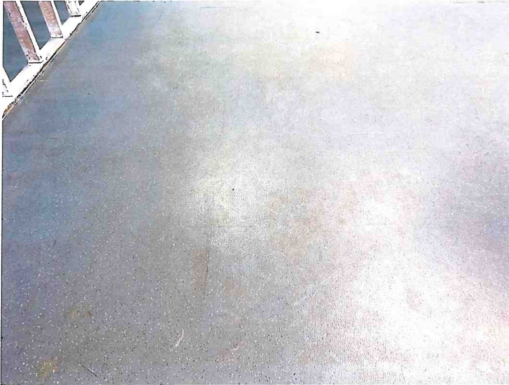
Rubber Flooring (Green), South Section of Building
