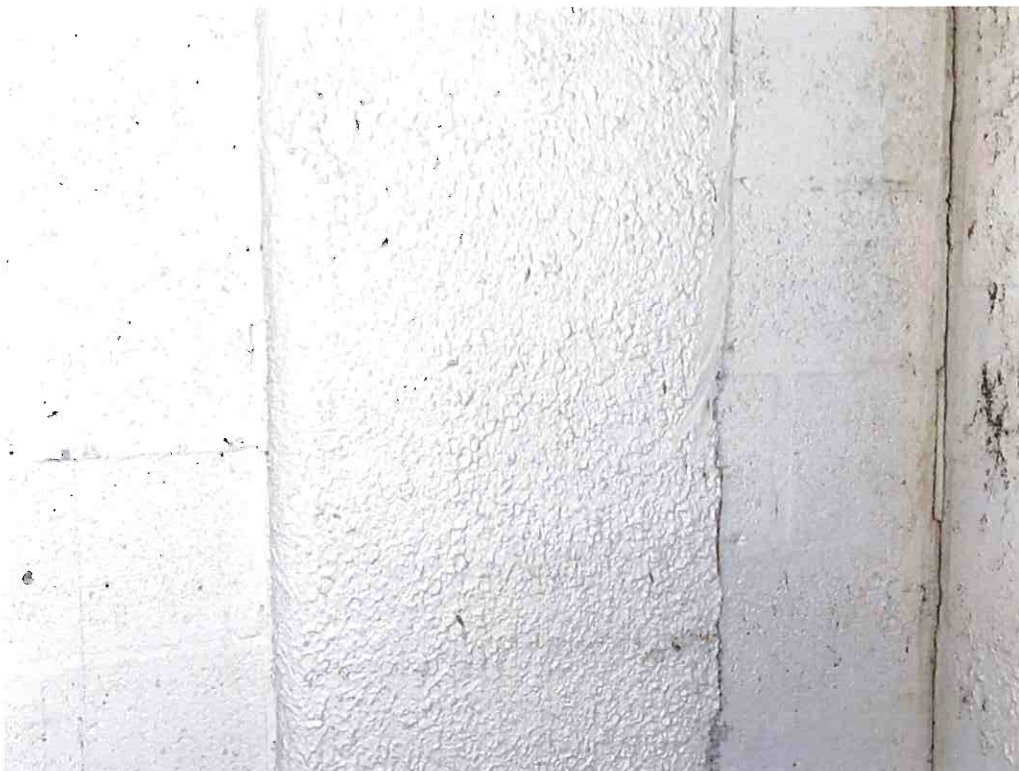
Plaster Skim Coat on Concrete Block, North Section of Building
