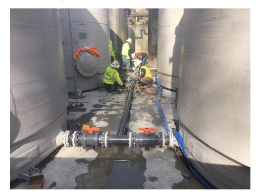
**Item #4:** The current containment area for the existing tanks contains rainwater. It is the Contractor's responsibility, as part of this work, to pump out the contents of the containment area and clean the containment area prior to the placement of new construction materials within the existing containment area. Content of the containment area is stormwater, which will be discharged (in a non-erosive manner) to the existing drainage channel located south of the current tank containment area.
